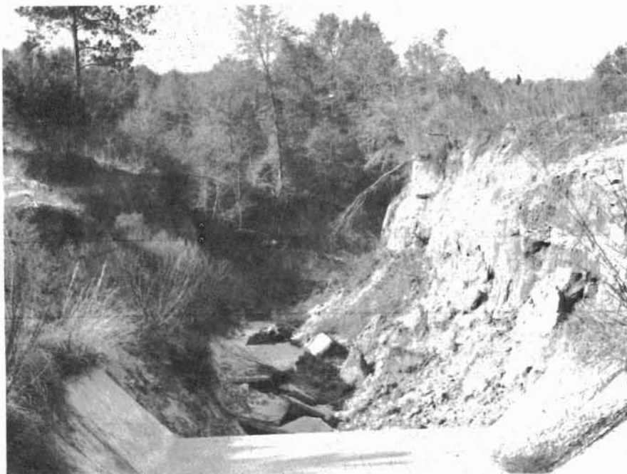
Stream pollution is often caused by the structural failure of the storm drain and outlet energy dissipator. When this happens, as pictured here, the unstable downstream channel is scoured.
