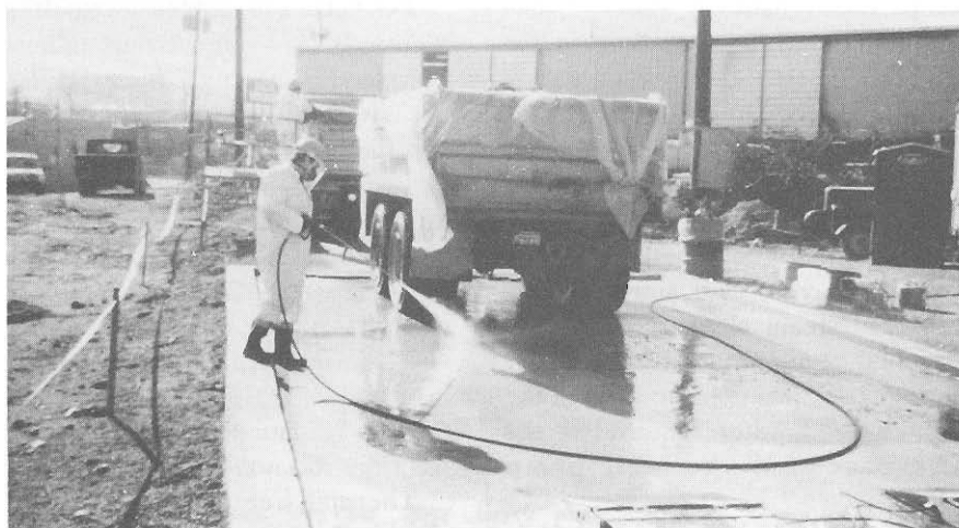
1705 decon site showing decontamination in progress.
