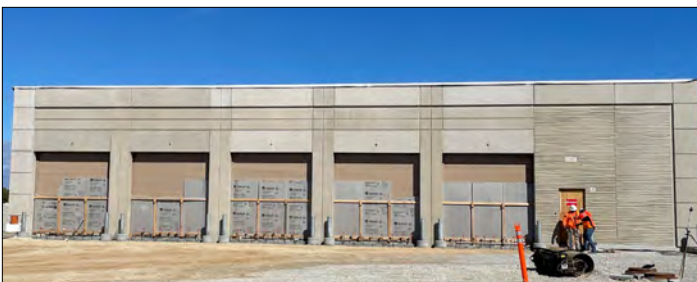
A view of the five-bay ambulance garage.
