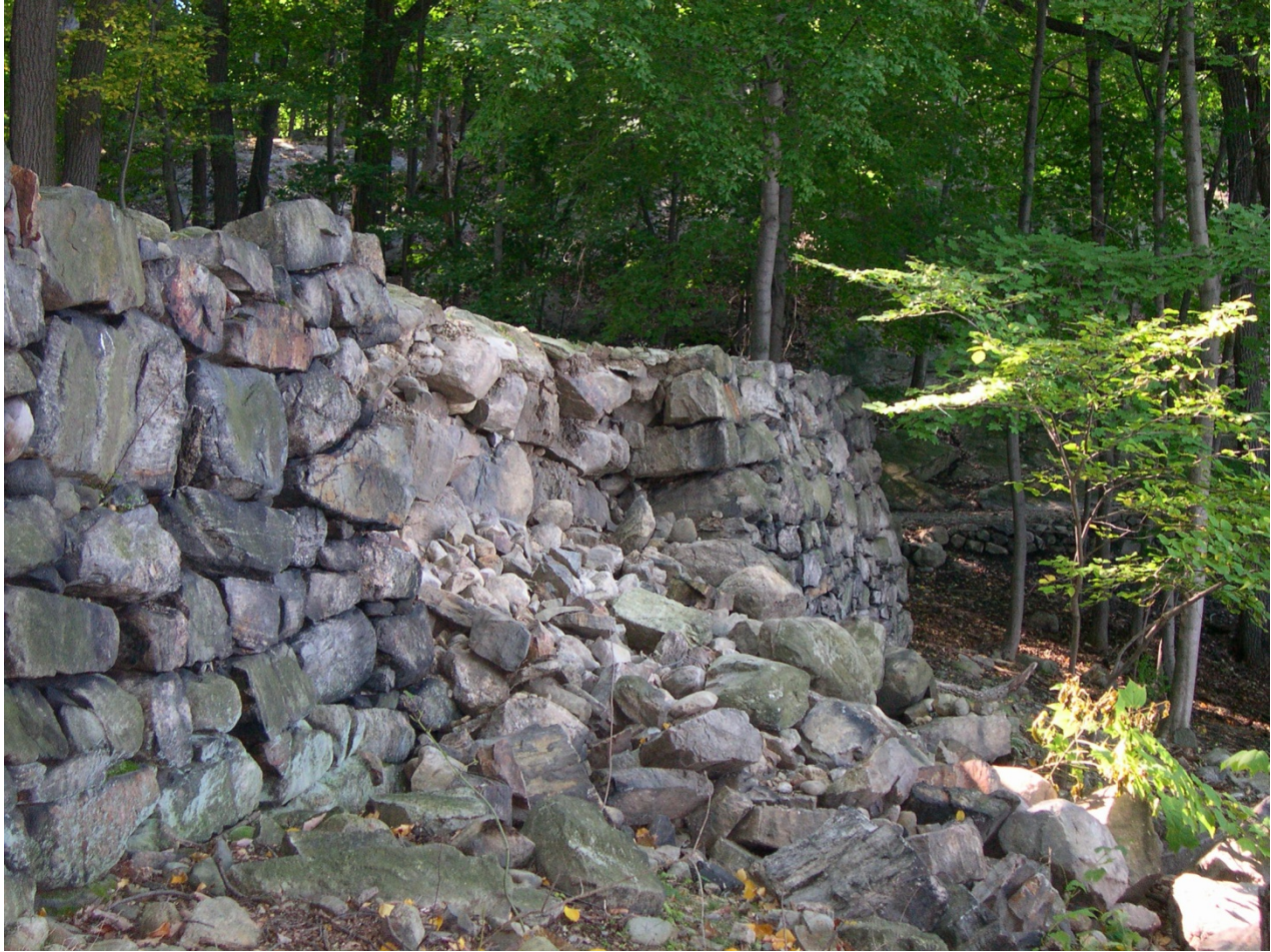
The 1778 Chain Battery collapsed as a result of Tropical Storm Jeanne on September 27-28, 2004; and has yet to be repaired by West Point. This Battery is regularly used by the Department of History and DMI for American history and military instruction. In addition to the Chain Battery being an irreplaceable part of West Point and Revolutionary War history, its damage seriously degrades the educational and military training experience of the Corps of Cadets.
