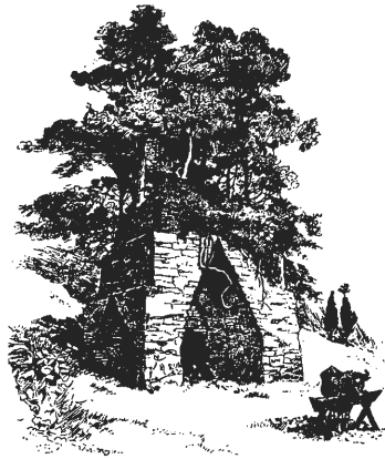
Figure 1: View of the former Queensboro Ironworks furnace stack, as it appeared in 1884. Source: Ransom, 1966: 161
