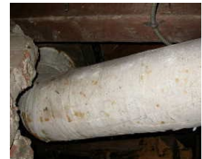
Paper Pipe Insulation
