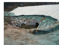
Silt Fence and soil stabilization
