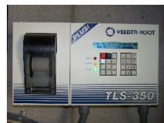
Electronic Leak Detection Systems
