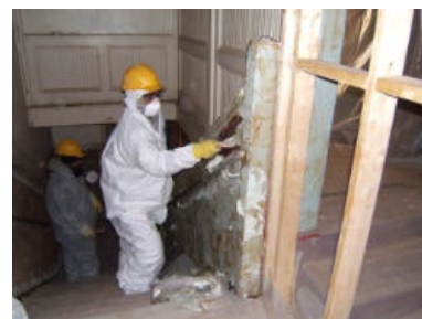
Lead Paint Removal
