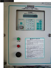
Electronic Leak Detection Systems
