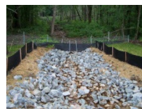
Silt Fence, rip rap, and hay stabilization
