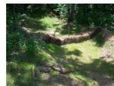
Hay bales and vegetative stabilization
