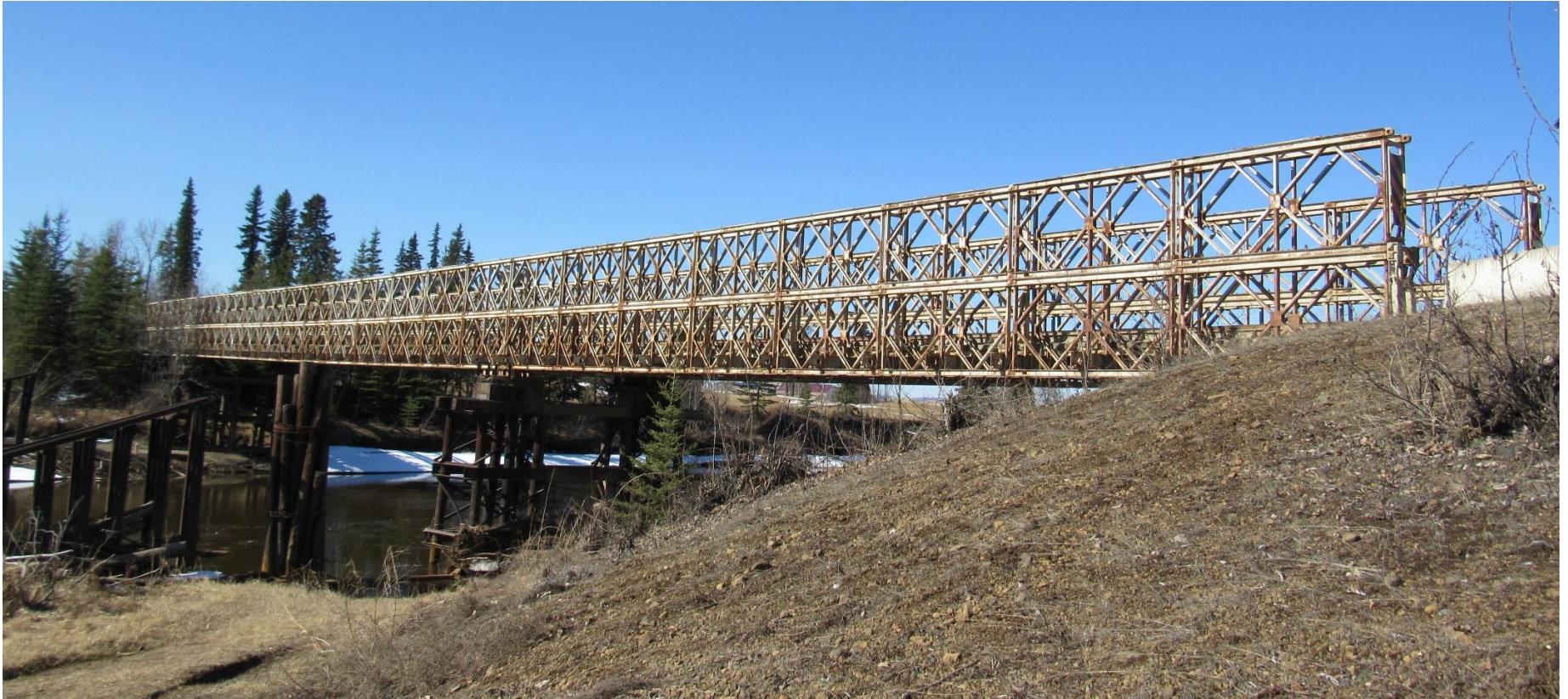
Figure 3. Photograph of Existing Bailey Bridge (2019)
