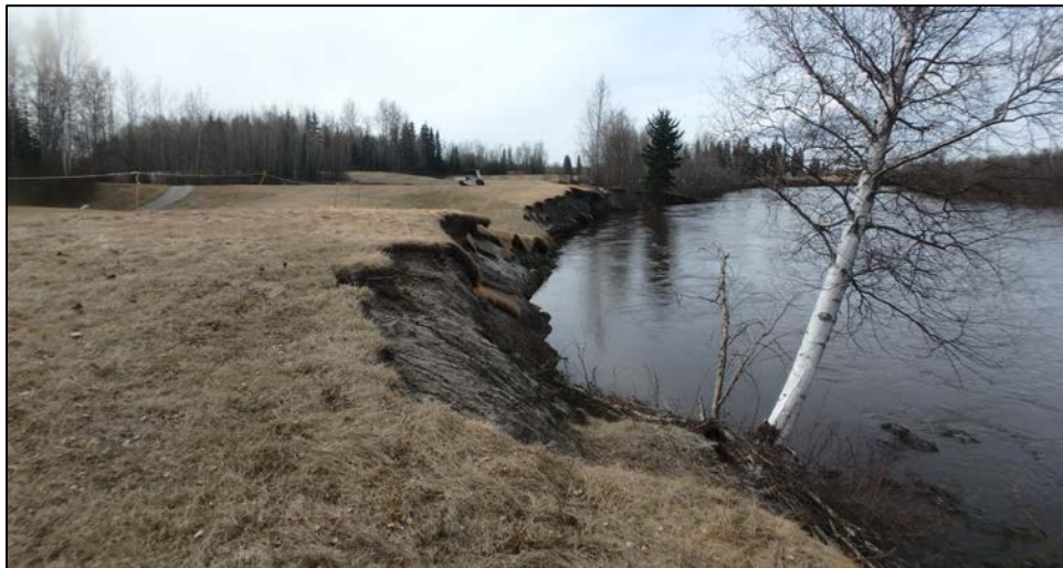
Figure 3. Bank stabilization project area.
