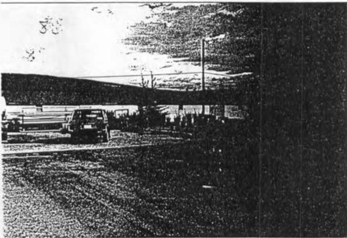
Photo #38 S-10 Waste Accumulation Point, Bldg. 112B, note unbermed tank on left
