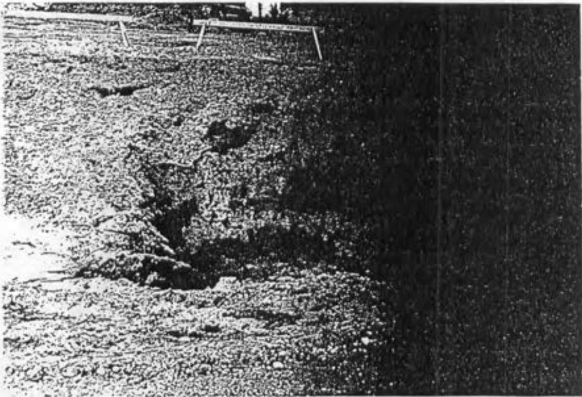
Photo #48 S-6 The UST trench reveals visibly contaminated soil
