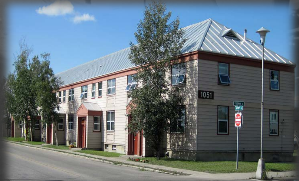
Building 1051 (FAI-00456) contains a hip and gable roof, a characteristic of the World War II era buildings on Post.
