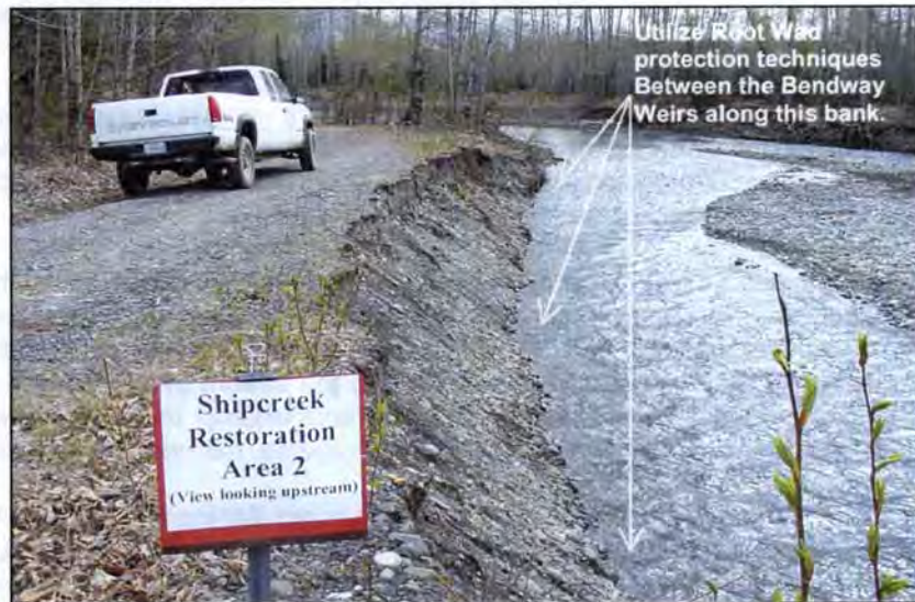
Figure 20. Area 2 example of proposed stabilization measures along Ship Creek banks.
