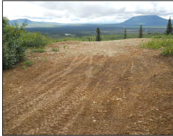
Figure 127. XMH-00277/00879, Point 1, 6/29/11 (SSW)
