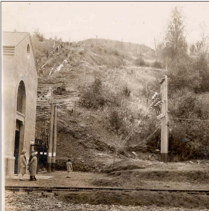
Figure 15. Penstock construction in background behind powerhouse. Note railroad spur in foreground, which was removed after construction was completed.
