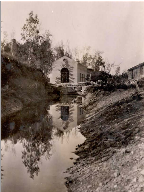
Figure 19. Tailrace extending from rear of powerhouse.
