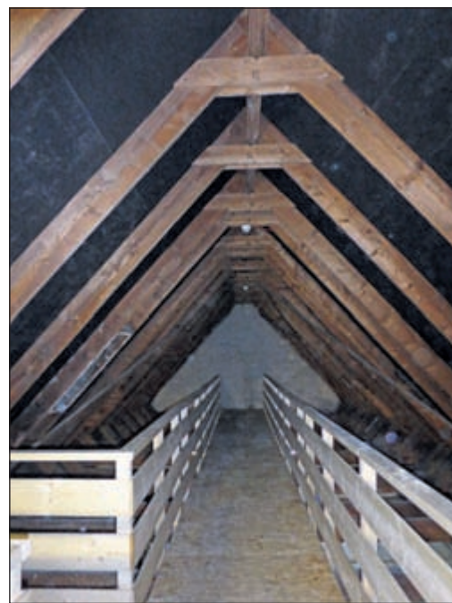
A wooden walkway inside the attic of Bldg. 154 nears completion for installation and maintenance of electrical parts of the solar panel system.
