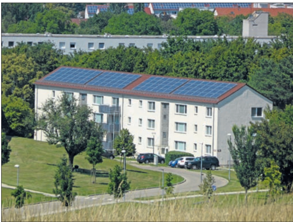
The solar systems on Robinson Barracks' buildings 301 and 302 are oriented toward the south for ideal solar collection.
