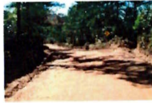
Turn-out at gradient changes.
