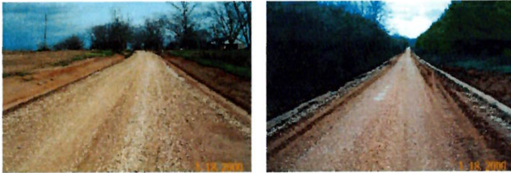
Exhibit 1.1a - Examples of 3/4" to 1' crown with road ditches in place. Water sheds readily off the crowned road surface and into the ditches. Proper drainage off the roadway surface helps to maintain a good "crust" which stabilizes the roadway and helps provide a good riding surface.
