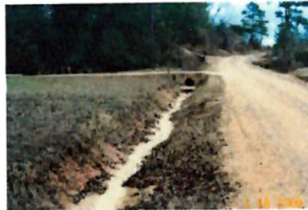
Rounded V-Shaped Ditch
