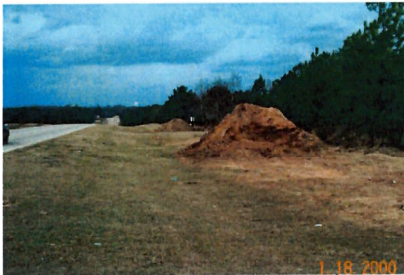
Soil stockpiles located on a well vegetated hillcrest and away from concentrated flow channels
