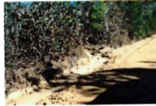
Turn-outs into filtering areas.
