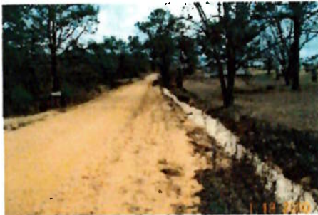
Flat Bottom (Trapezoidal) Shaped Ditch
