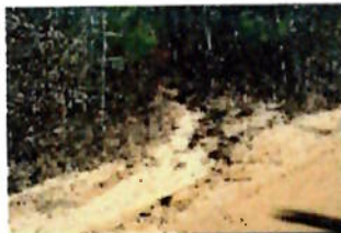
Turn-out to a drop inlet.
