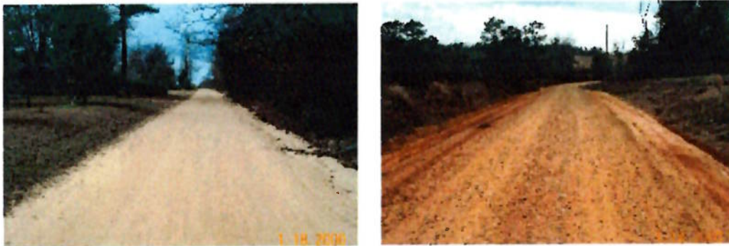
Exhibit 1.1b - Examples of 0" to 1/4" crown with no road ditches in place. Water infiltrates the soil of the sandy and flat road surface minimizing runoff from the roadway. The water that sheds from the roadway is readily removed from the road surface into the roadway edges allowing a passable lane in the center of the roadway.
