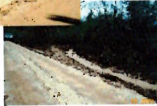
Turn-outs into filtering areas.
