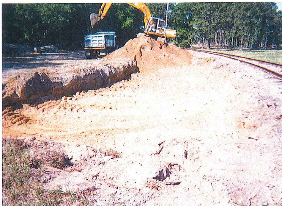
SWMU 31: Removal of contaminated soil at SWMU 31.
