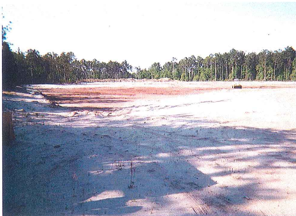
SWMU 31: Borrow pit used for backfill material at SWMU 31.
