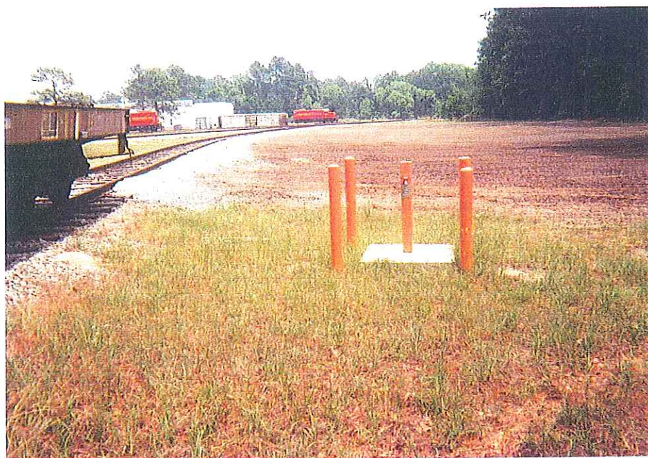
SWMU 31: SWMU 31 area after backfilling.
