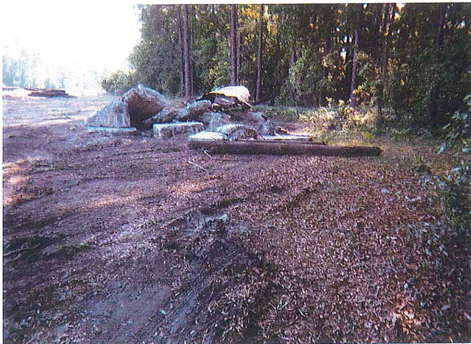
SWMU 31: Concrete from tank supports and power pole at SWMU 31 stockpiled for disposal.
