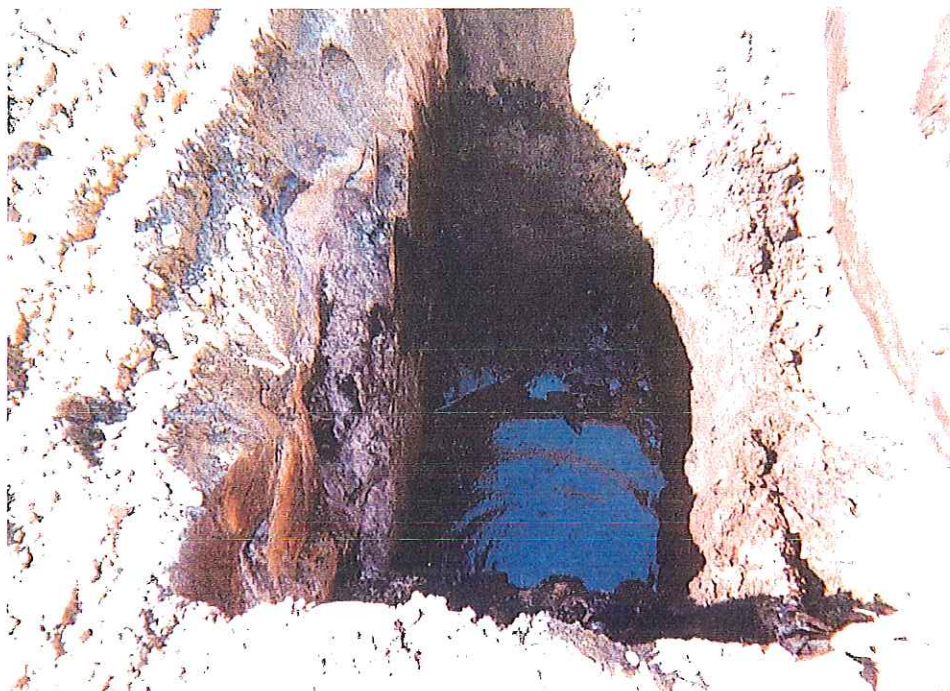
SWMU 31: Groundwater which was encountered during the excavation of SWMU 31.
