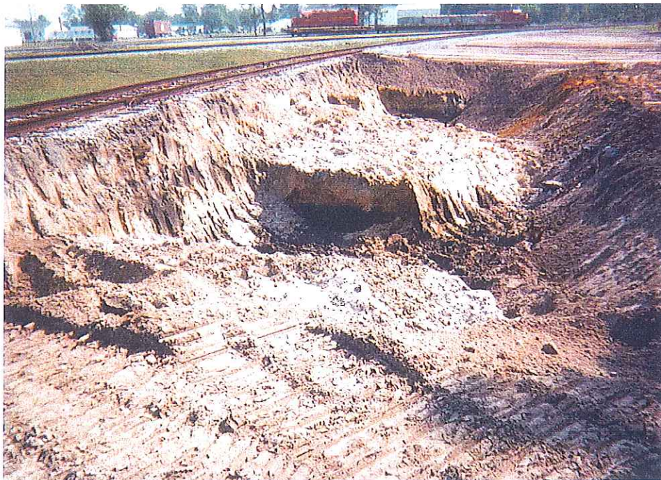
SWMU 31: Part of excavation area at SWMU 31.
