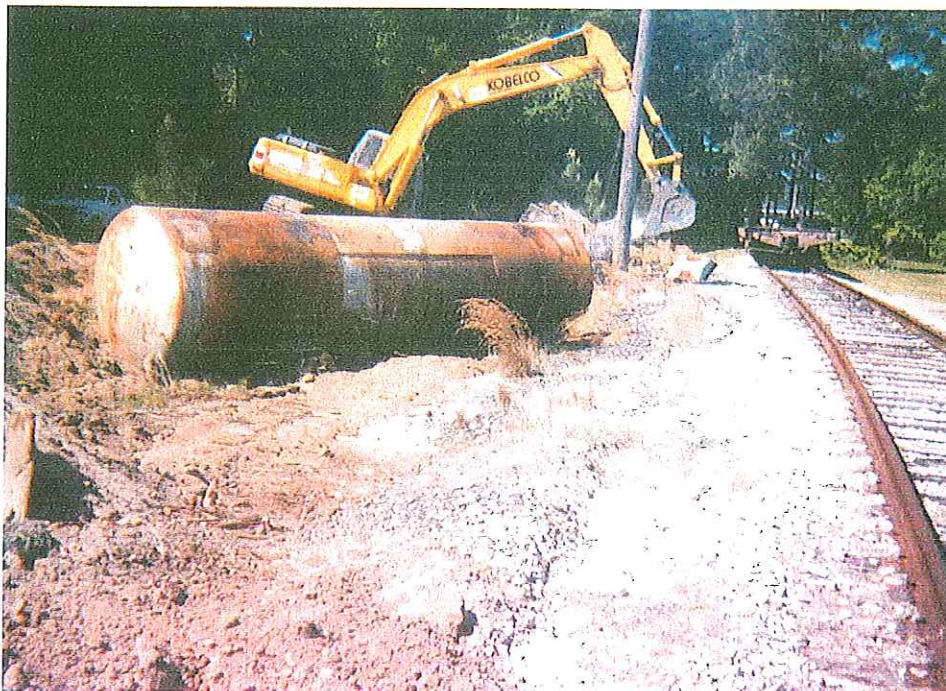
SWMU 31: Removal of 1500-gallon AST at SWMU 31.
