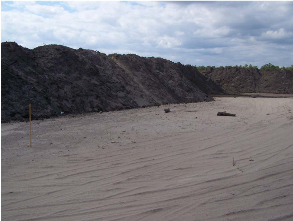
Inspected clean soil moved at the west side of the South Pond site
