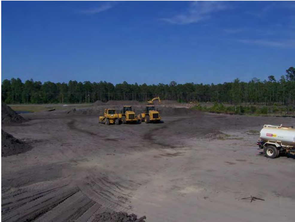
Current progress on the west side of the South Pond site
