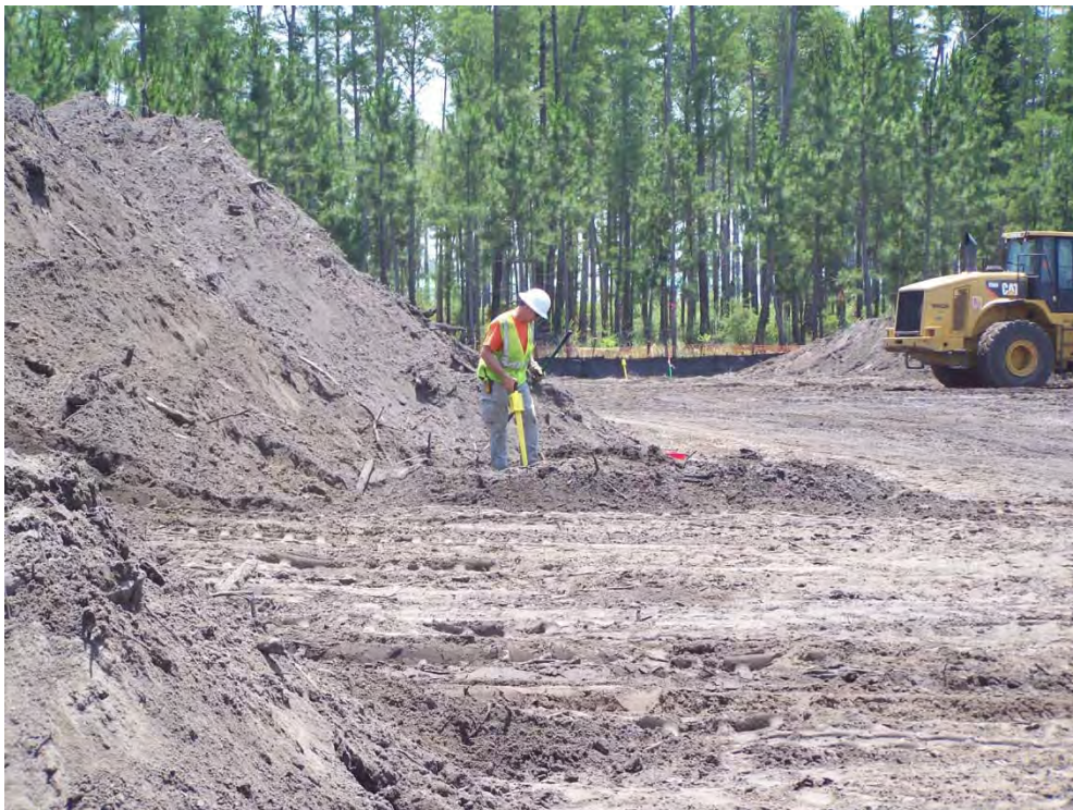
QC inspection at the South Pond site
