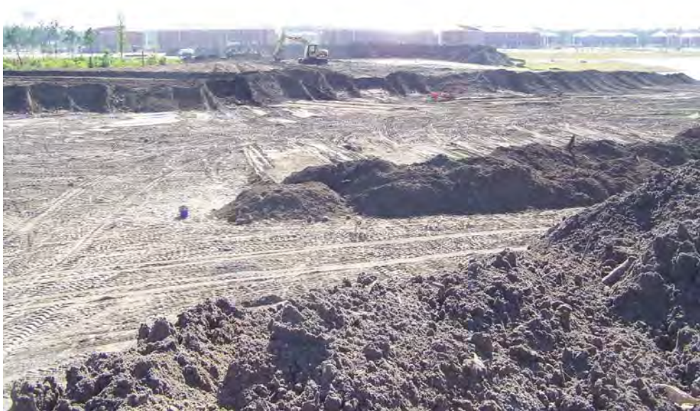
Current progress on the east side of the South Pond site
