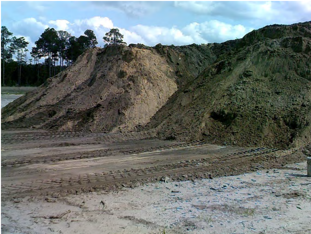
Inspected soil pile at South Pond site. (1130 cys)
