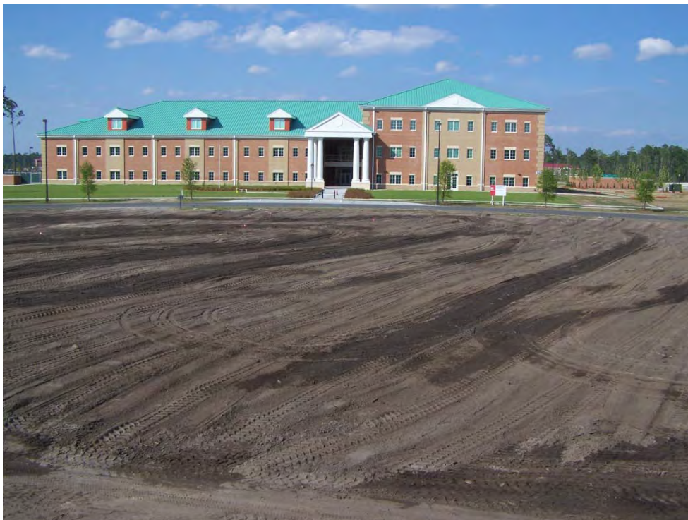
Current progress at the HHQ site
