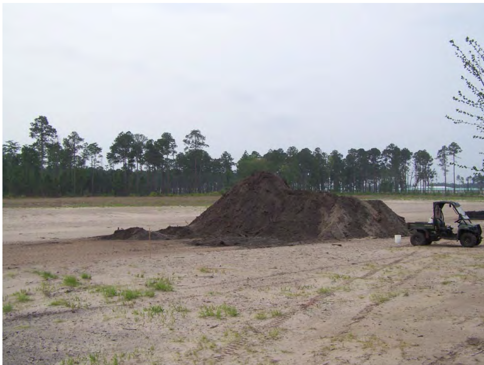
The 405 cys of dirt moved at the South Ponds site
