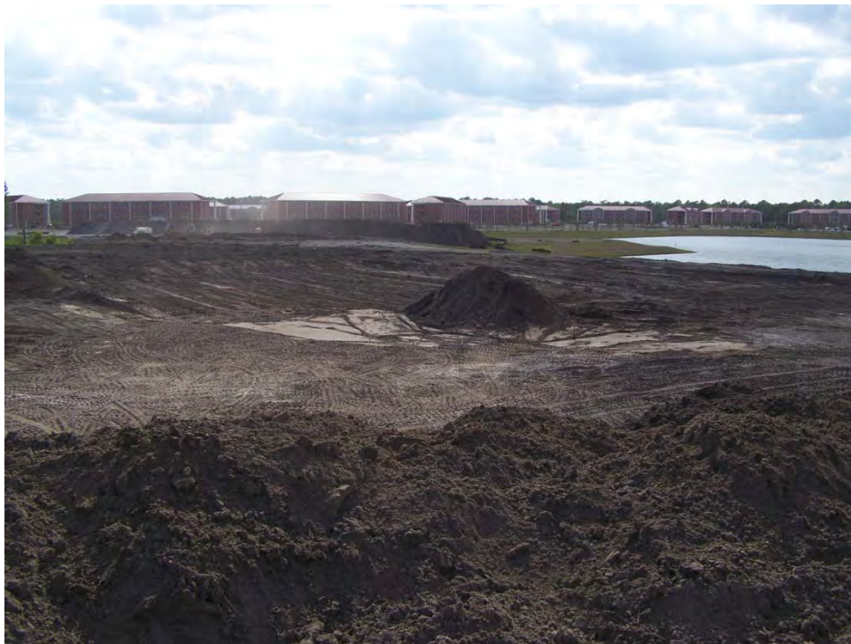
Current progress at the east side of the South Pond site
