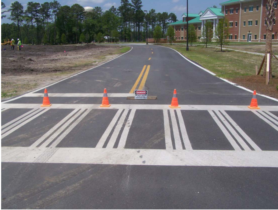
Road to the HHQ building that has been closed off
