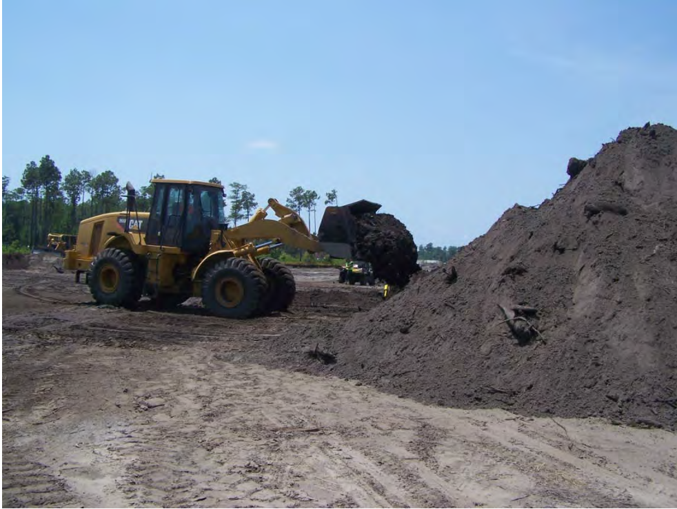
Working soil pile at the South Pond site
