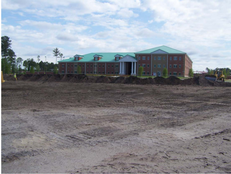
Current progress at the HHQ site
