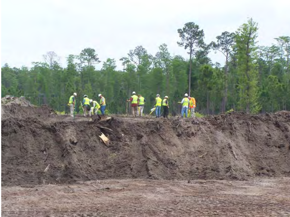
Inspection of the upper shelf at the South Pond site
