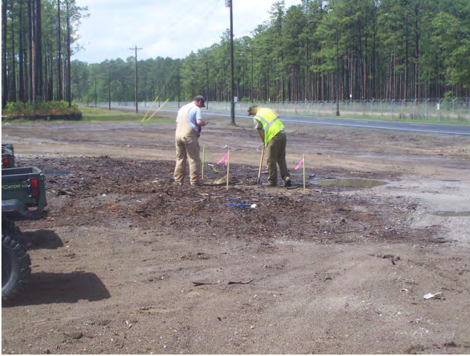
Installation of new schonstedt test grid.
