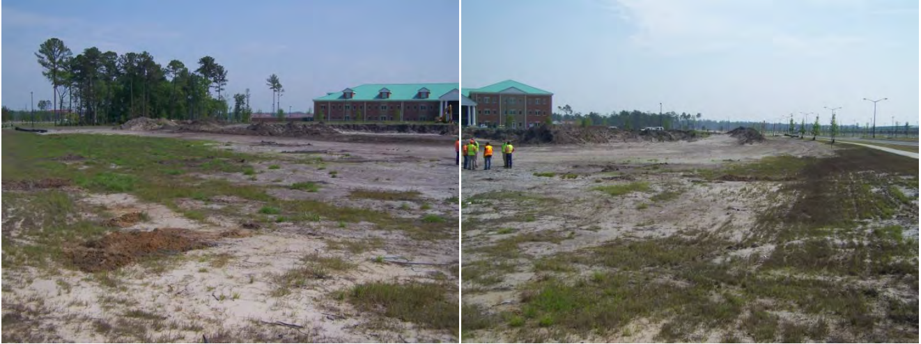
HHQ Site initial visit.
