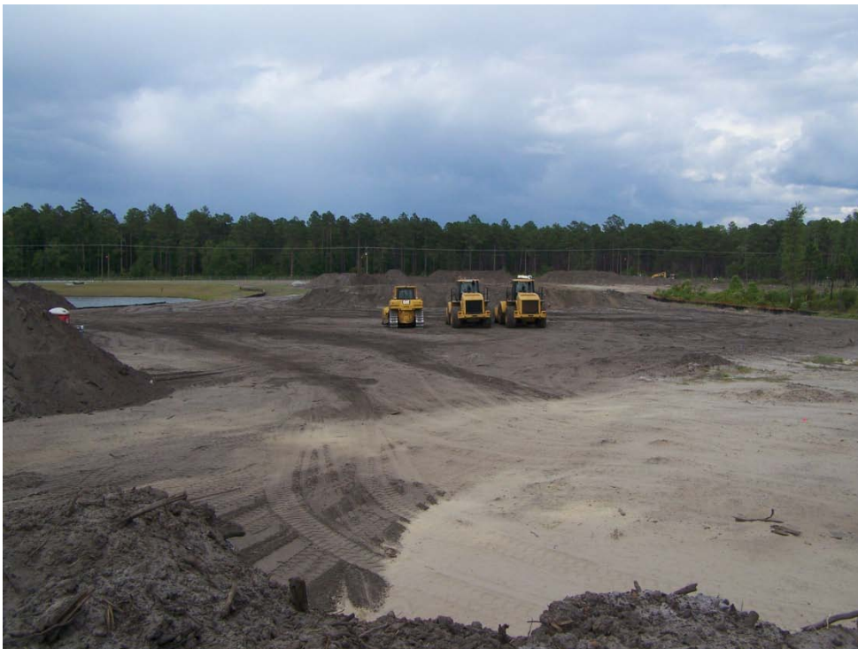
Current progress at the west side of the South Pond site
