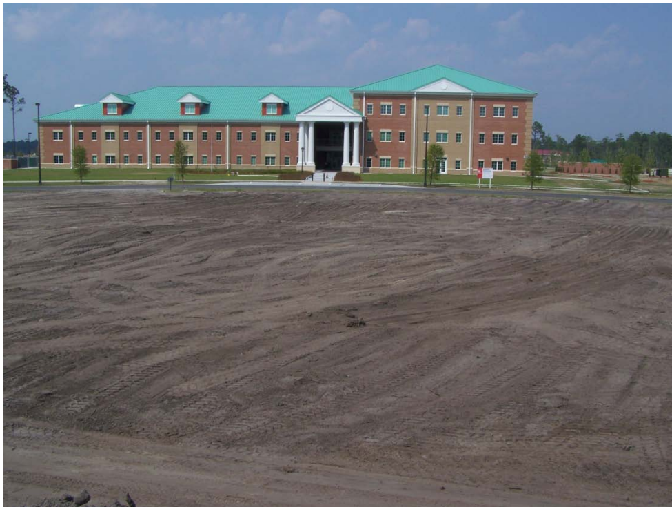
HHQ site at its current state
