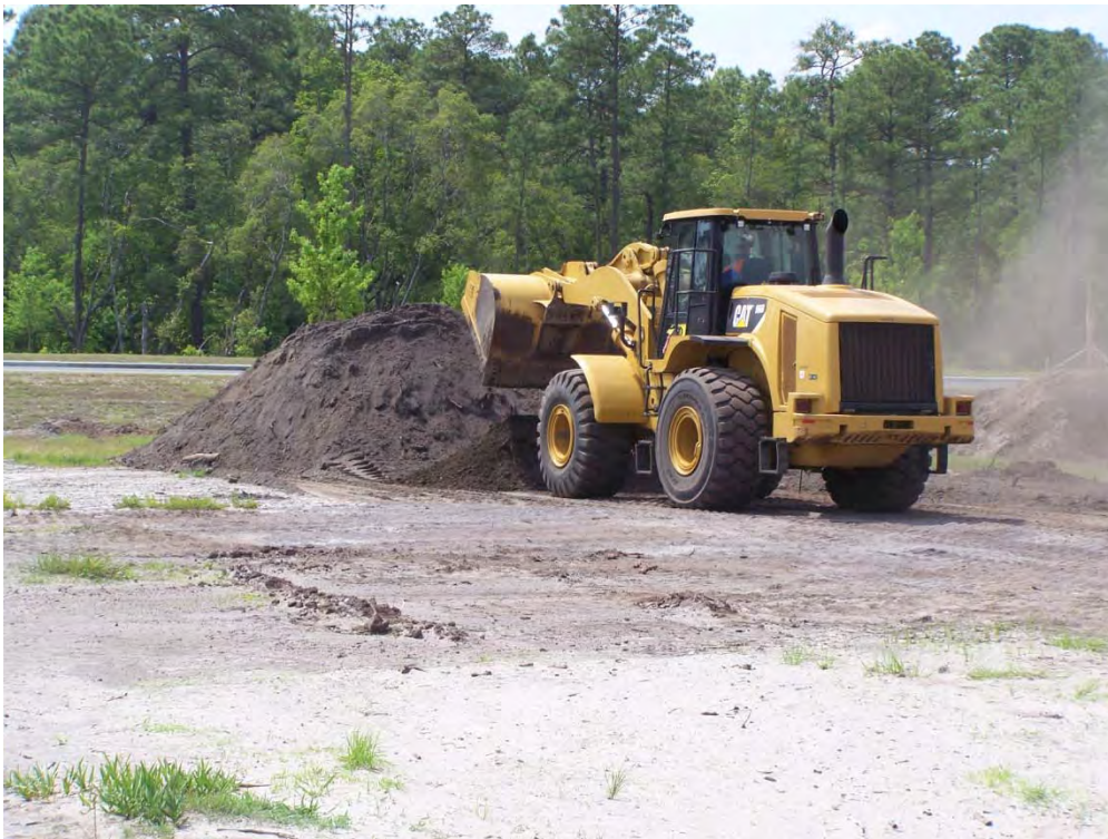
Working HHQ soil pile
