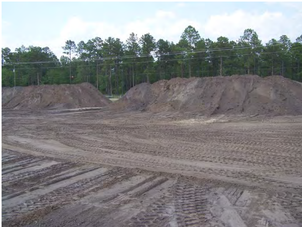
Inspected clean soil stockpiled at the east side of the South Pond site
