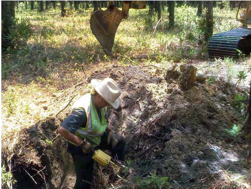
Equipment assist team inspecting anomalies deeper than 1 ft
