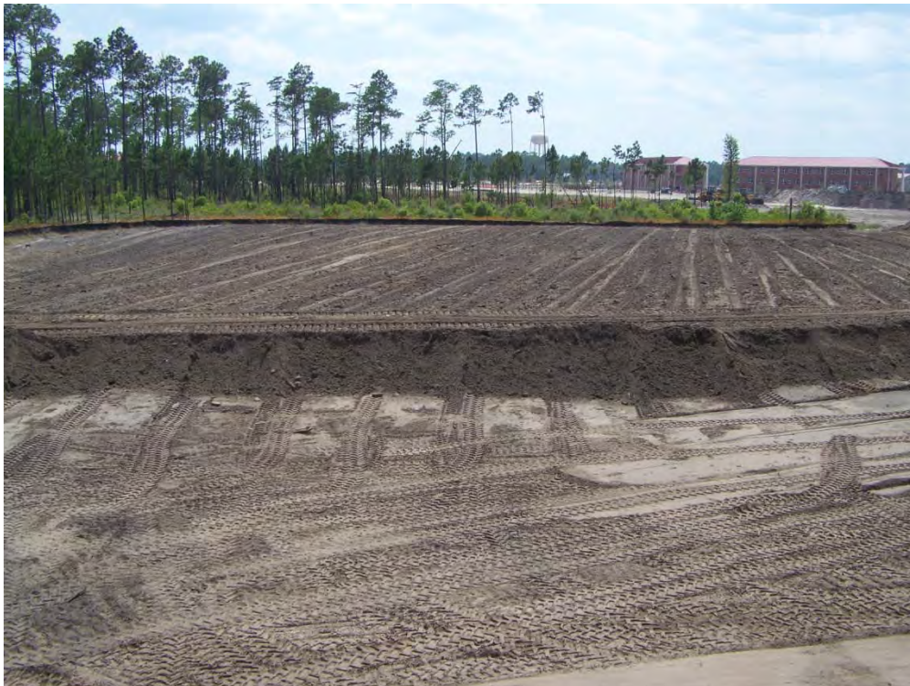
Current progress at the South Pond site
