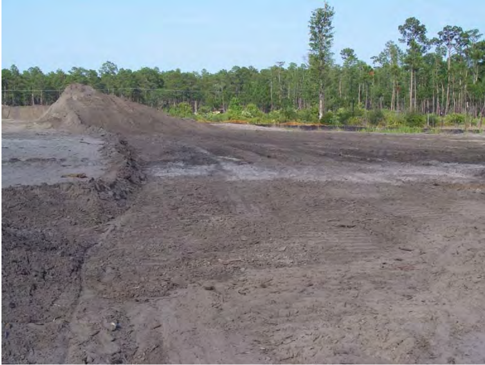
Cut to the original contours on the west side of the South Pond site
