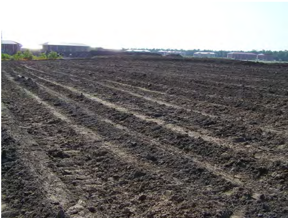
Remaining area at the South Pond site to clear
