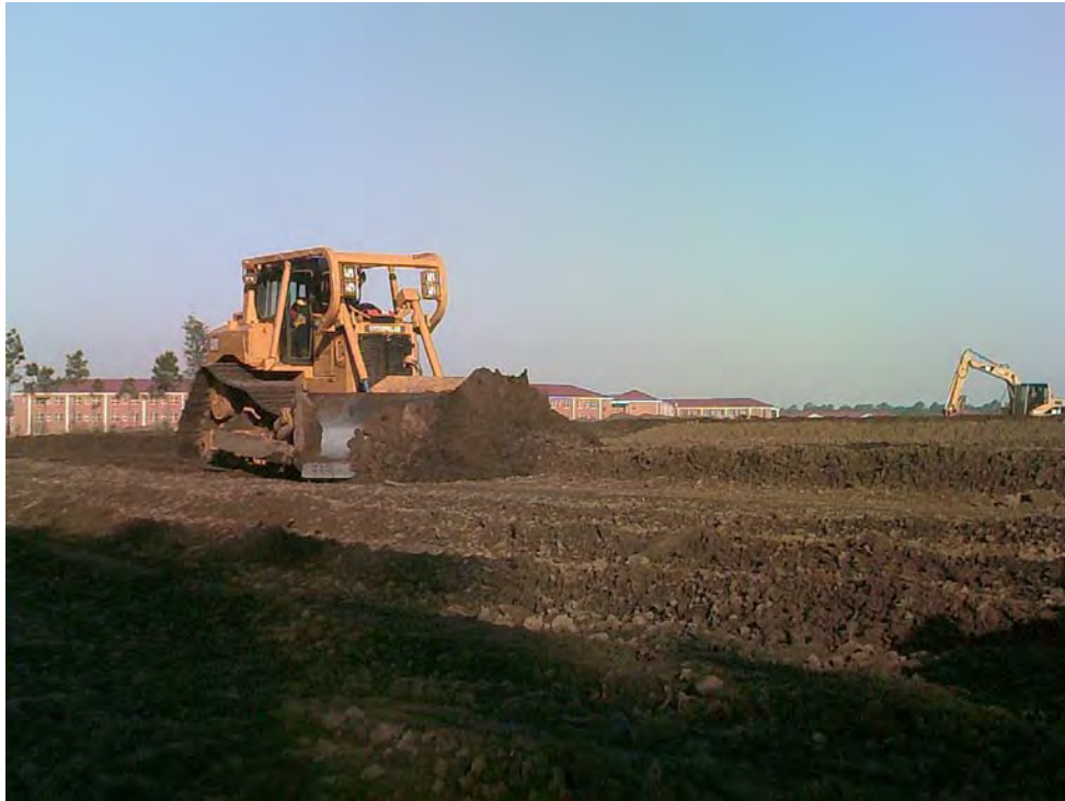
D6 CAT dozer working South Pond area
