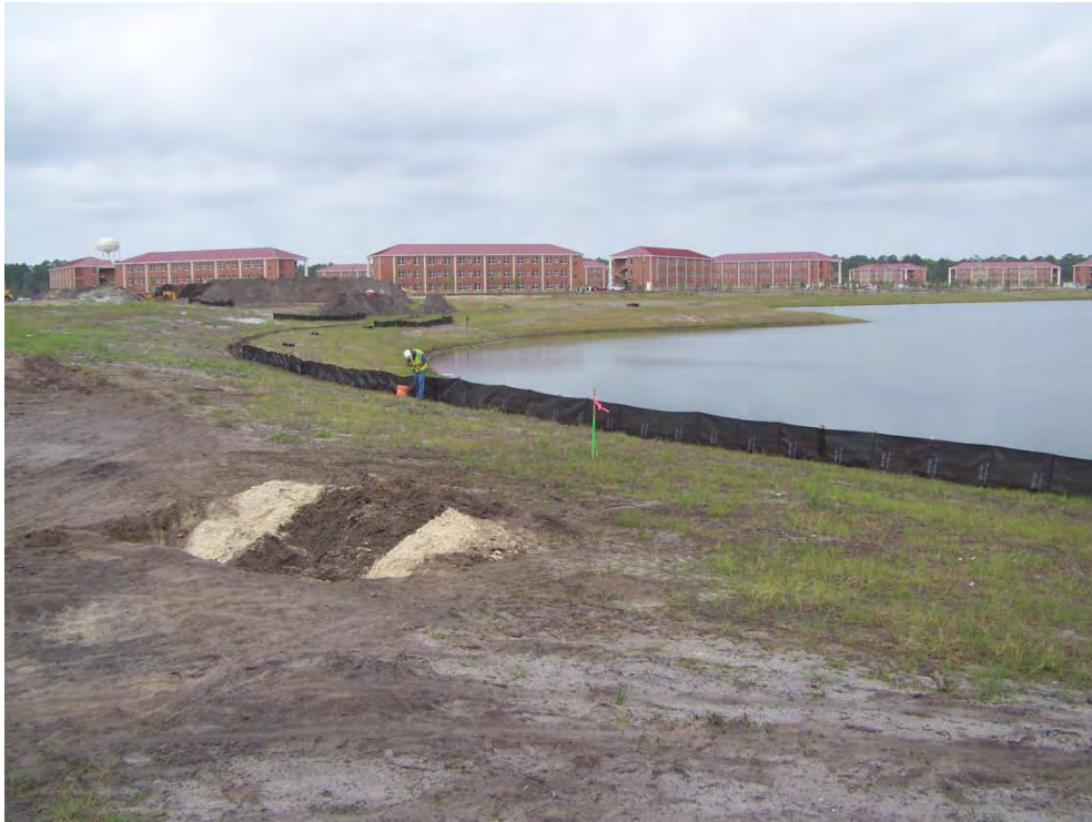
Installation of the silt fence at the South Pond site
