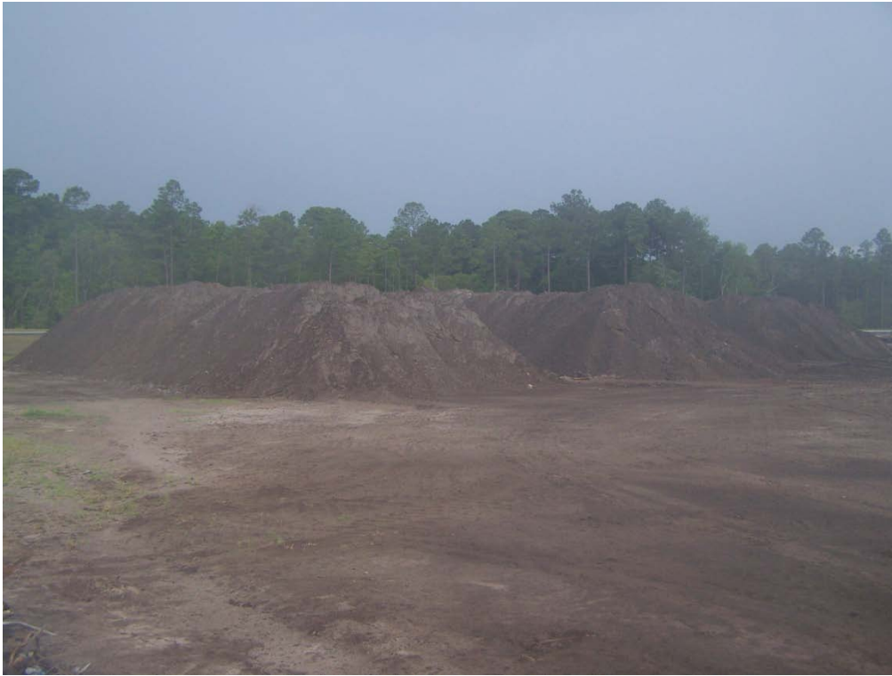
The 5300.4 cys of dirt moved at the HHQ site
