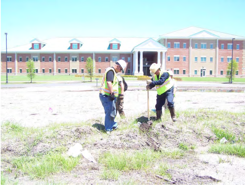
Sweep of the upper shelf at the HHQ site.
