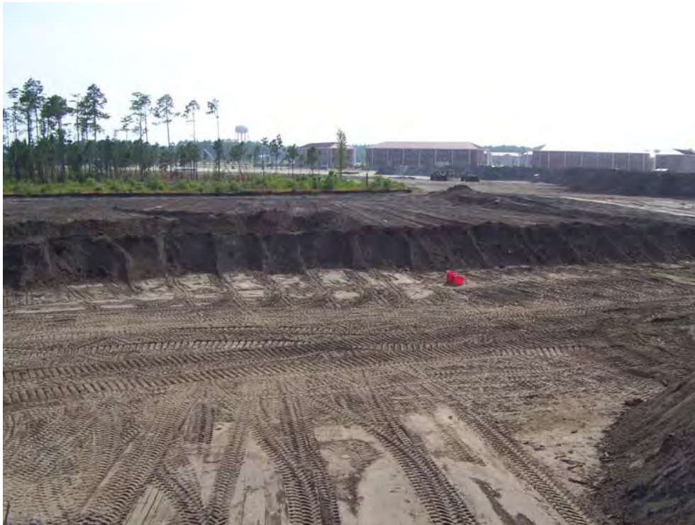
Current progress as the South Pond site
