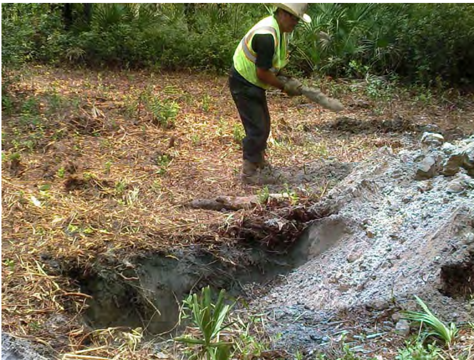
Equipment assisted operations investigating anomalies deeper than 1ft
