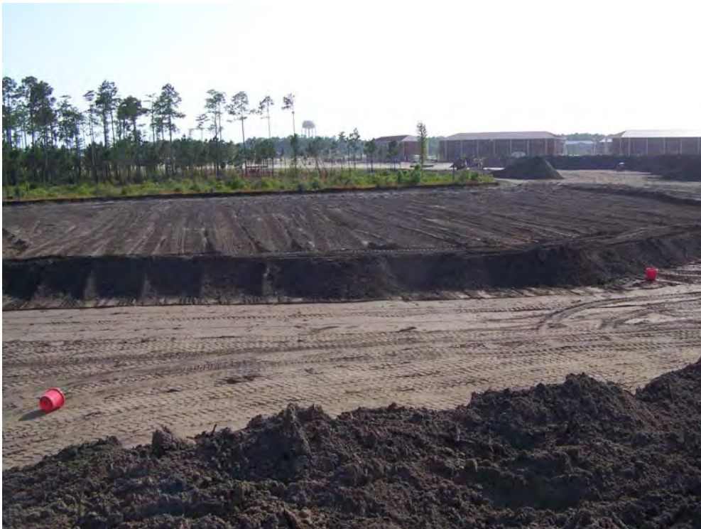
Current progress at the South Pond site
