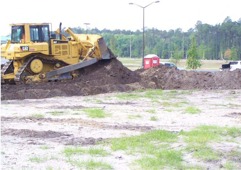
D6 CAT dozer working upper shelf at HHQ site.
