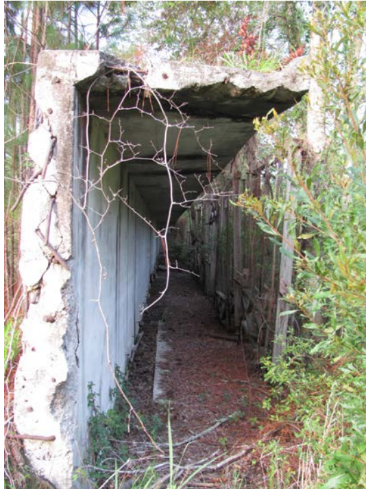
Figure 4-11: Behind Concrete Wall with Wood Target Frames
