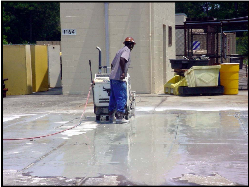
Cutting concrete for removal
