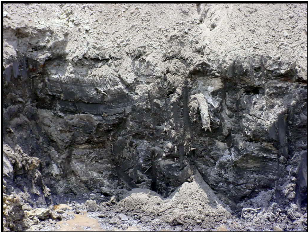
ORC® applied to walls and bottom of excavation
