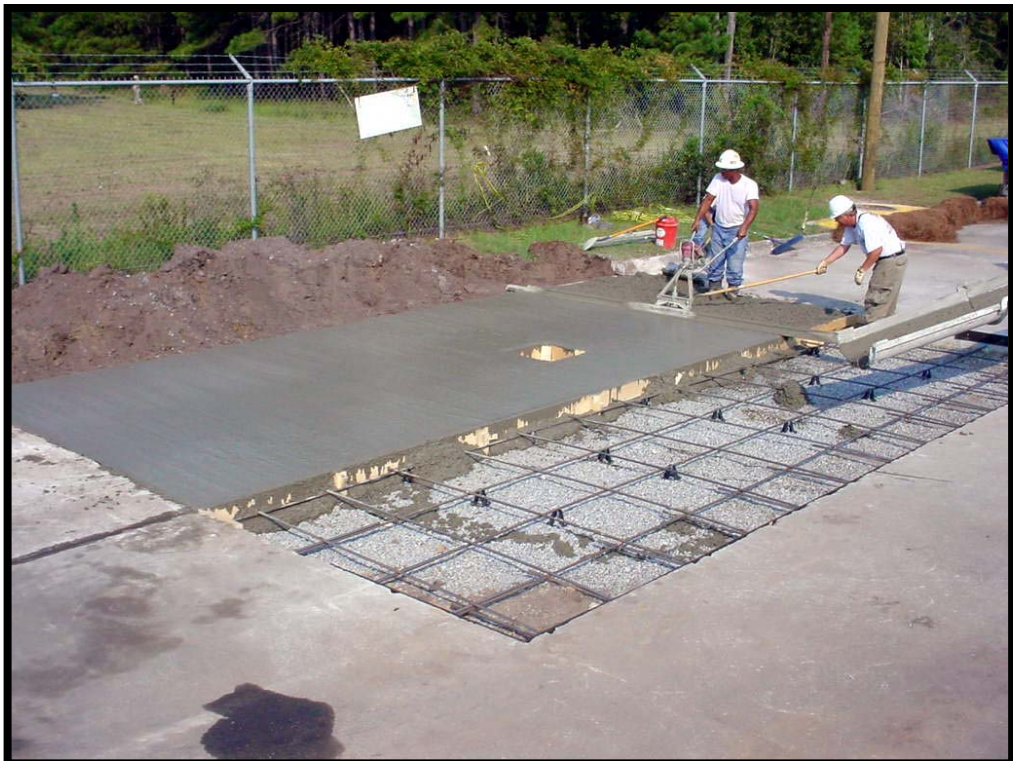
Placing and finishing concrete
