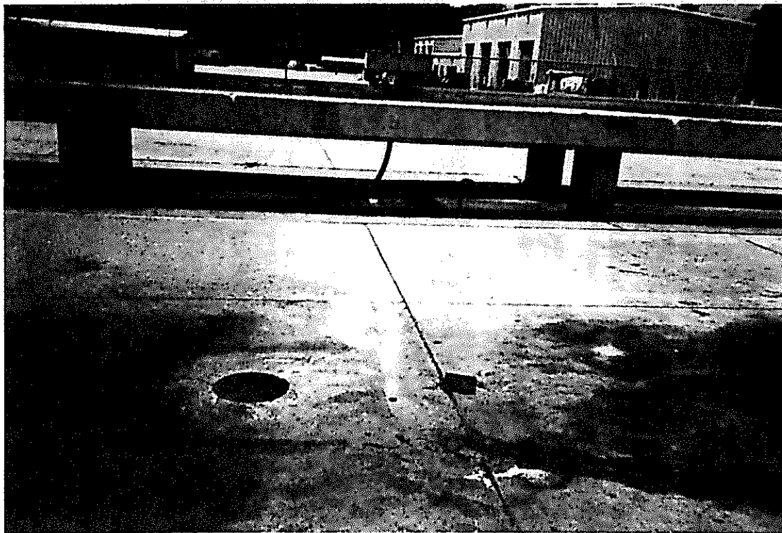
Photo 1. The Tank 38 site prior to removal.
