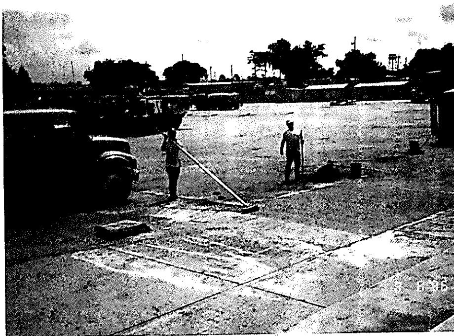
Photo 2. The Tank 38 site after tank removal.
