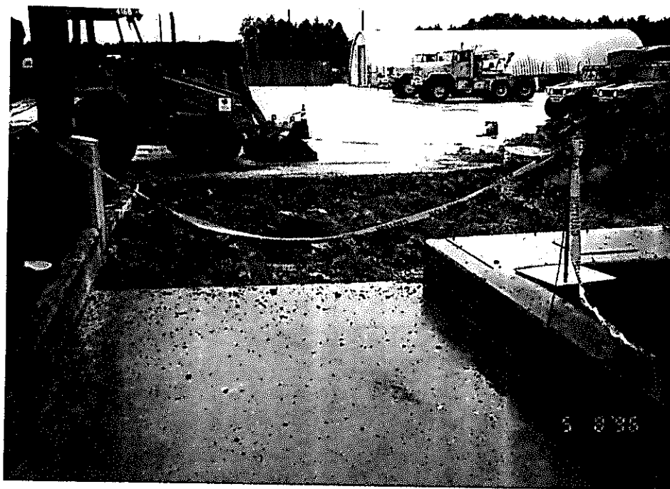
Photo 1. Concrete broken over Tank 238.
