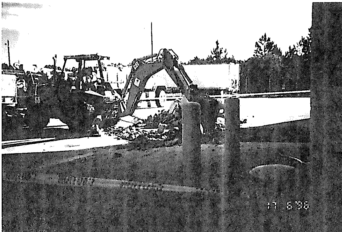
Photo 1. The site during concrete breaking and removal.
