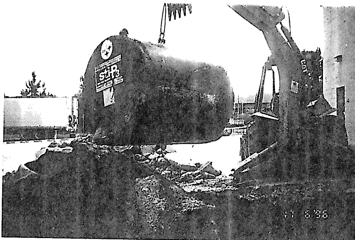
Photo 2. The tank being removed from the excavation.
