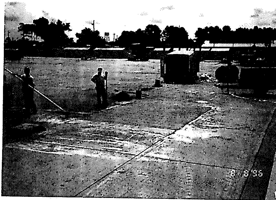
Photo 3. Photograph of a fresh concrete slab being finished over the tank pit.
