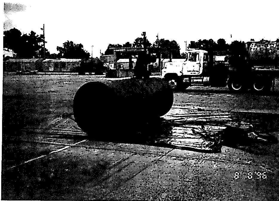
Photo 2. Tank 216 after removal from the tank pit.
