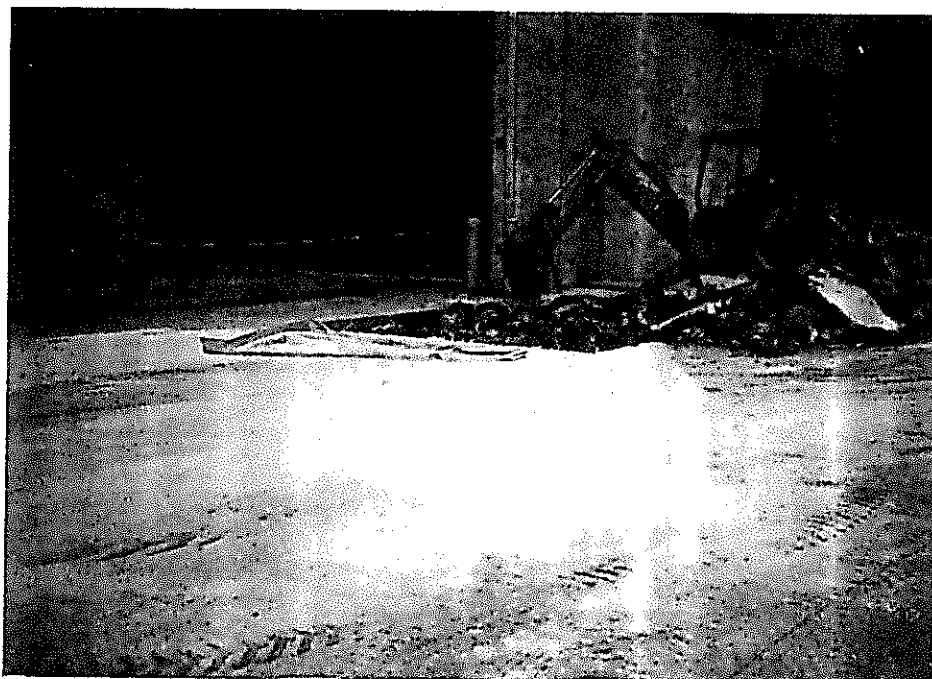
Photo 2. Concrete above Tank 201A being removed.
