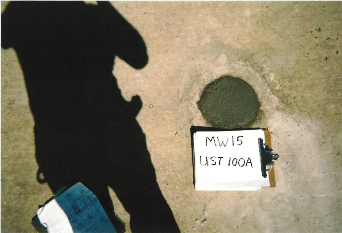
UST 100A: Well Abandonment – MW15
