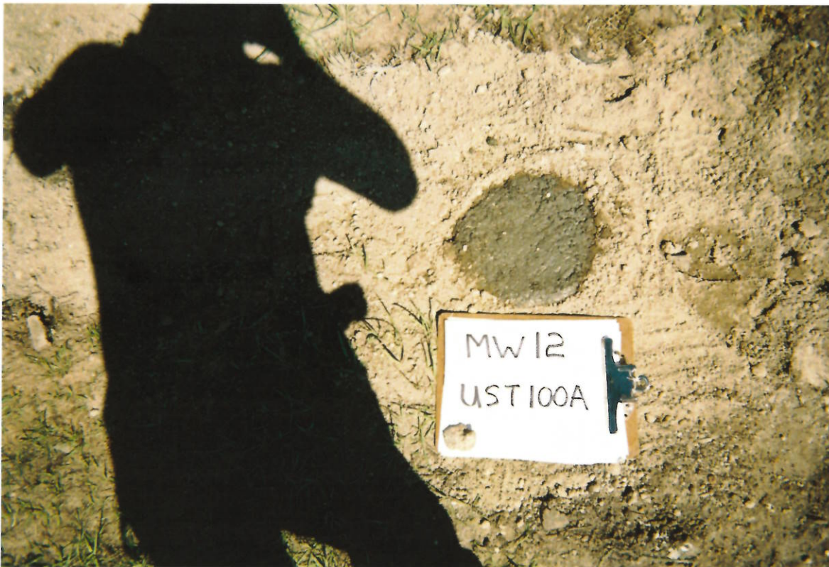
UST 100A: Well Abandonment – MW12
