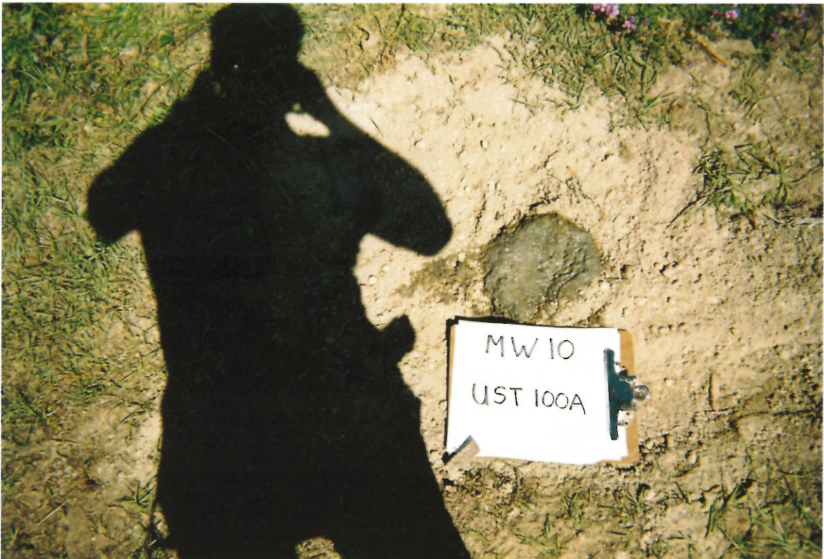
UST 100A: Well Abandonment – MW10
