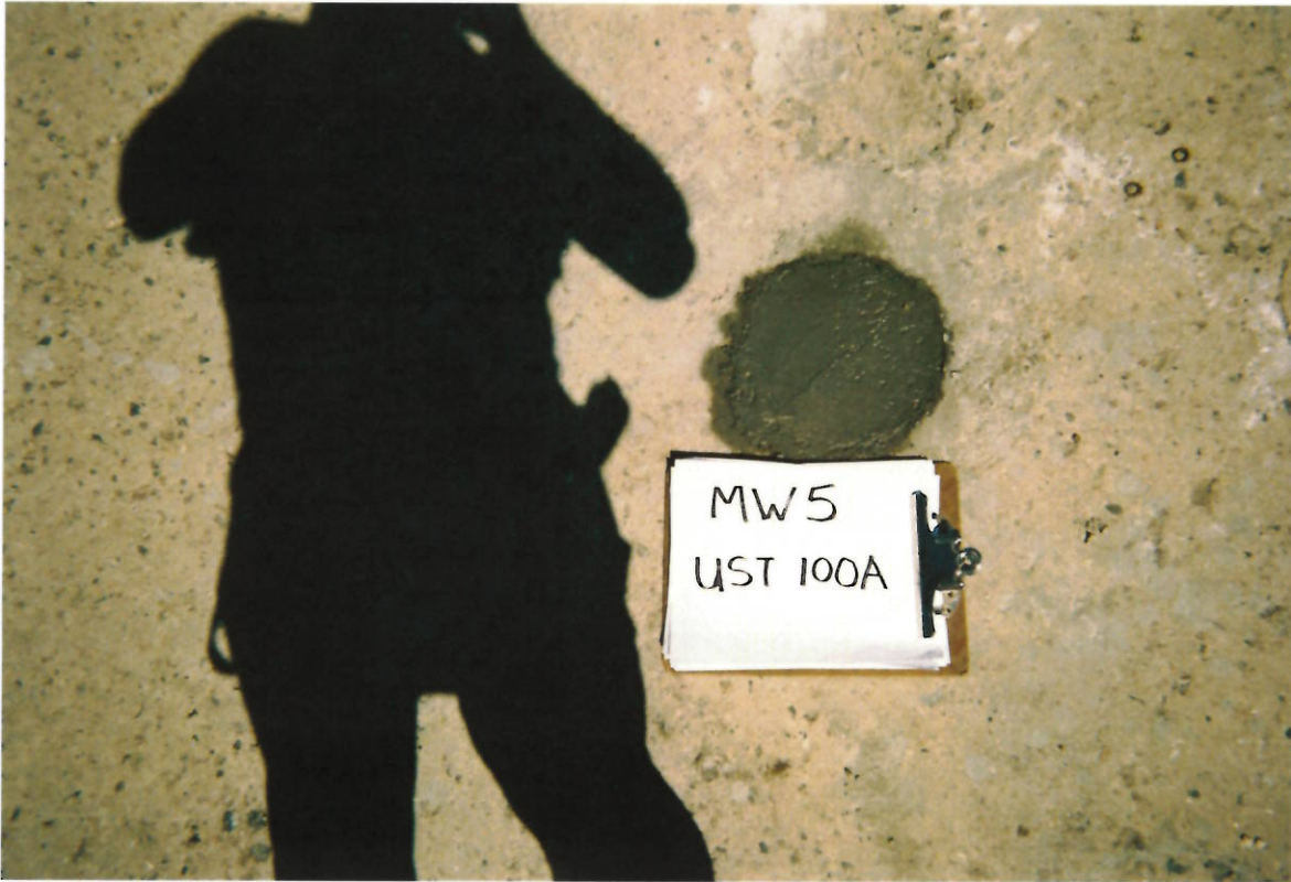
UST 100A: Well Abandonment – MW5
