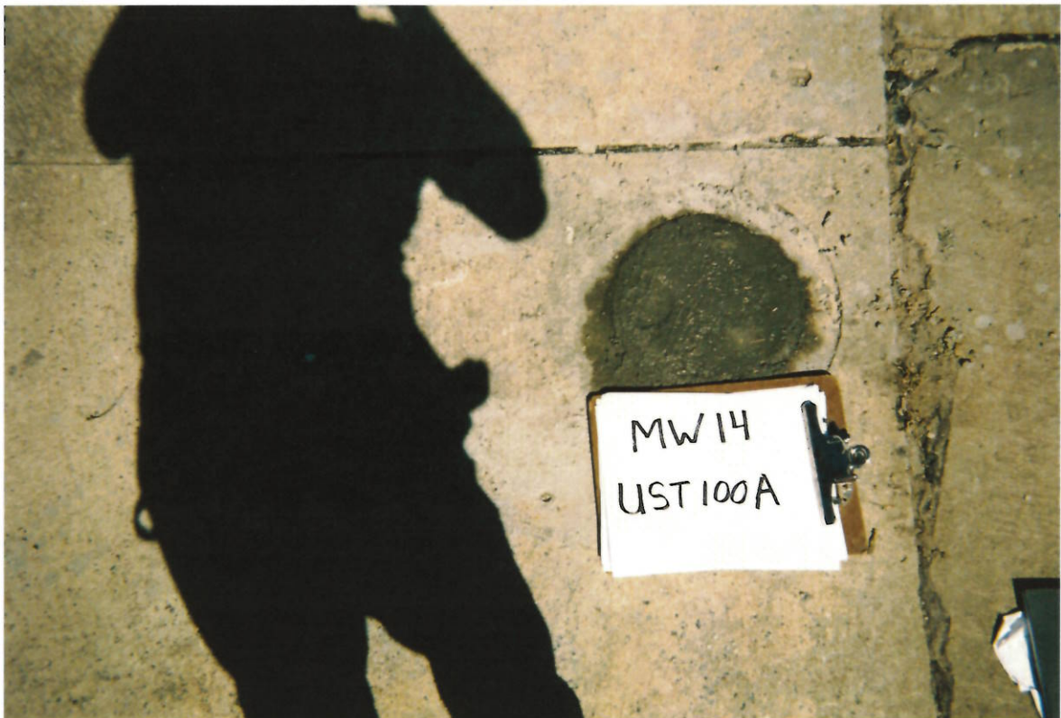
UST 100A: Well Abandonment – MW14
