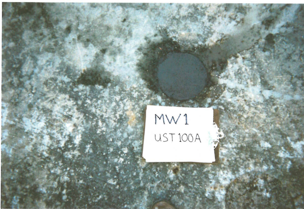
UST 100A: Well Abandonment – MW1
