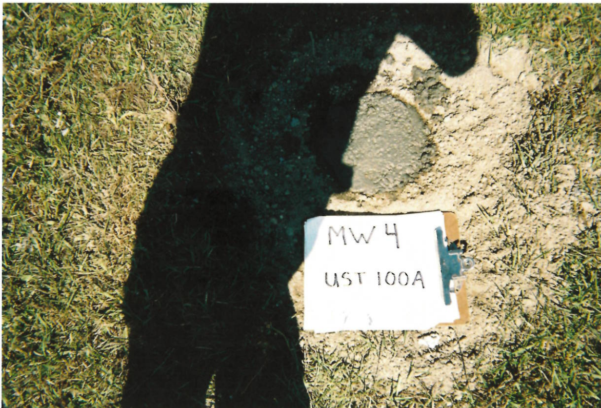
UST 100A: Well Abandonment – MW4
