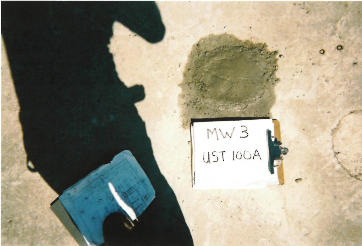
UST 100A: Well Abandonment – MW3
