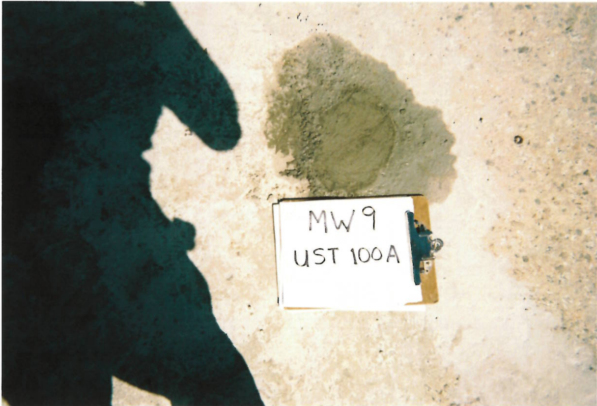
UST 100A: Well Abandonment – MW9
