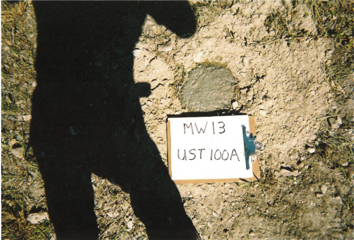
UST 100A: Well Abandonment – MW13
