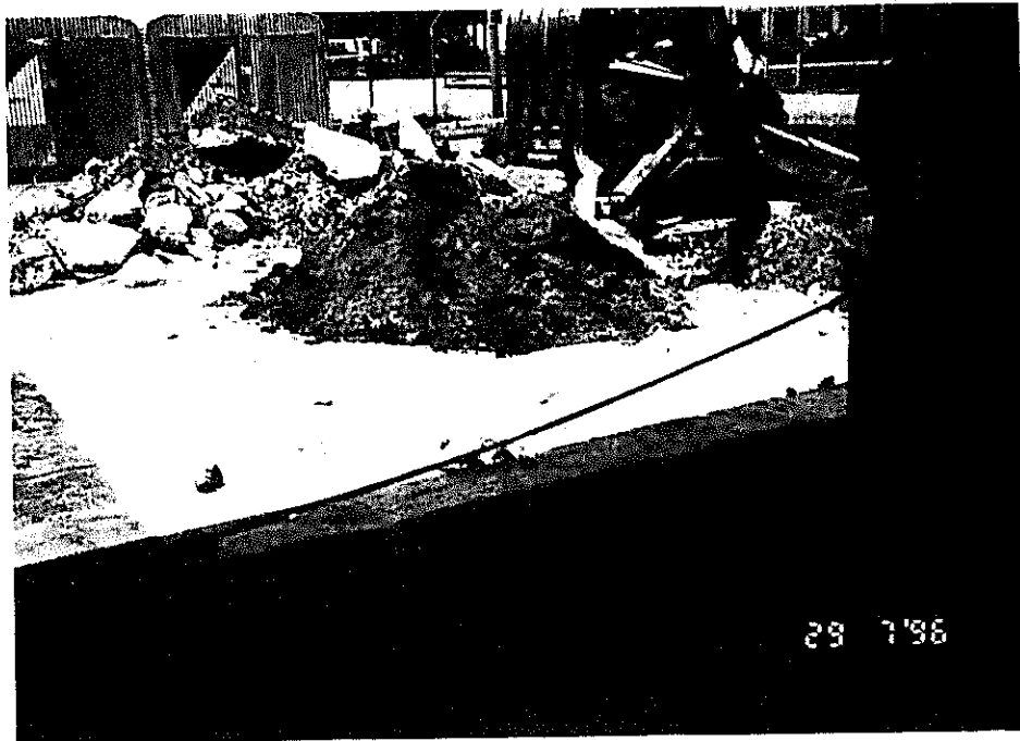
Photo 1. Concrete over Tank 94C being removed.
