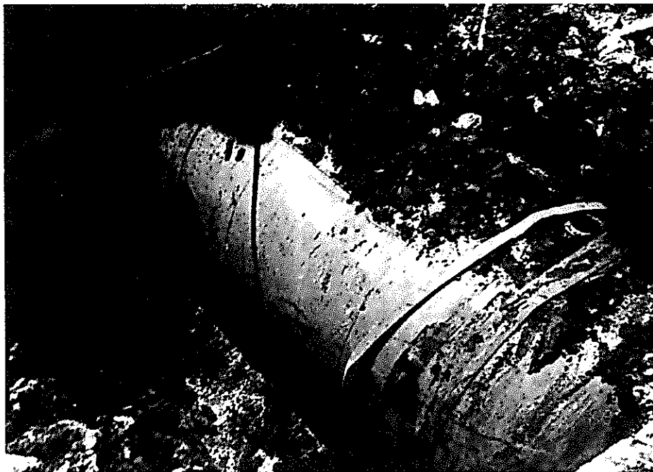
Photo 2. Tank 74 being uncovered.
