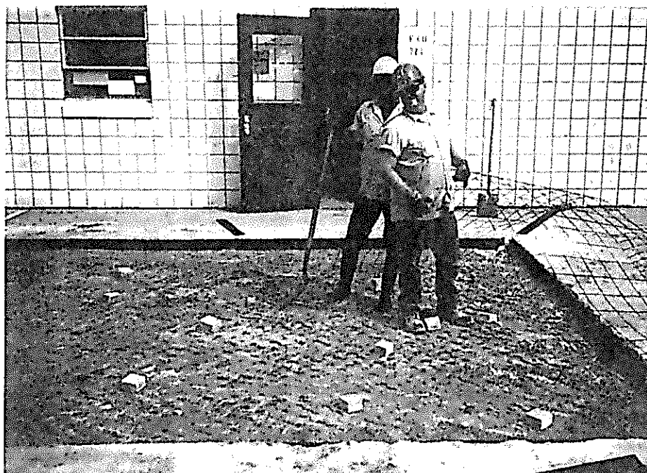
Photo 2. ACE concrete experts prepare to pour a fresh slab over tank pit.
