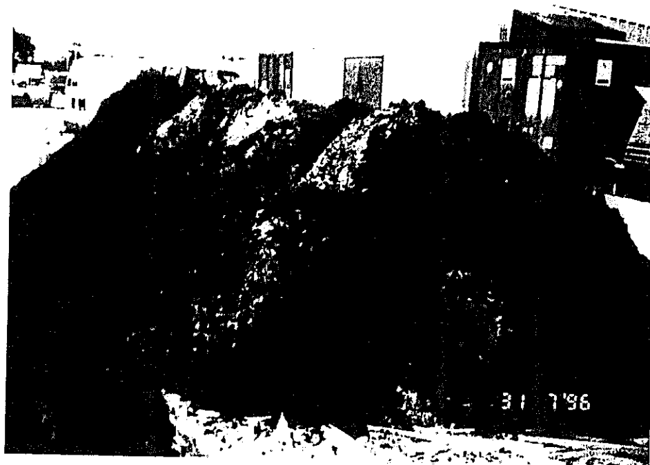
Photo 3. Clean soil that was excavated during the tank removal process.
