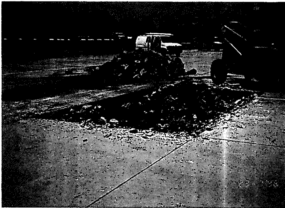
Photo 1. Concrete over Tank 93 being broken and removed.
