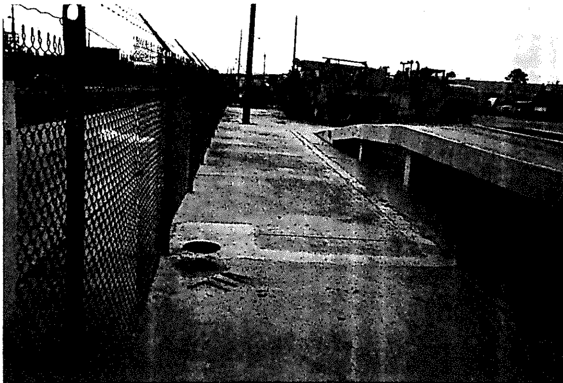
Photo 1. The Tank 71A site prior to tank removal.
