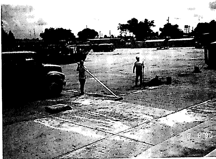
Photo 2. The Tank 38 site after tank removal.
