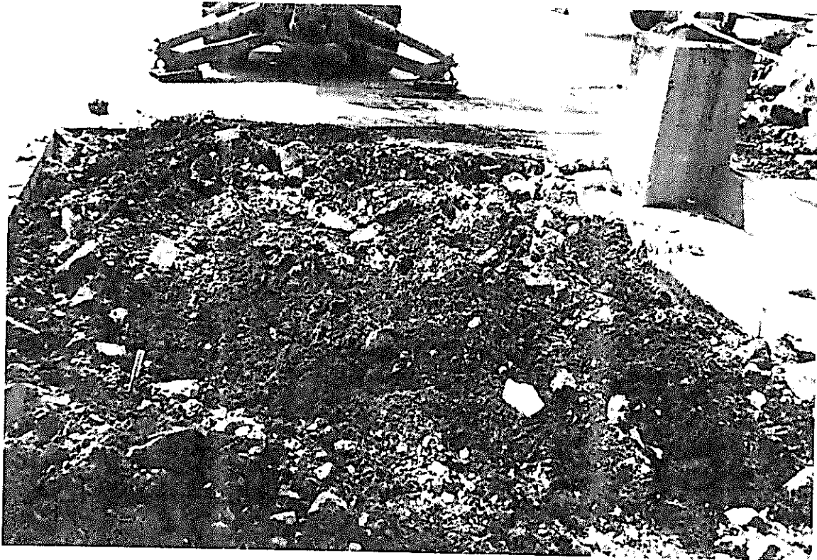
Photo 1. Tank pit after concrete breaking and removal.
