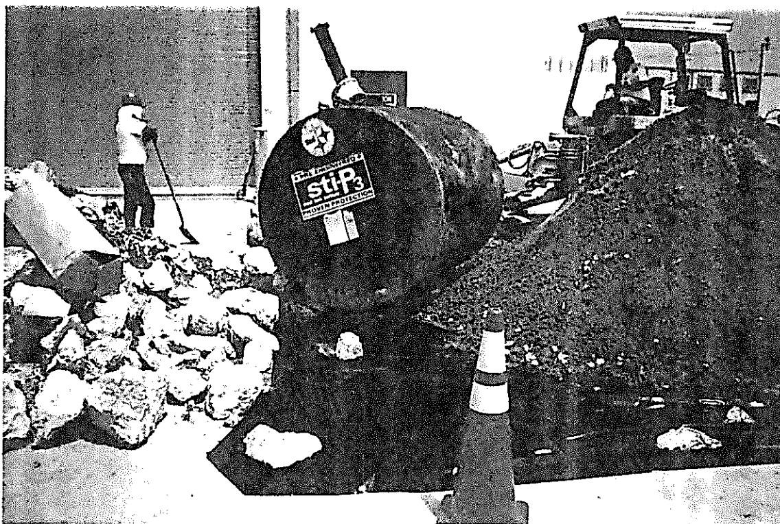
Photo 2. Tank 28B after removal from the tank pit.
