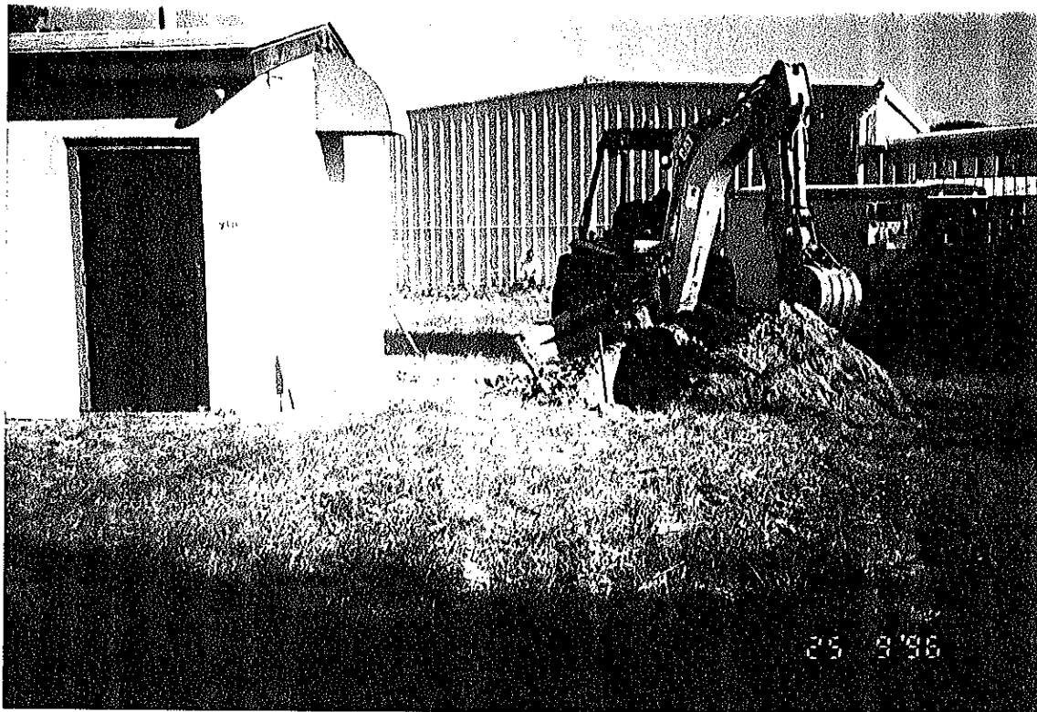
Photo 1. Beginning excavation of tank 116.
