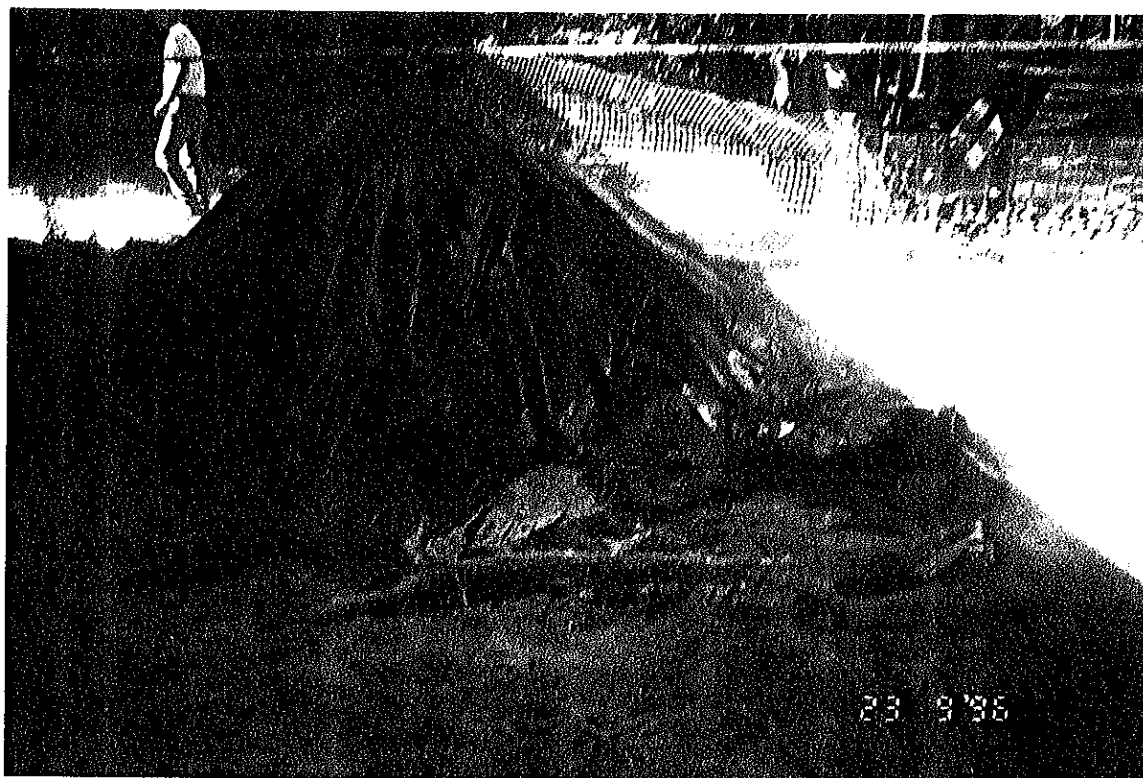
Photo 3. Petroleum contaminated soil stockpile at the Tank 112 site.
