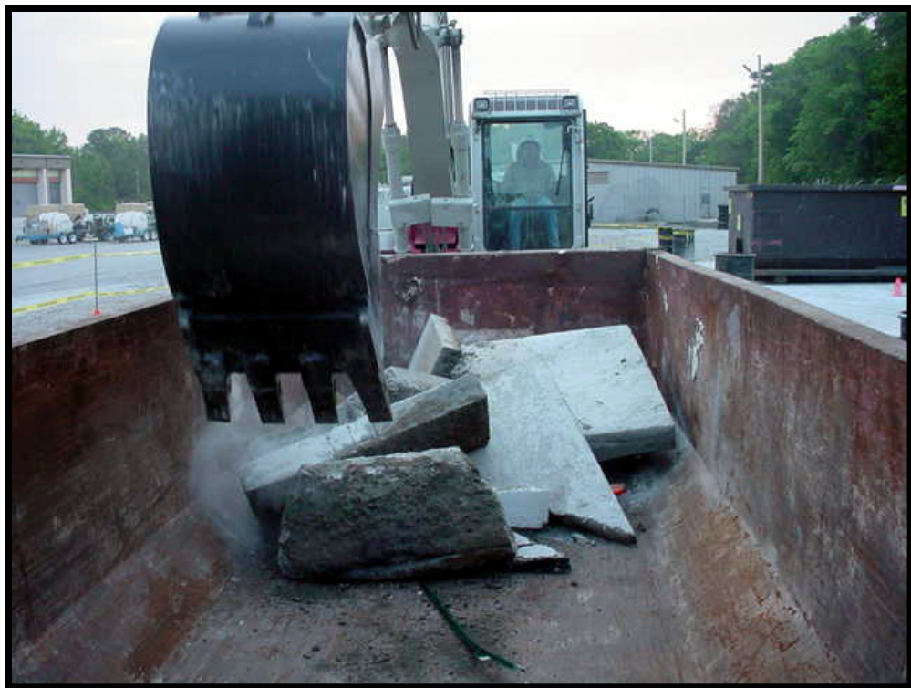
Placing concrete in roll-off for disposal
