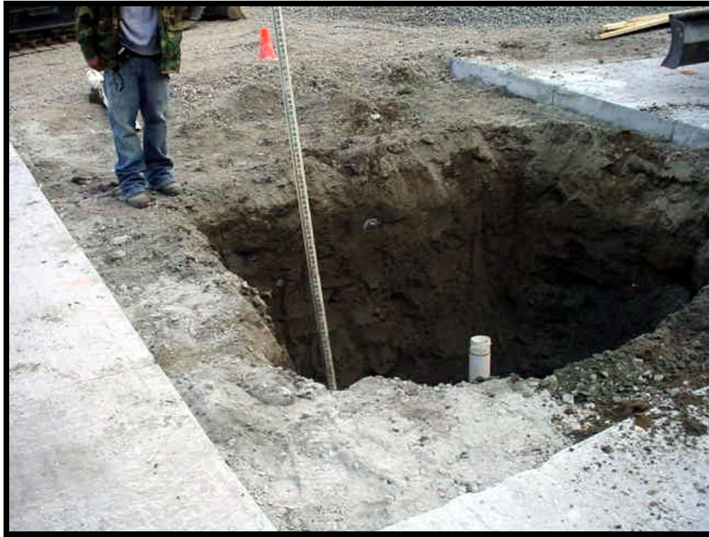
Excavation at well AF-12
