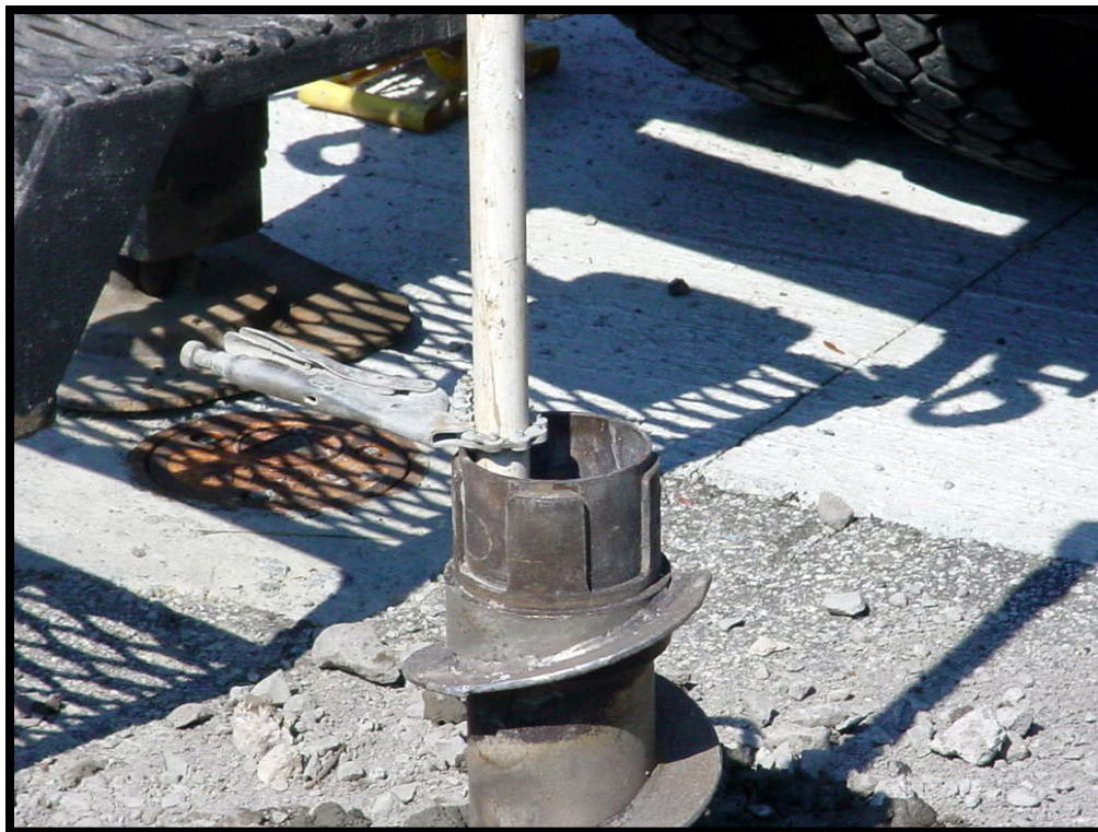
Grouting well AF-40 with Tremie Pipe
