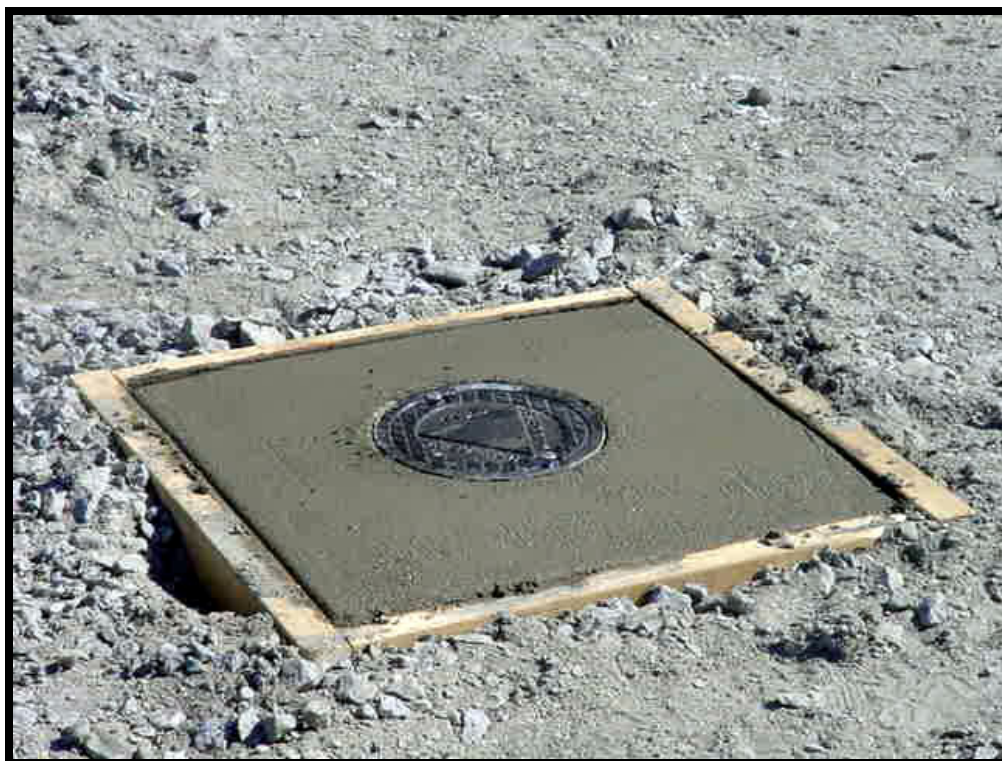
Finishing well pad at AF-07R
