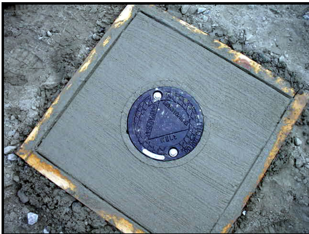
Finishing well pad at AF-12R
