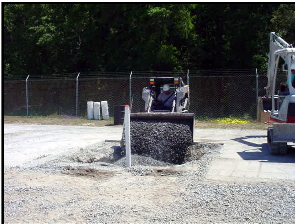
Backfilling around well AF-07R
