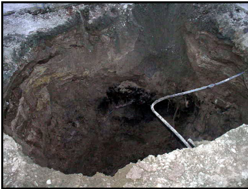
Well AF-07 Excavation
