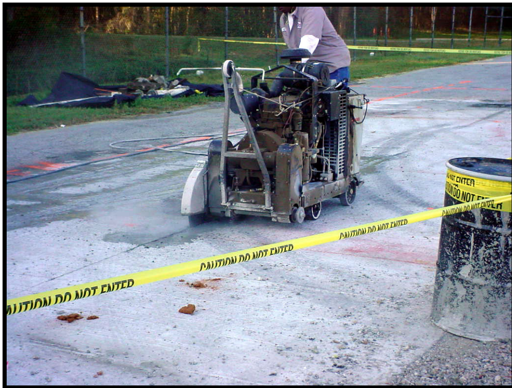
Cutting concrete
