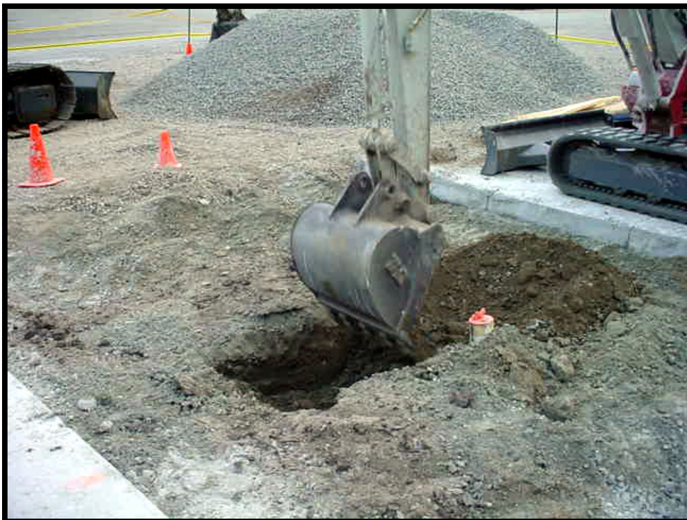
Excavating well AF-12
