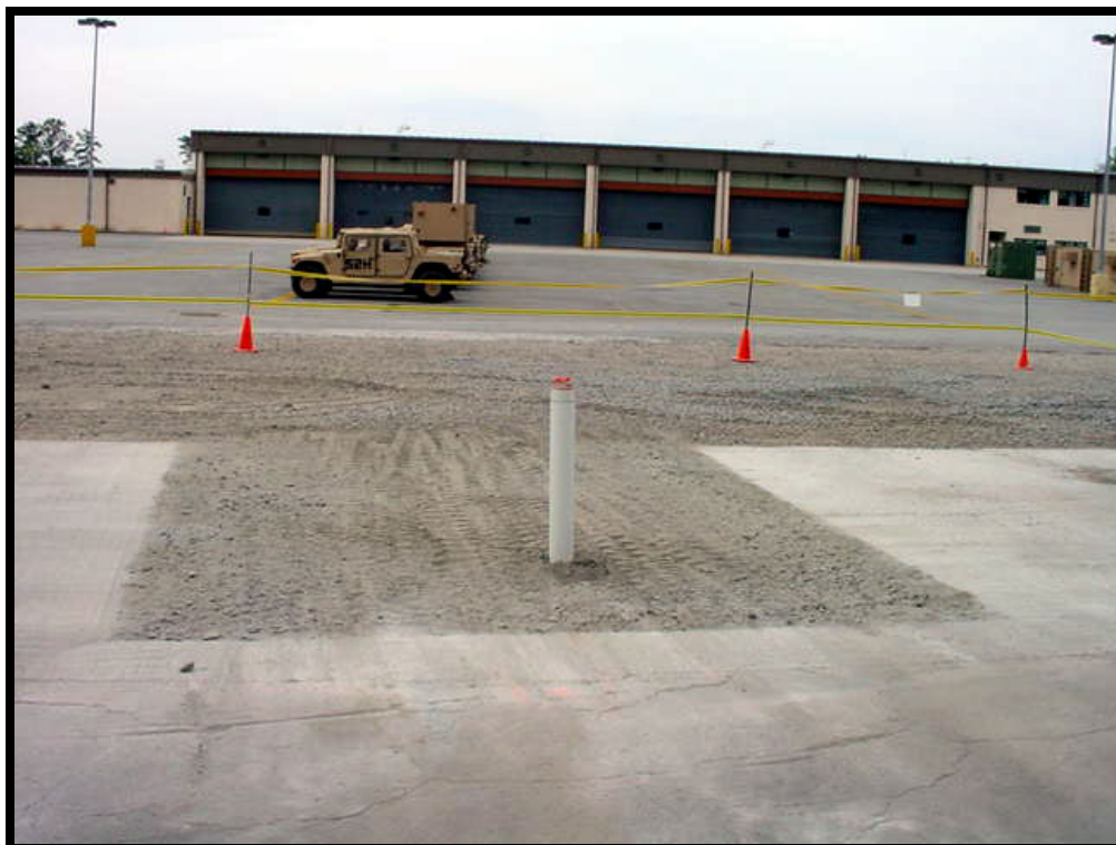
Excavation backfilled at well AF-12R
