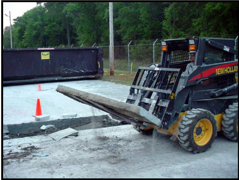
Removing concrete
