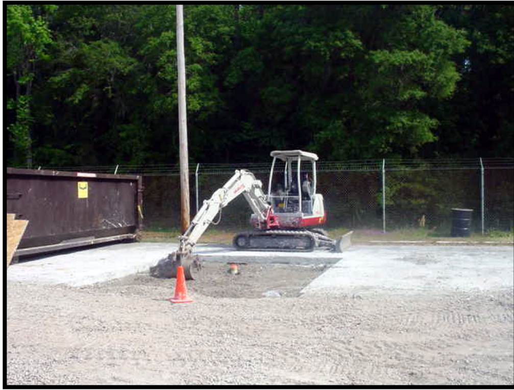
Excavating Well AF-07
