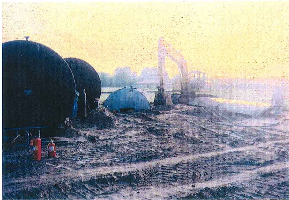
PDO Yard: PDO Yard during removal of tanks.
