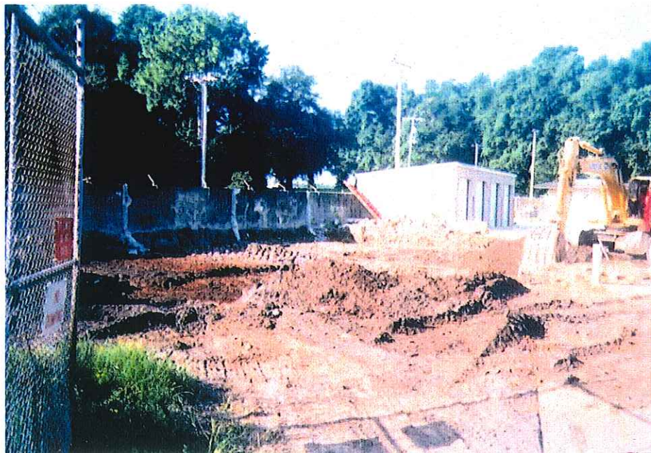
PDO Yard: PDO Yard after removal of tanks.
