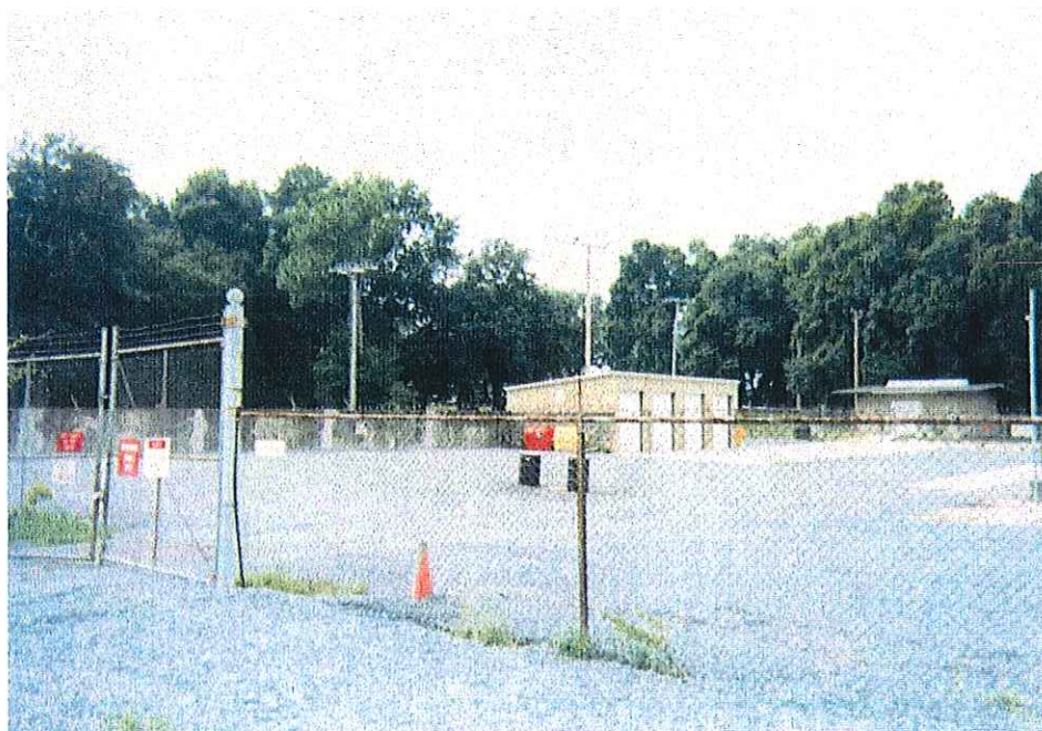
PDO Yard: PDO Yard after site restoration.
