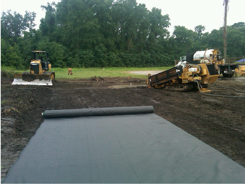
07/27/11: Geotextile liner (foreground) placed beneath the gravel pad for the MPE/injection system trailer. Horizontal boring rig (background) used to install the effluent line beneath Lamar Canal
