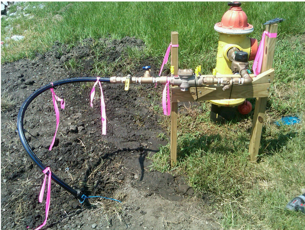
07/30/11: Connection to water supply
