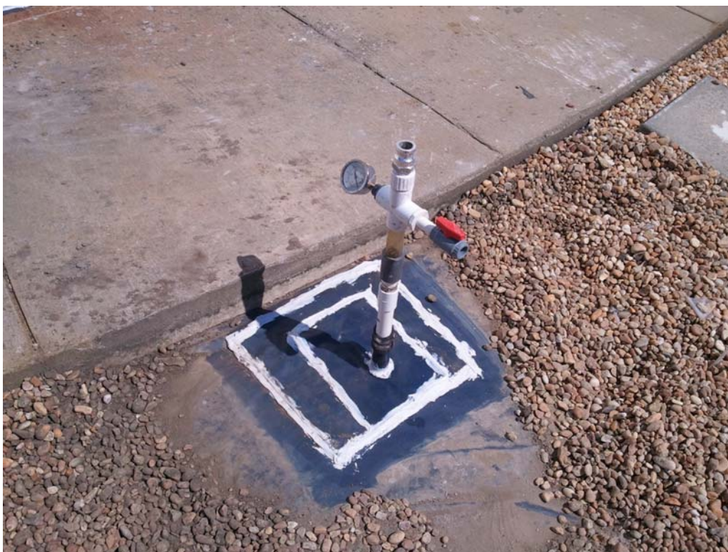
09/09/11: Completed replacement injection well BFF-7JR
