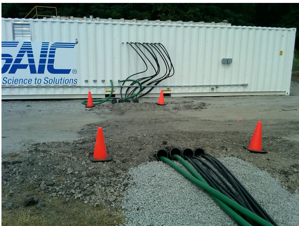
08/03/11: Injection and extraction lines lead from the MPE/injection system to wells encircling AST 7009 within the BFF
