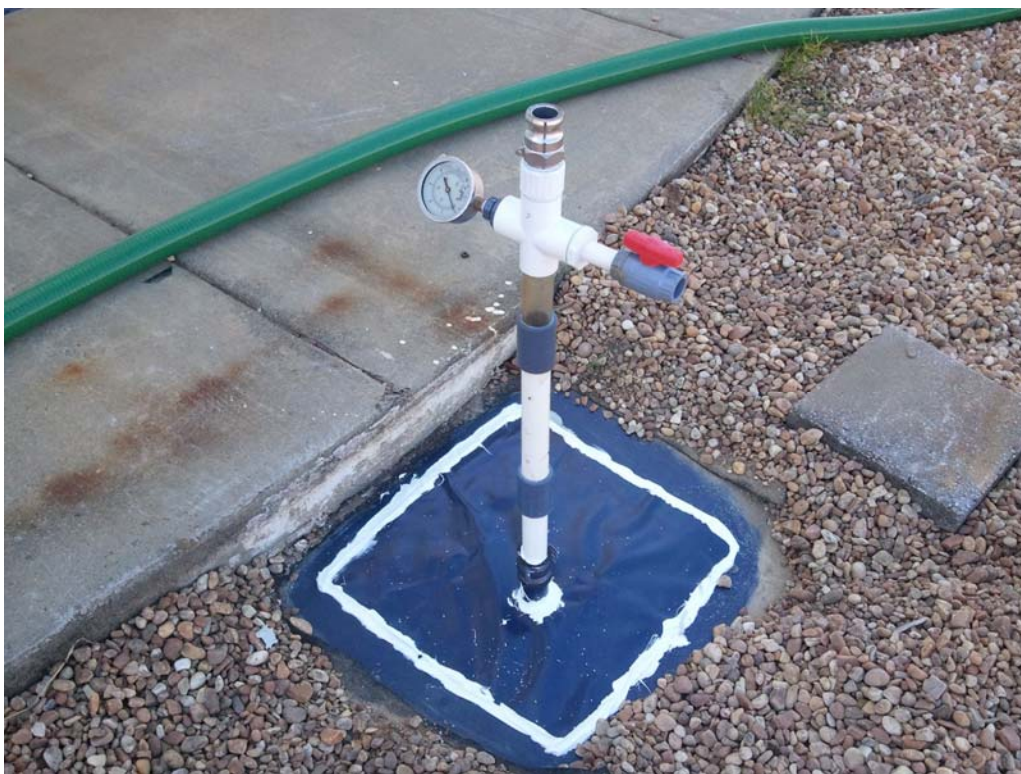
09/09/11: Completed replacement injection well BFF-3JR
