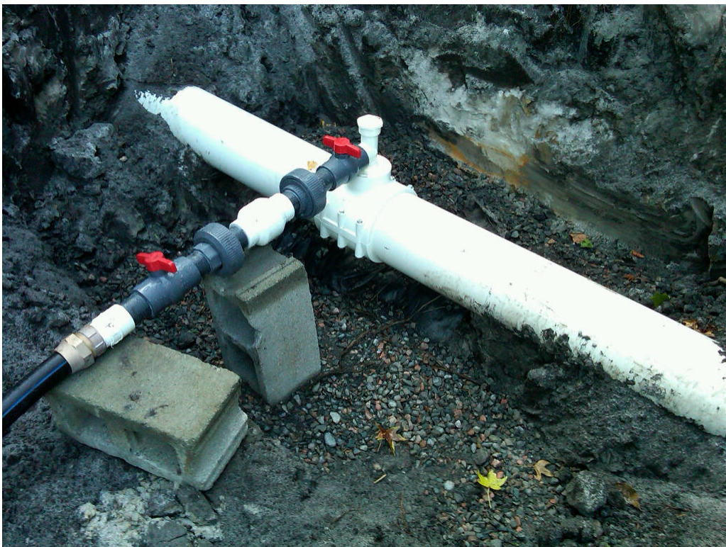
08/01/11: Connection of treatment discharge line to the sewer line leading to the Hunter WWTP
