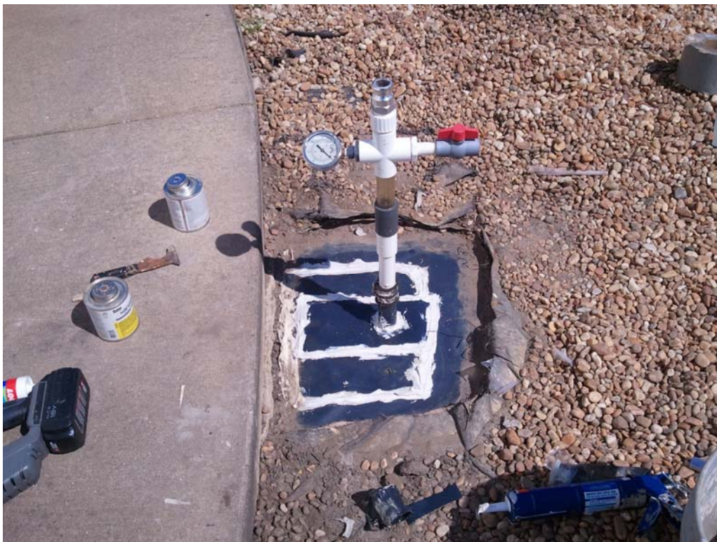
09/09/11: Completed replacement injection well BFF-2JR
