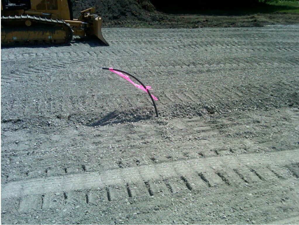
07/30/11: Water supply line for the MPE/injection system trailer following completion of the gravel pad but prior to arrival of the trailer
