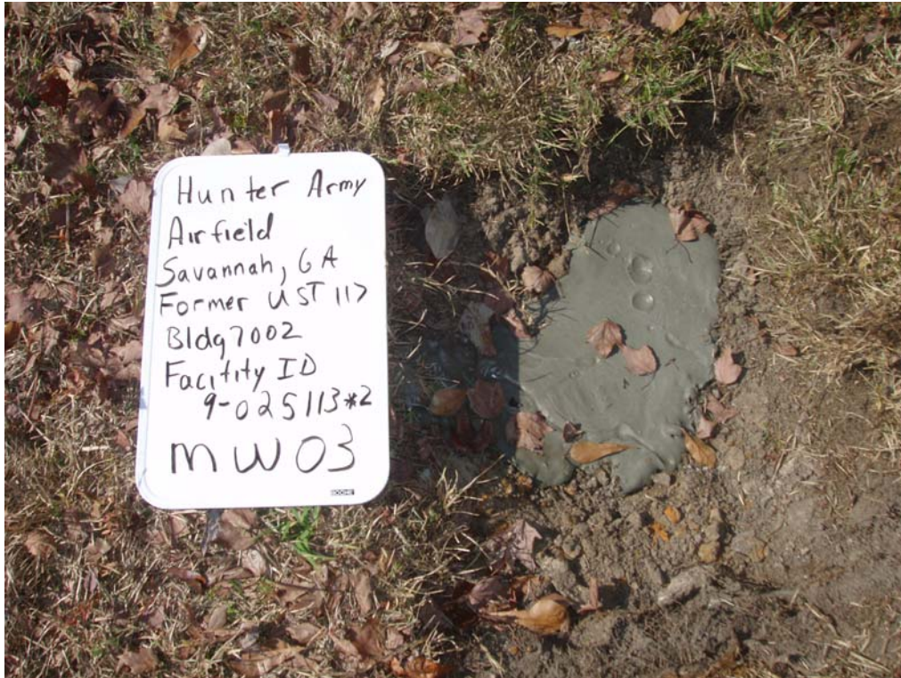
Bulk Fuel Facility (UST 117): Well Abandonment – MW-03
