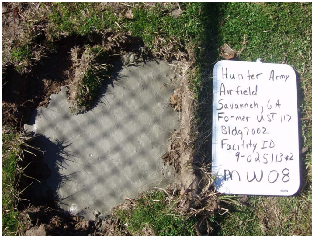
Bulk Fuel Facility (UST 117): Well Abandonment – MW-08
