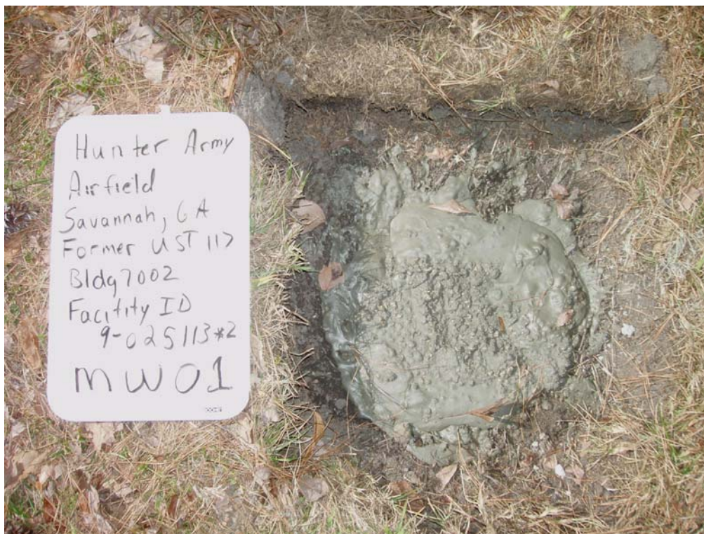
Bulk Fuel Facility (UST 117): Well Abandonment – MW-01
