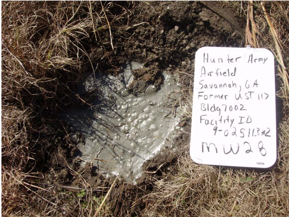
Bulk Fuel Facility (UST 117): Well Abandonment – MW-28
