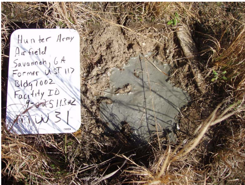
Bulk Fuel Facility (UST 117): Well Abandonment – MW-31
