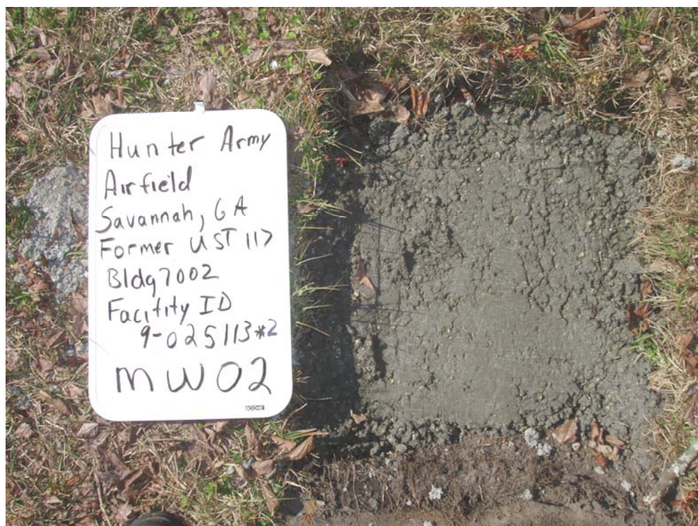
Bulk Fuel Facility (UST 117): Well Abandonment – MW-02
