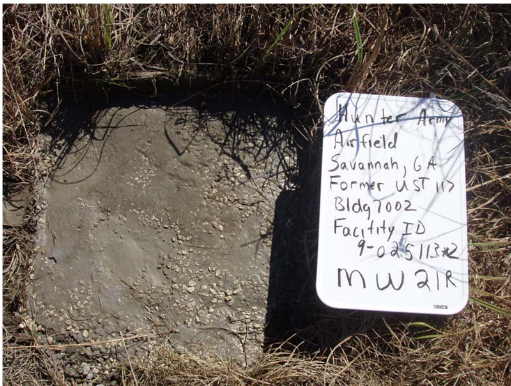
Bulk Fuel Facility (UST 117): Well Abandonment – MW-21R
