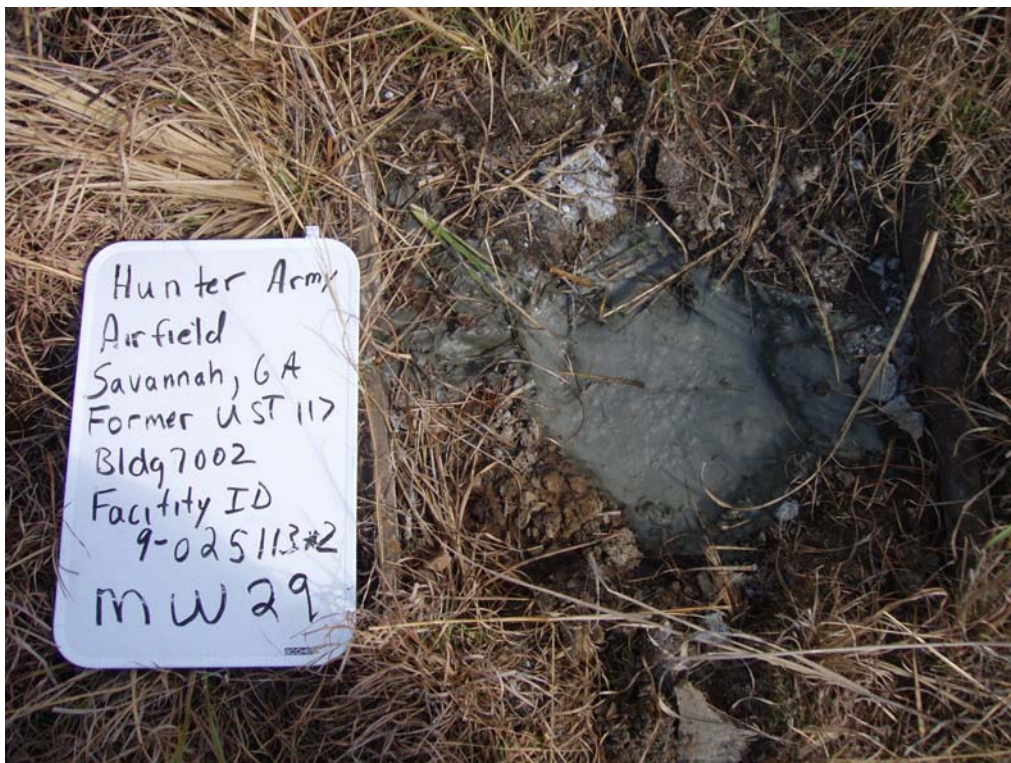
Bulk Fuel Facility (UST 117): Well Abandonment – MW-29
