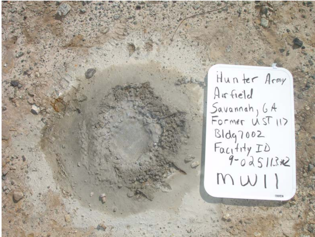
Bulk Fuel Facility (UST 117): Well Abandonment – MW-11
