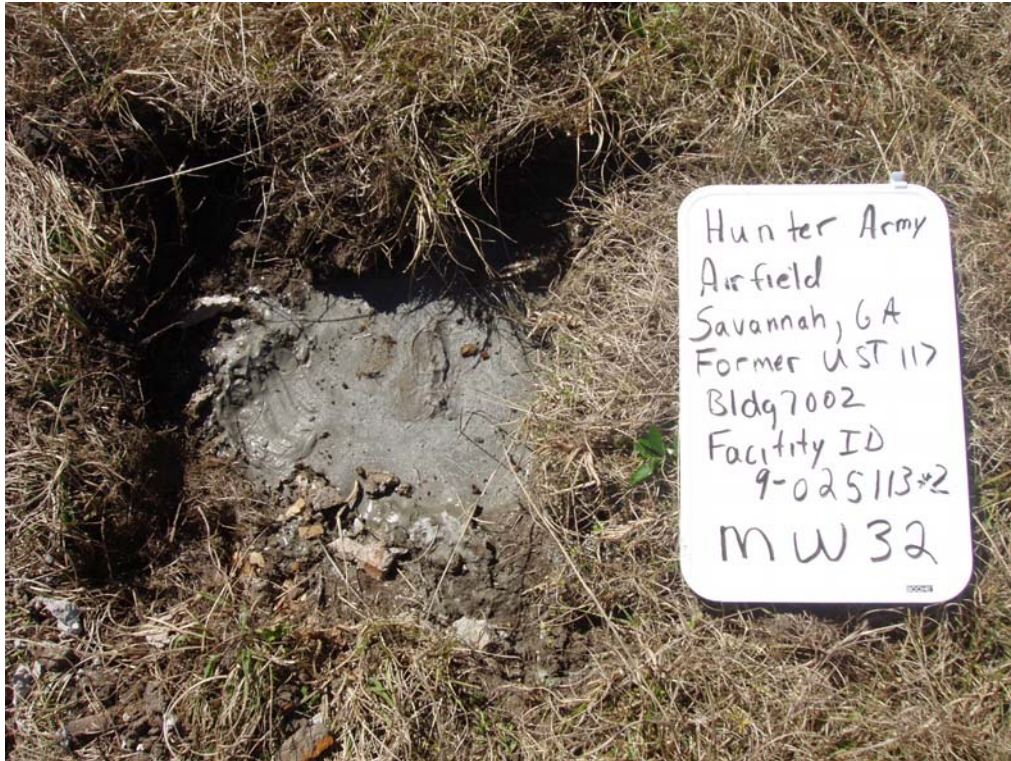
Bulk Fuel Facility (UST 117): Well Abandonment – MW-32
