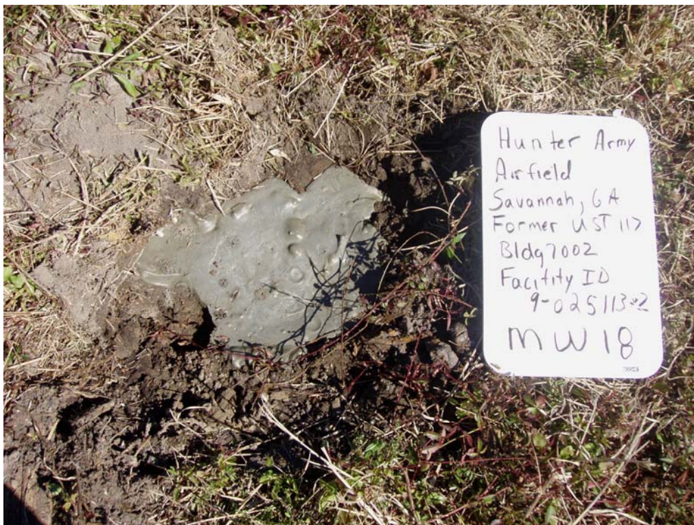
Bulk Fuel Facility (UST 117): Well Abandonment – MW-18
