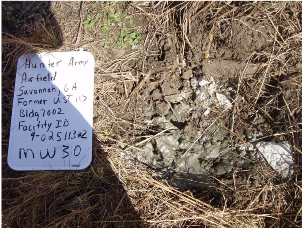
Bulk Fuel Facility (UST 117): Well Abandonment – MW-30
