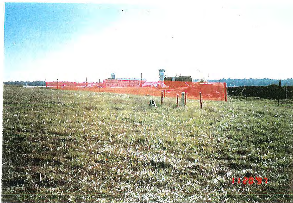
PHOTOGRAPH -20- PERIMETER FENCE INSTALLATION
