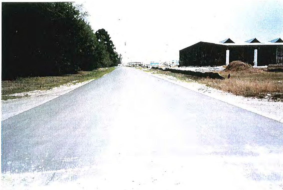
PHOTOGRAPH -100- STRACHAN ROAD (truck haul route)
