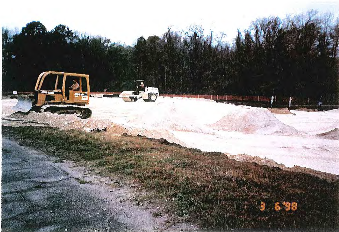
PHOTOGRAPH -91- BACKFILL ACTIVITIES
