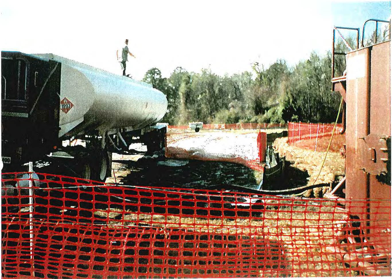
PHOTOGRAPH -76- REMOVAL OF GENERATED WASTEWATER
