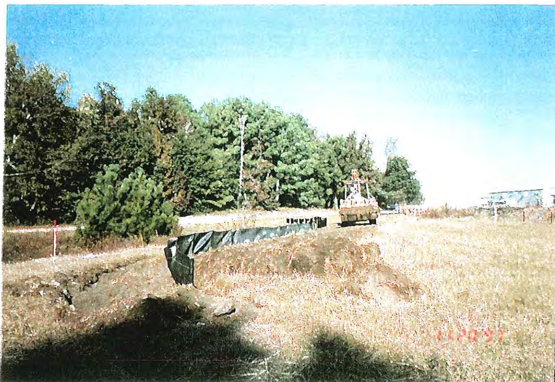
PHOTOGRAPH -19- SILT FENCE INSTALLATION
