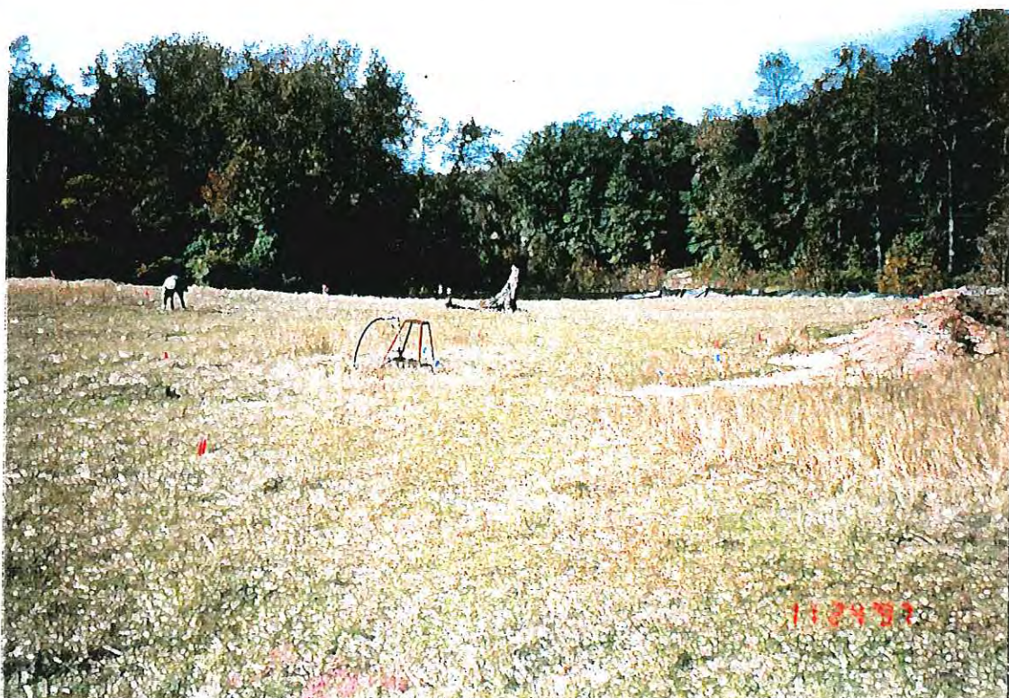
PHOTOGRAPH -29- MARKING OF ON-SITE UTILITIES
