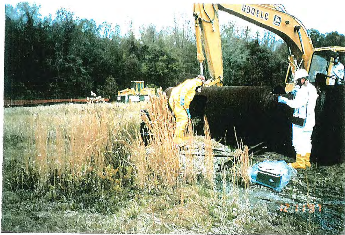
PHOTOGRAPH -41- SIMULATED AIRCRAFT TANK CLEANING
