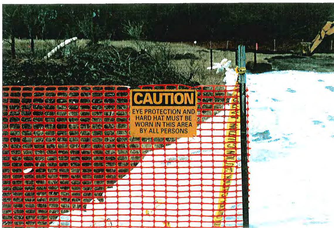
PHOTOGRAPH -38- PERIMETER FENCE SITE SIGN
