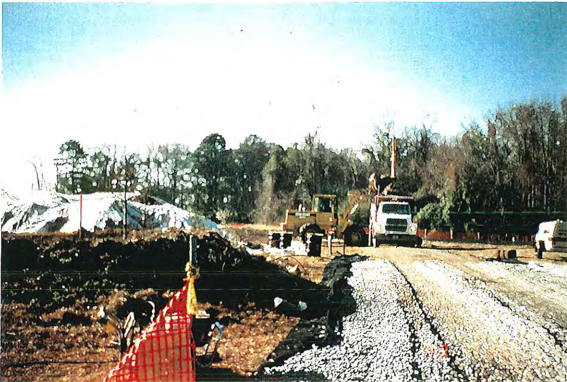
PHOTOGRAPH -58- LOADING OF EXCAVATED SOILS
