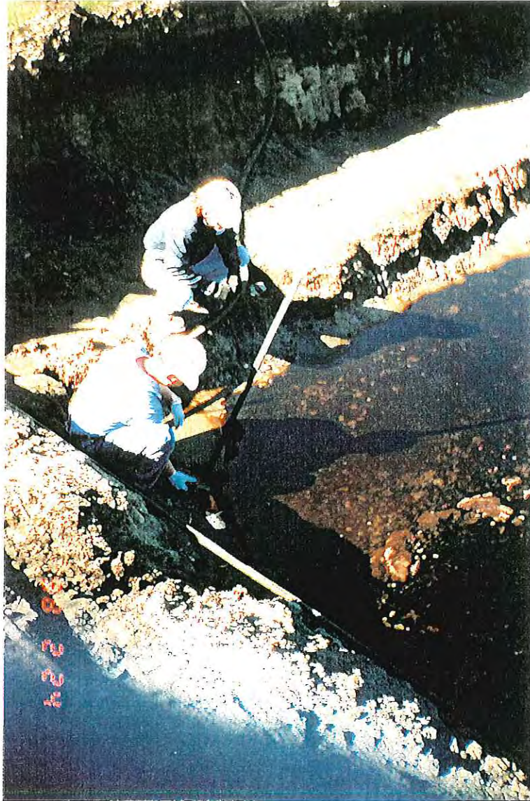
PHOTOGRAPH -82- REMOVAL OF FREE PRODUCT FROM EXCAVATION
