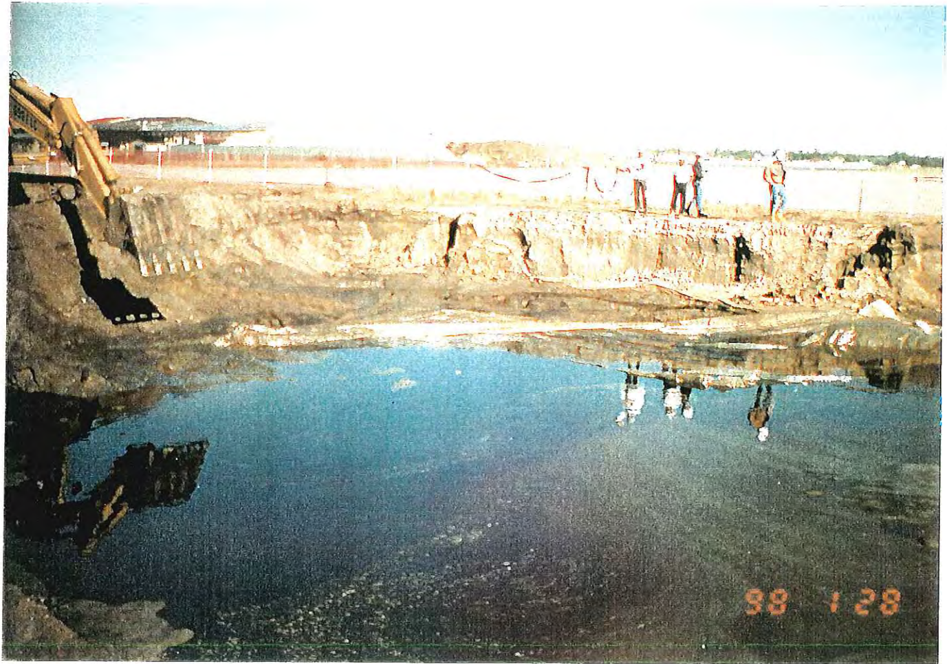
PHOTOGRAPH -69- REMOVAL OF PLASTIC LINING FROM EXCAVATION
