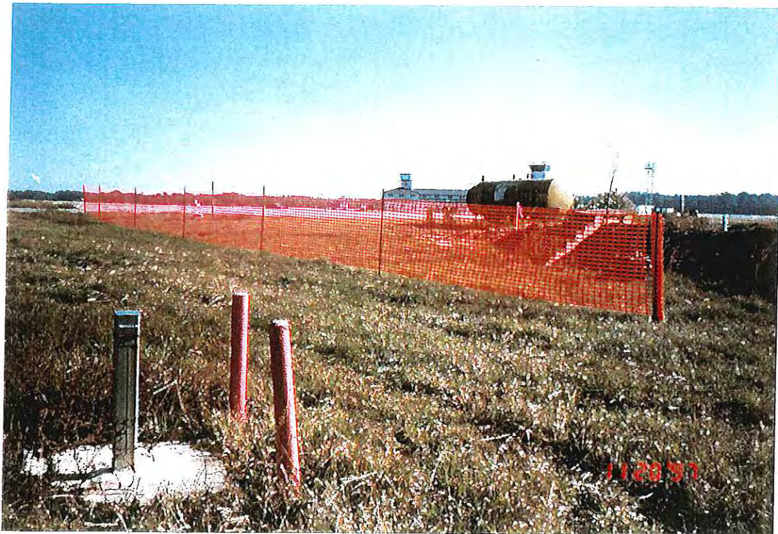
PHOTOGRAPH -21- PERIMETER FENCE INSTALLATION
