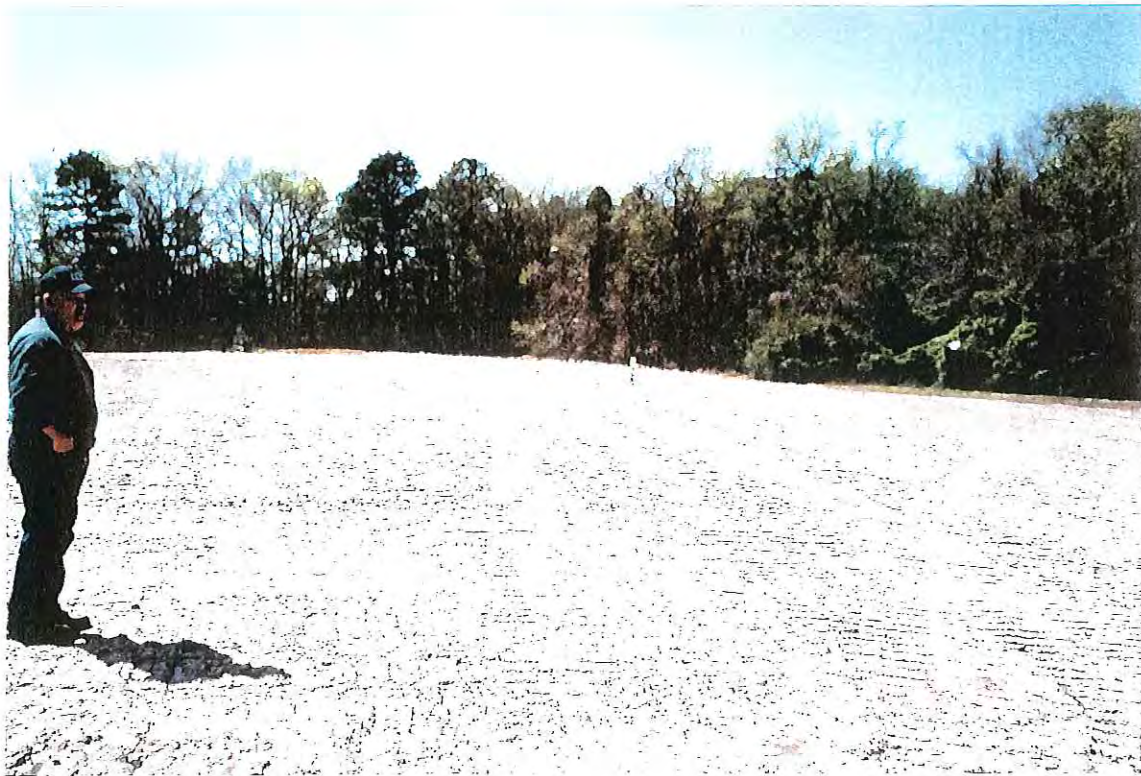
PHOTOGRAPH -93- BACKFILLED EXCAVATION
