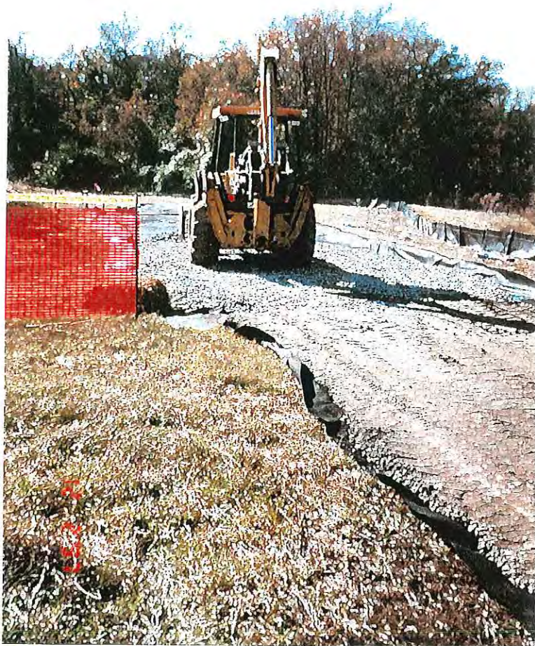
PHOTOGRAPH -34- DECON PAD CONSTRUCTION ACTIVITIES
