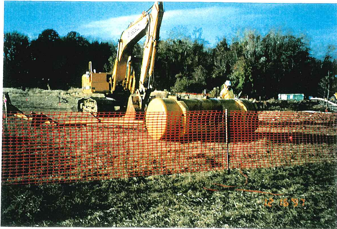
PHOTOGRAPH -43- DESTRUCTION OF 1100 GALLON ALUMINUM TANK
