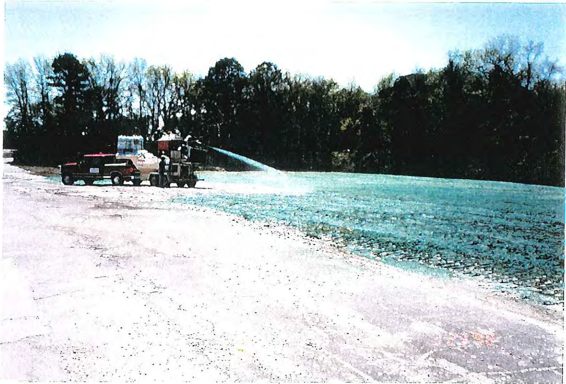
PHOTOGRAPH -95- HYDRO-SEEDING ACTIVITIES
