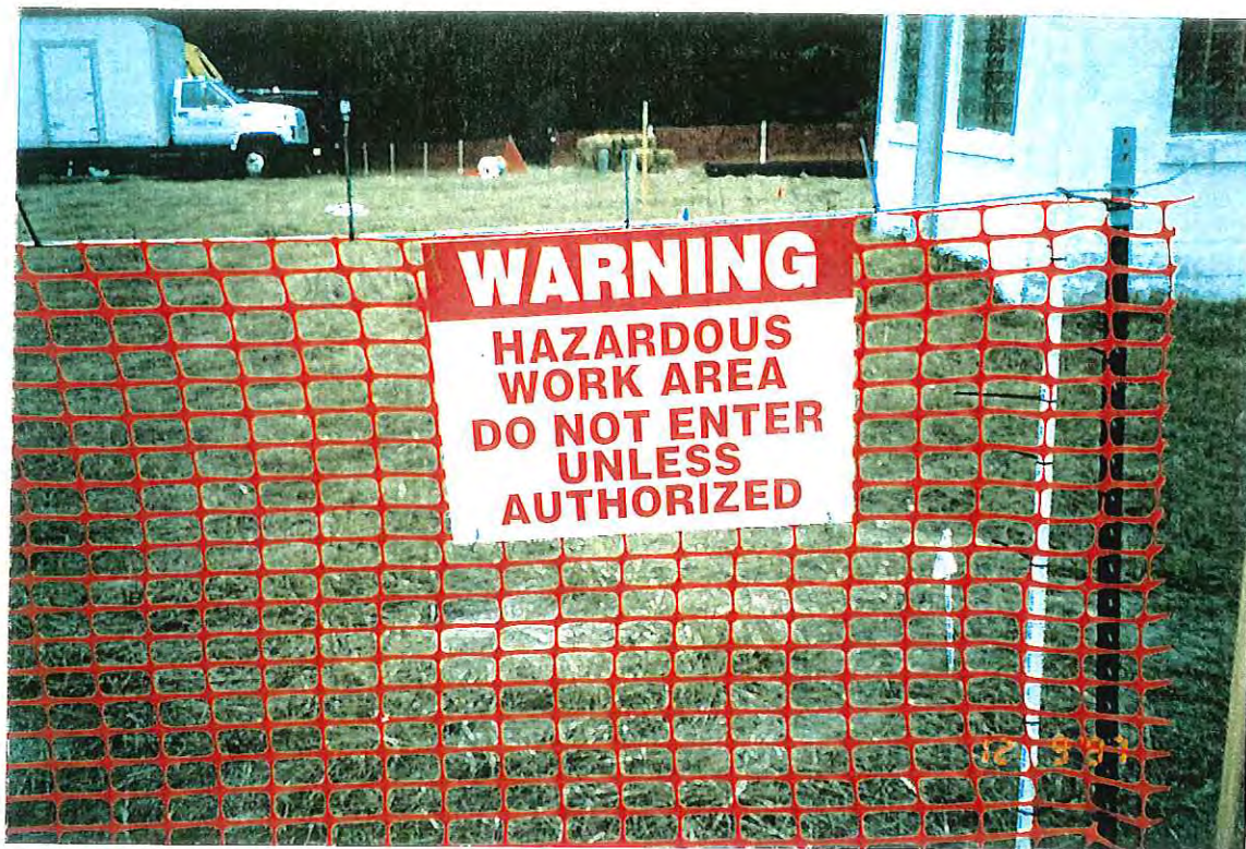
PHOTOGRAPH -39- PERIMETER FENCE SITE SIGN
