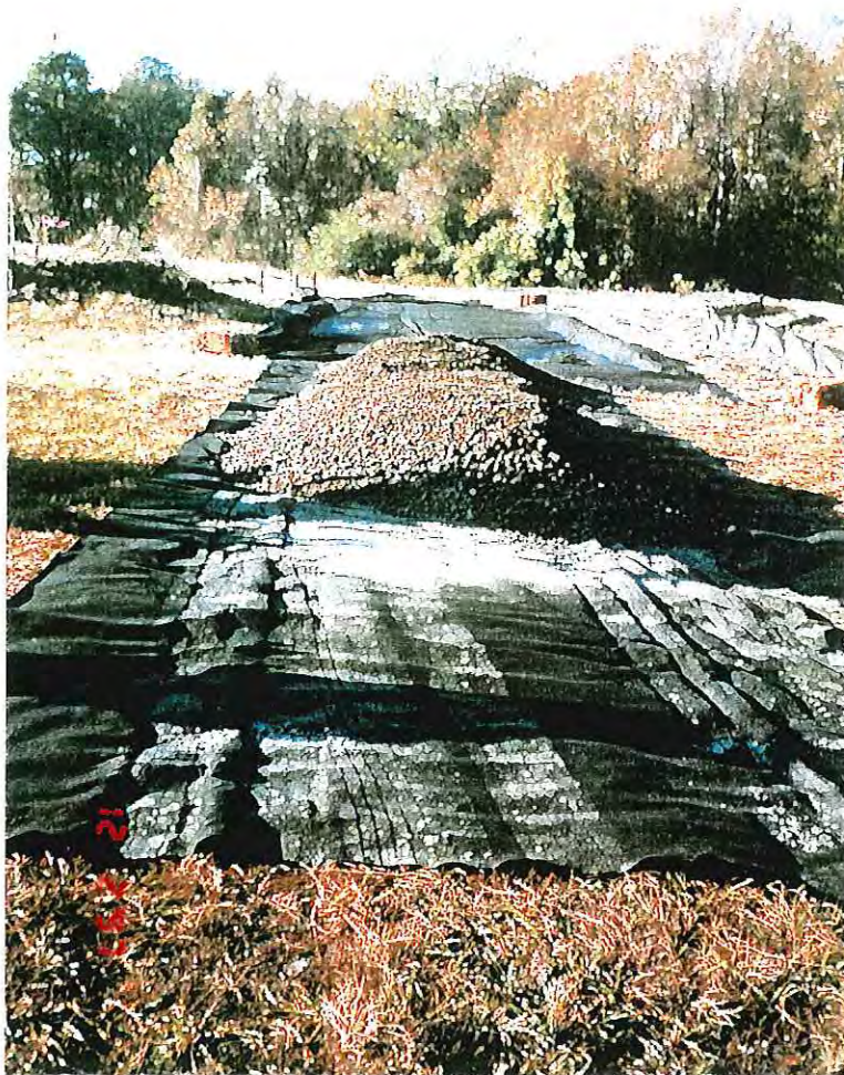
PHOTOGRAPH -32- DECON PAD CONSTRUCTION ACTIVITIES
