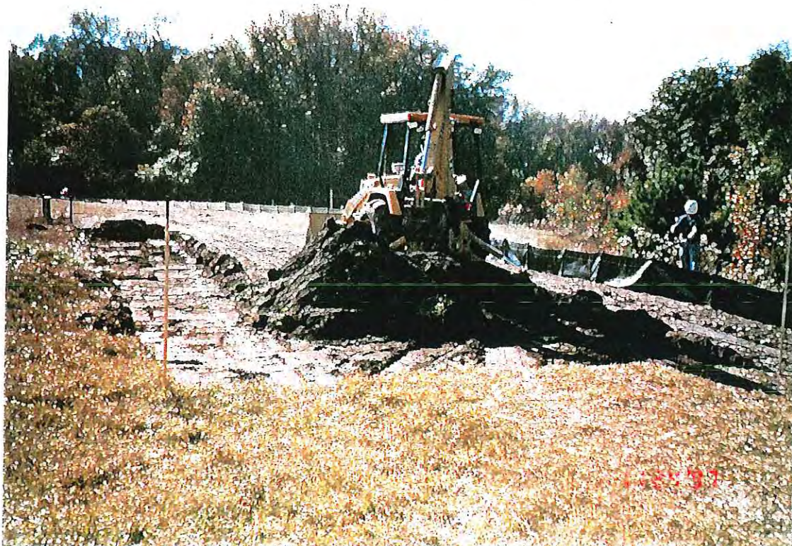
PHOTOGRAPH -27- DECON PAD BASE EARTHWORK
