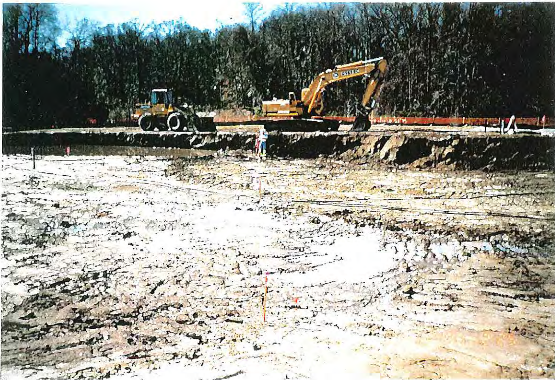
PHOTOGRAPH -84- GRID AND CONFIRMATORY SAMPLE LOCATIONS
