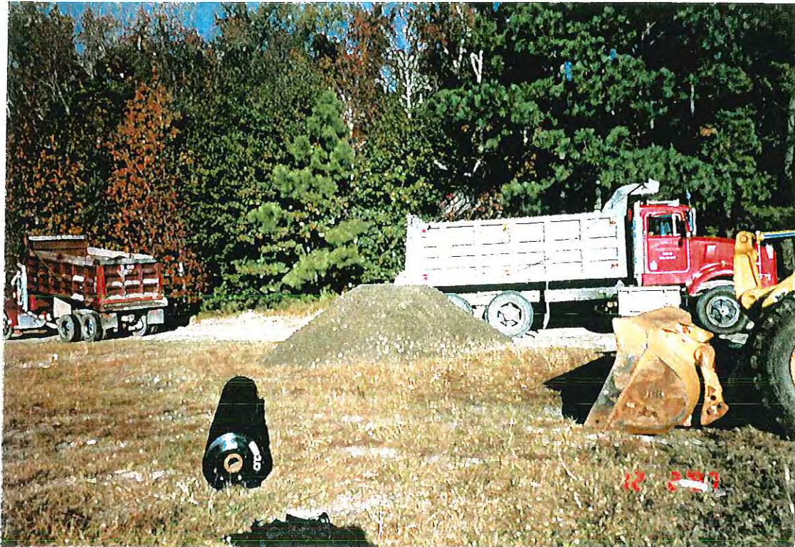
PHOTOGRAPH -31- DECON PAD CONSTRUCTION ACTIVITIES
