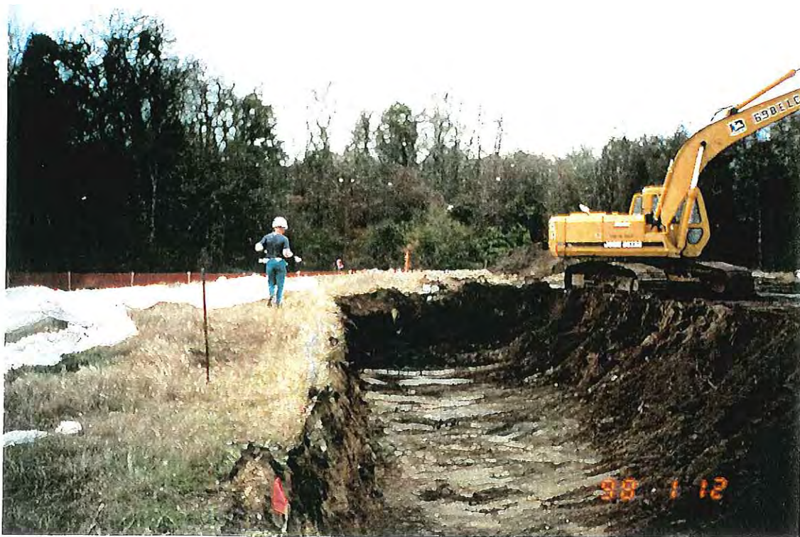
PHOTOGRAPH -53- AMBIENT AIR MONITORING DURING EXCAVATION ACTIVITIES
