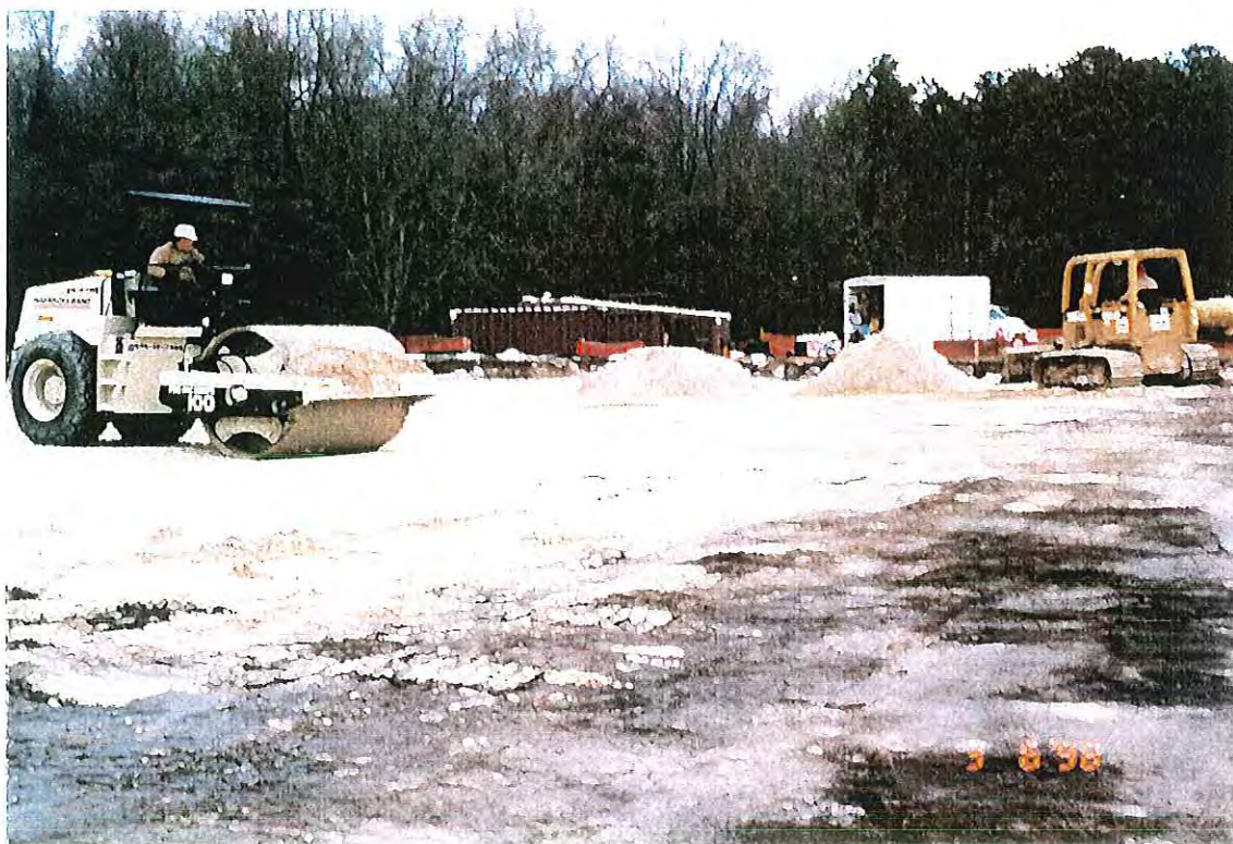
PHOTOGRAPH -92- BACKFILL ACTIVITIES
