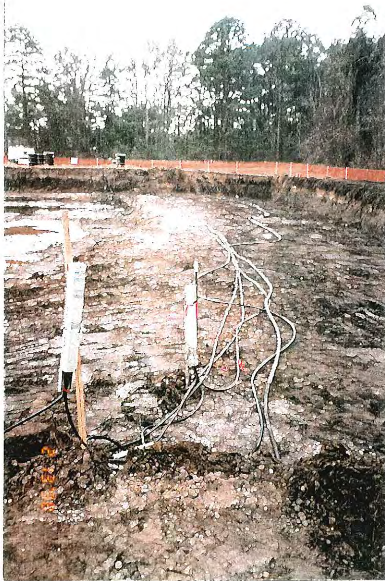
PHOTOGRAPH -73- EXPOSED UTILITIES
