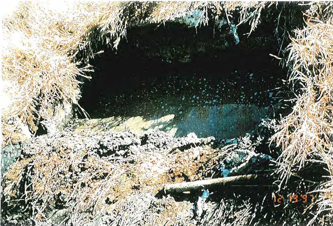
PHOTOGRAPH -51- SUMP AND VALVE REMOVAL ACTIVITIES
