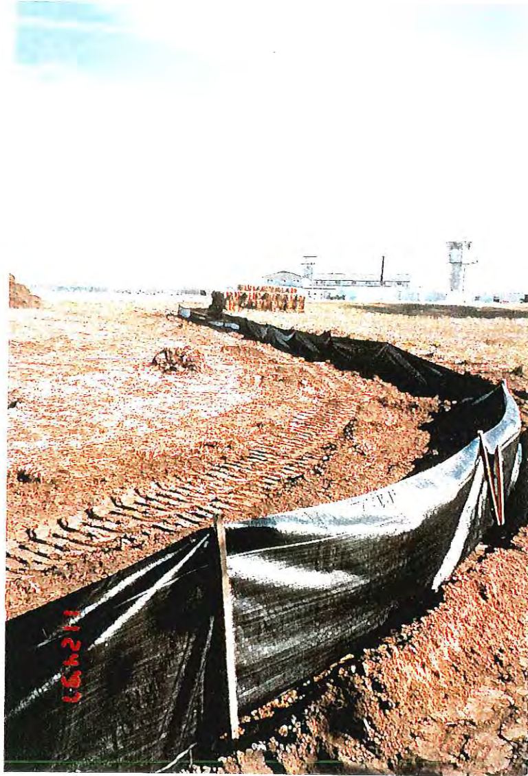
PHOTOGRAPH -22- SILT FENCE INSTALLATION
