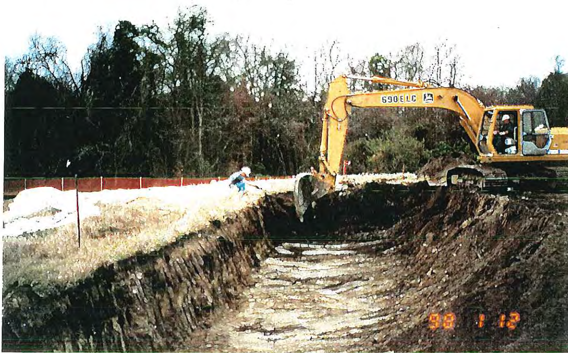
PHOTOGRAPH -54- AMBIENT AIR MONITORING DURING EXCAVATION ACTIVITIES
