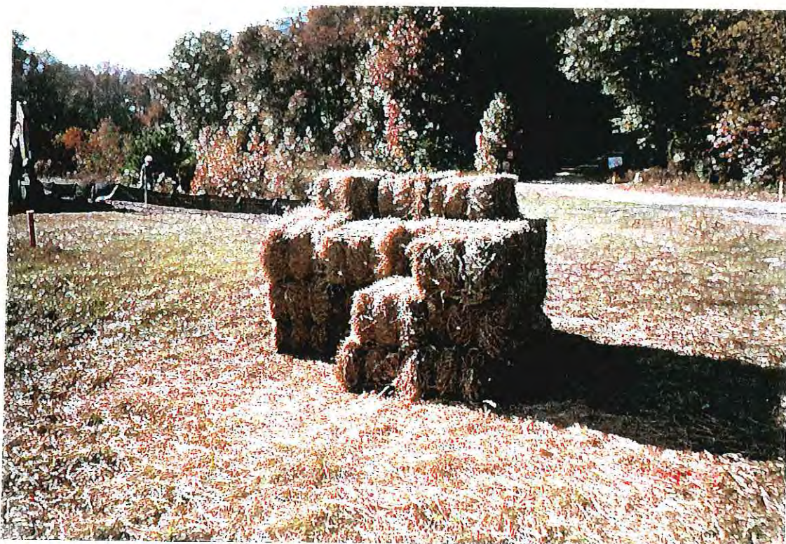
PHOTOGRAPH -23- HAY BALES TO BE PLACED ALONG OUTSIDE OF SILT FENCE
