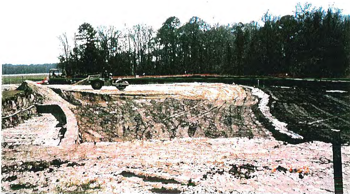
PHOTOGRAPH -88- BACKFILL ACTIVITIES
