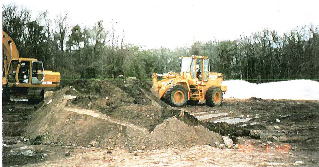
PHOTOGRAPH -56- STOCKPILING EXCAVATED SOILS
