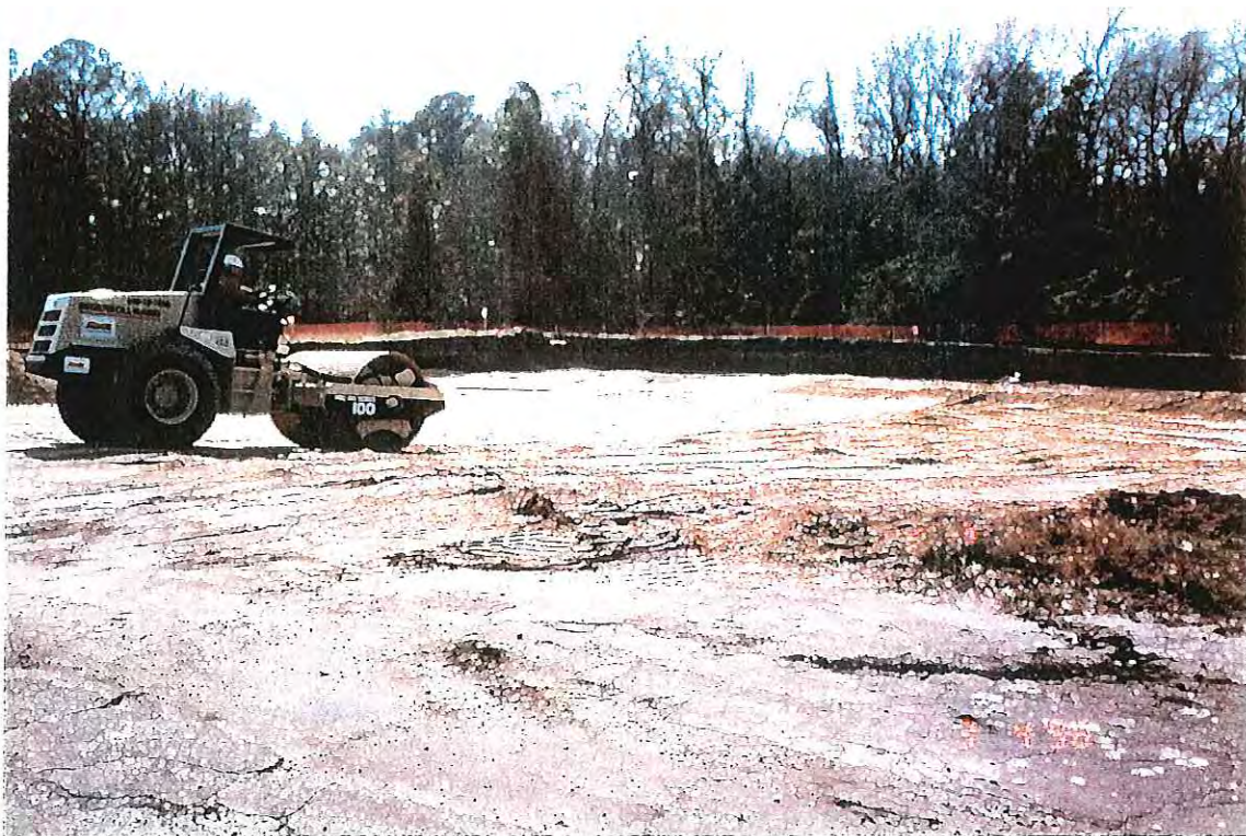
PHOTOGRAPH -89- BACKFILL ACTIVITIES
