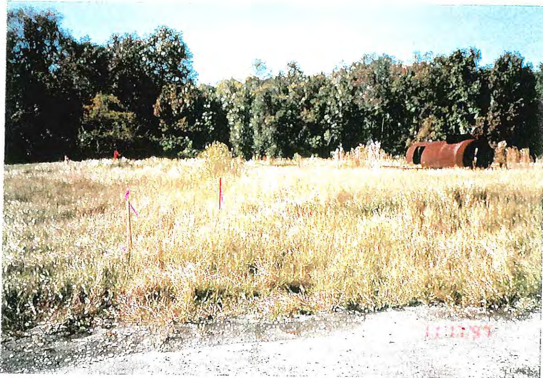
PHOTOGRAPH -7- SURVEY STAKES MARKING EXCAVATION LIMITS
