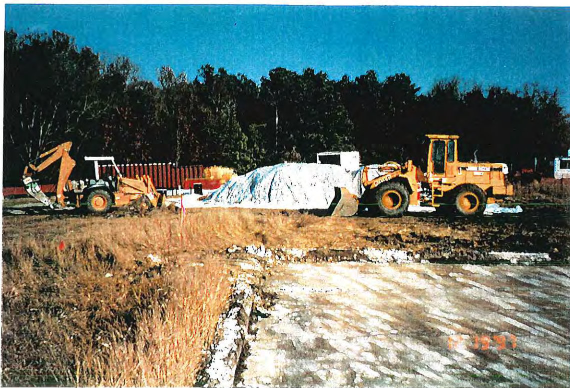
PHOTOGRAPH -50- COVERED STOCKPILED SOILS FROM CONCRETE PAD
