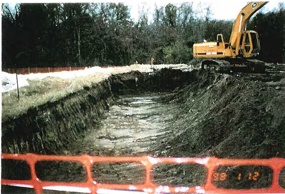
PHOTOGRAPH -55- EXCAVATION ACTIVITIES
