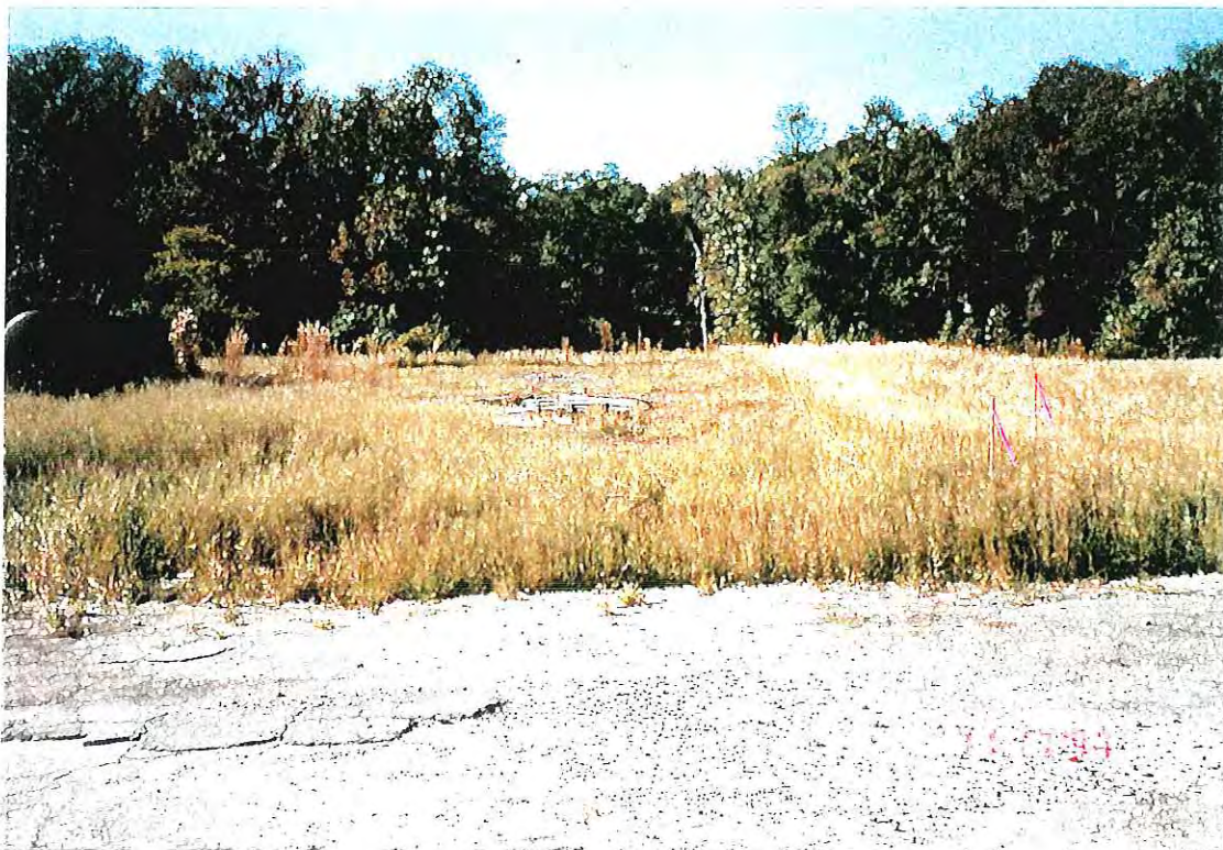
PHOTOGRAPH -8- SURVEY STAKES MARKING EXCAVATION LIMITS
