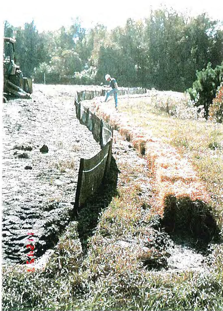
PHOTOGRAPH -24- INSTALLATION OF HAY BALES
