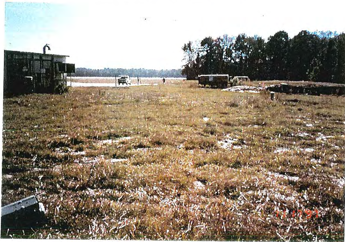
PHOTOGRAPH -6- SITE SURVEY OF EXCAVATION LIMITS
