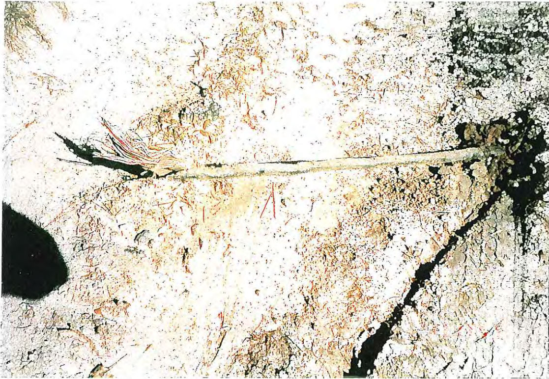
PHOTOGRAPH -9- OUT OF SERVICE UTILITY LINE ALONG DIRT ROAD NORTH OF THE SITE
