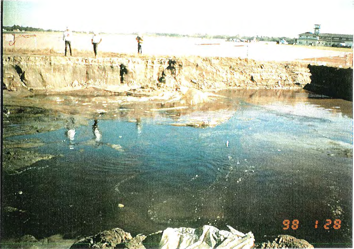
PHOTOGRAPH -68- FREE PRODUCT IN EXCAVATION
