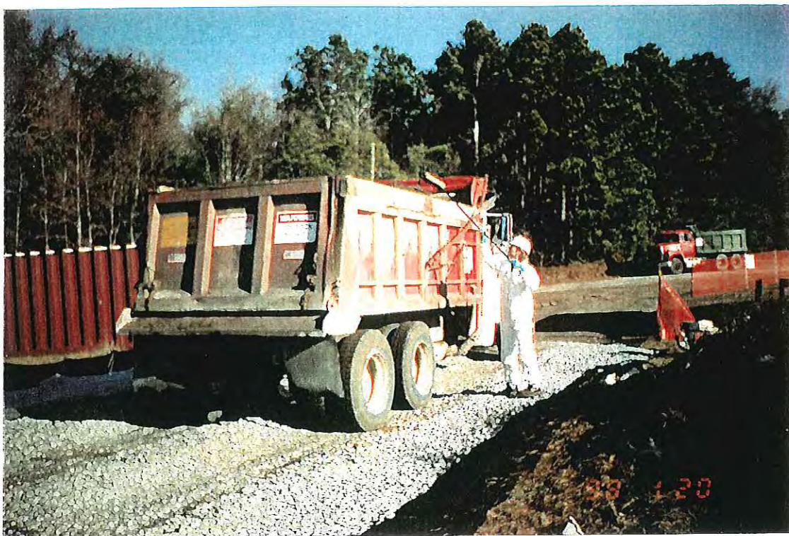
PHOTOGRAPH -59- CLEANING TRUCKS ON DECON PAD PRIOR TO LEAVING SITE
