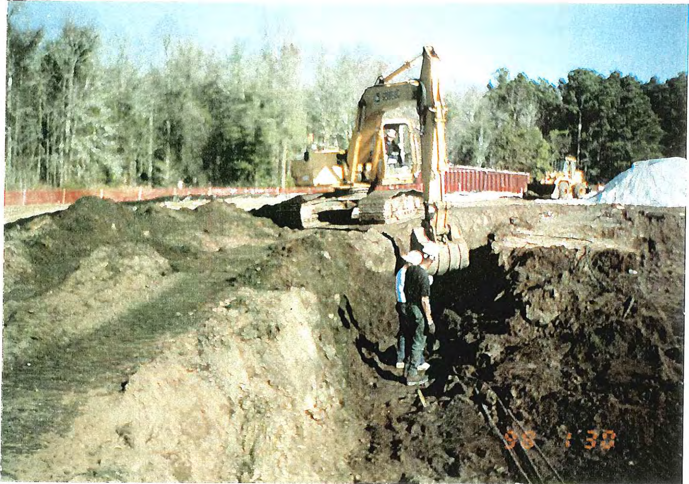
PHOTOGRAPH -70- EXCAVATION ACTIVITIES (EXPOSING UTILITIES)
