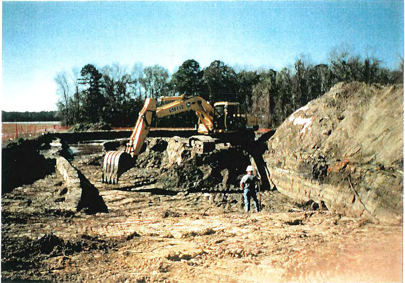
PHOTOGRAPH -77- EXCAVATION ACTIVITIES
