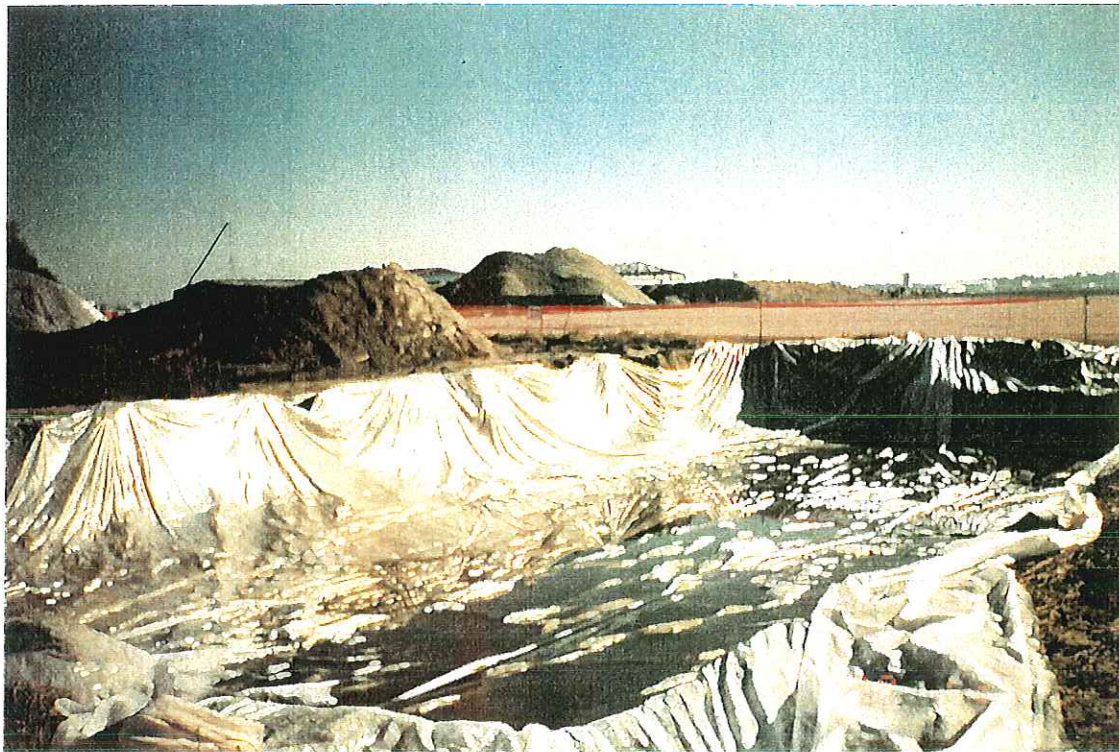
PHOTOGRAPH -66- LINING OF EXCAVATION
