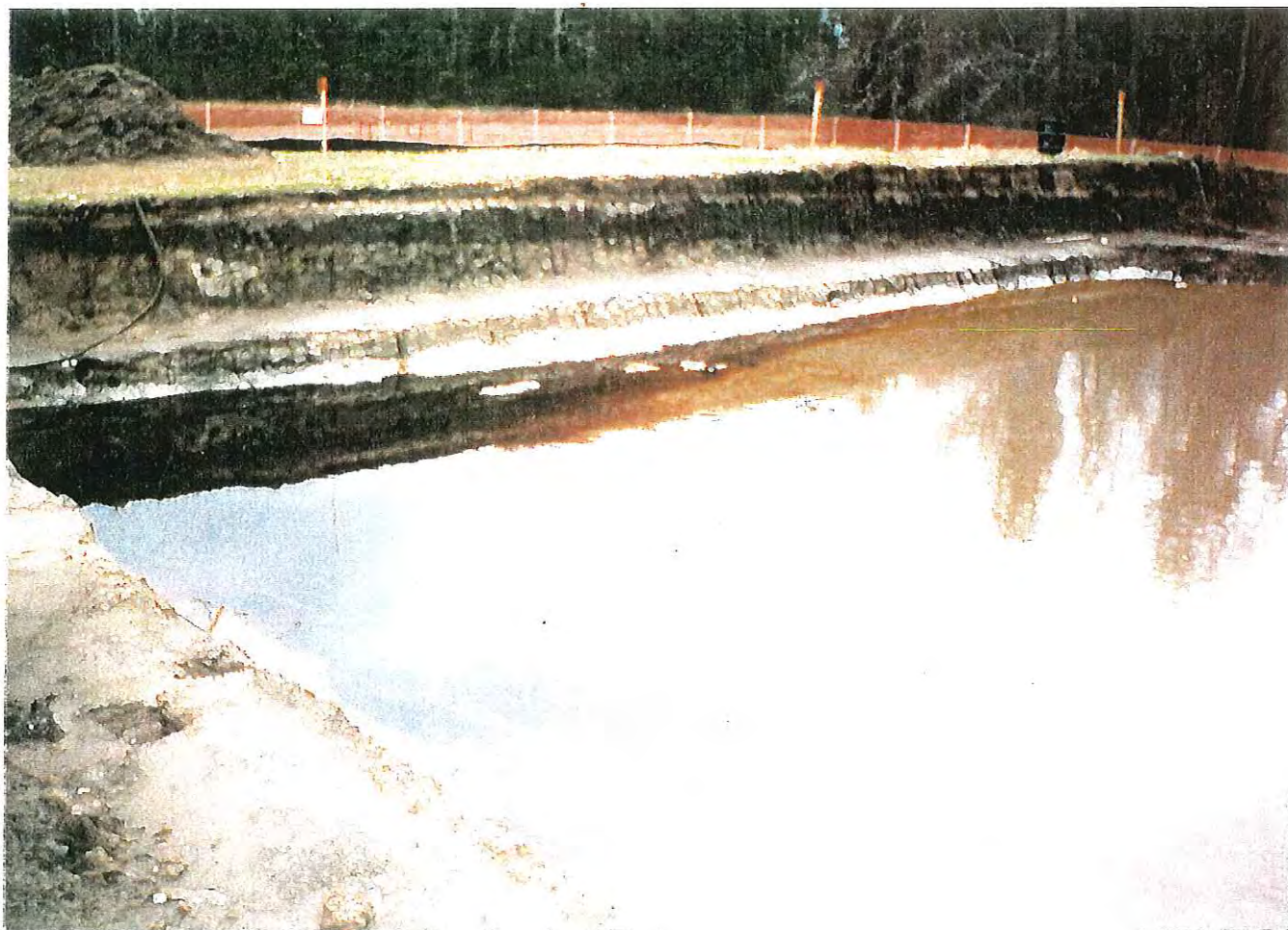
PHOTOGRAPH -80- FREE PRODUCT IN EXCAVATION
