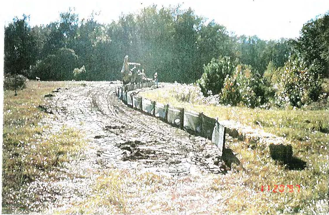
PHOTOGRAPH -18- SILT FENCE INSTALLATION
