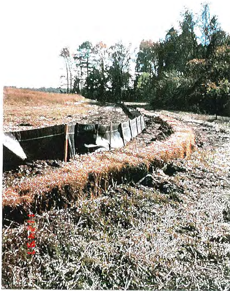
PHOTOGRAPH -25- INSTALLATION OF HAY BALES
