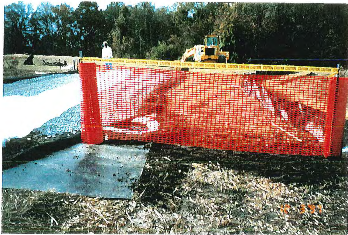
PHOTOGRAPH -36- COMPLETED DECON PAD
