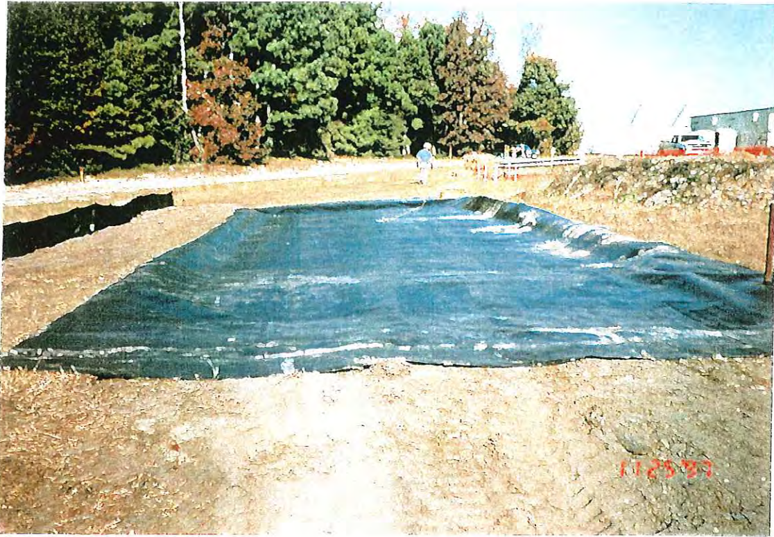
PHOTOGRAPH -30- DECON PAD CONSTRUCTION ACTIVITIES
