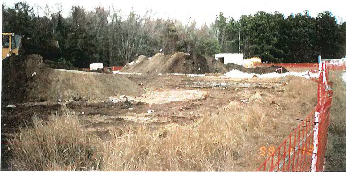
PHOTOGRAPH -57- STOCKPILED EXCAVATED SOILS
