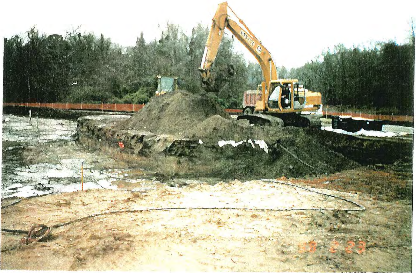
PHOTOGRAPH -81- EXCAVATION ACTIVITIES
