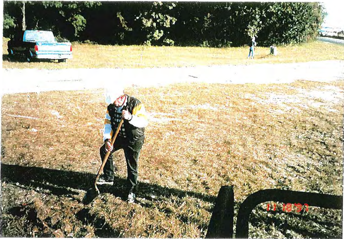
PHOTOGRAPH -17- HAND DIGGING LOCATING UTILITY LINES
