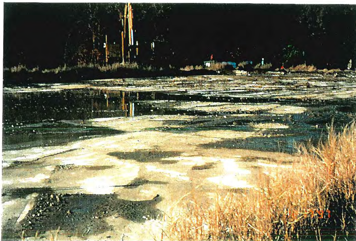
PHOTOGRAPH -48- CONCRETE PAD AFTER SOIL REMOVAL
