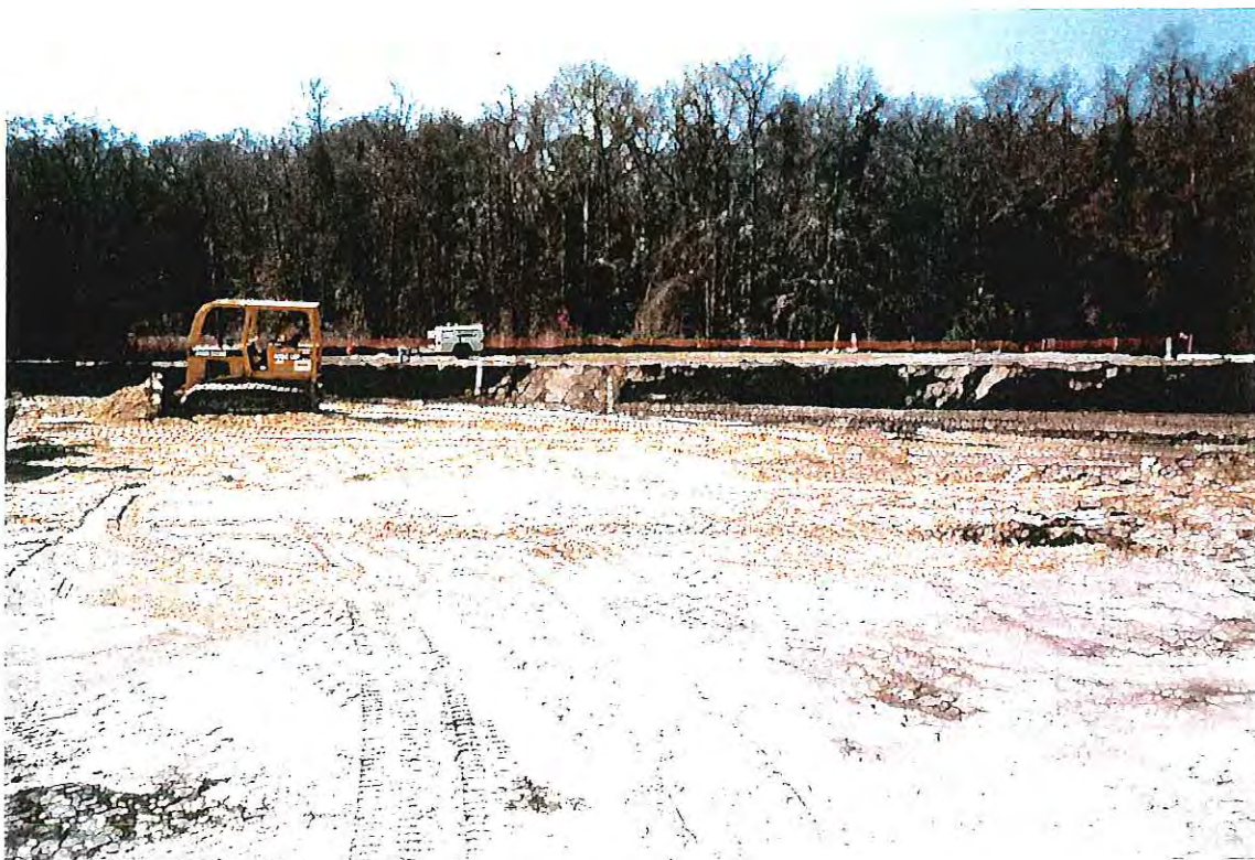
PHOTOGRAPH -90- BACKFILL ACTIVITIES
