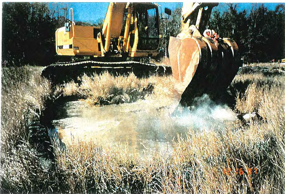
PHOTOGRAPH -47- SOIL REMOVAL FROM CONCRETE PAD
