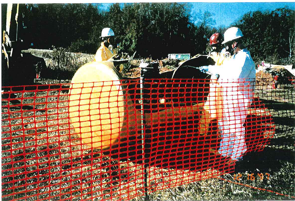
PHOTOGRAPH -46- ALUMINUM TANK CLEANING AND AIR MONITORING
