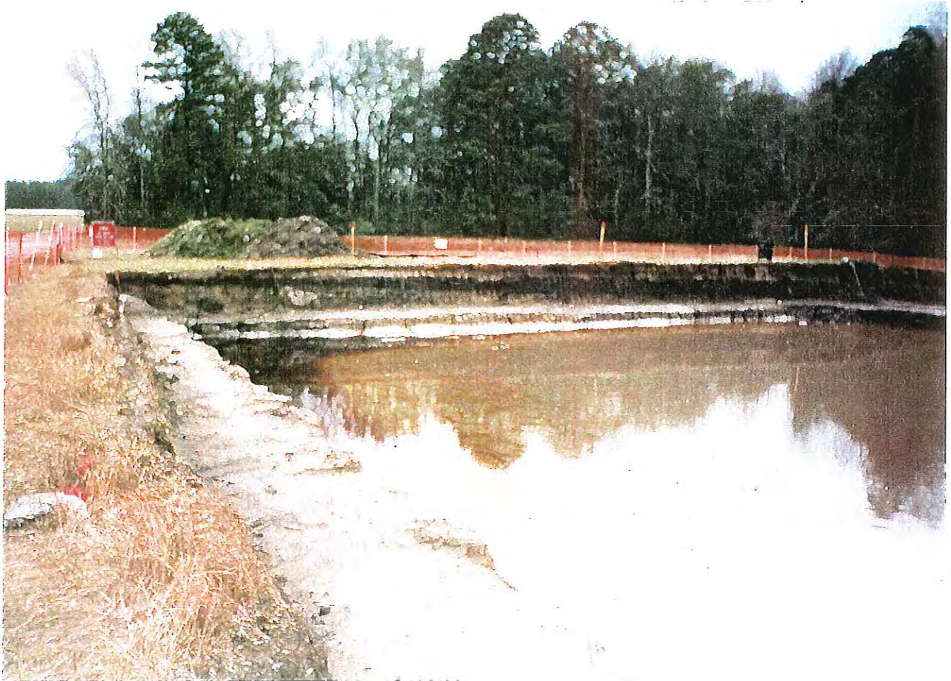
PHOTOGRAPH -79- FREE PRODUCT IN EXCAVATION
