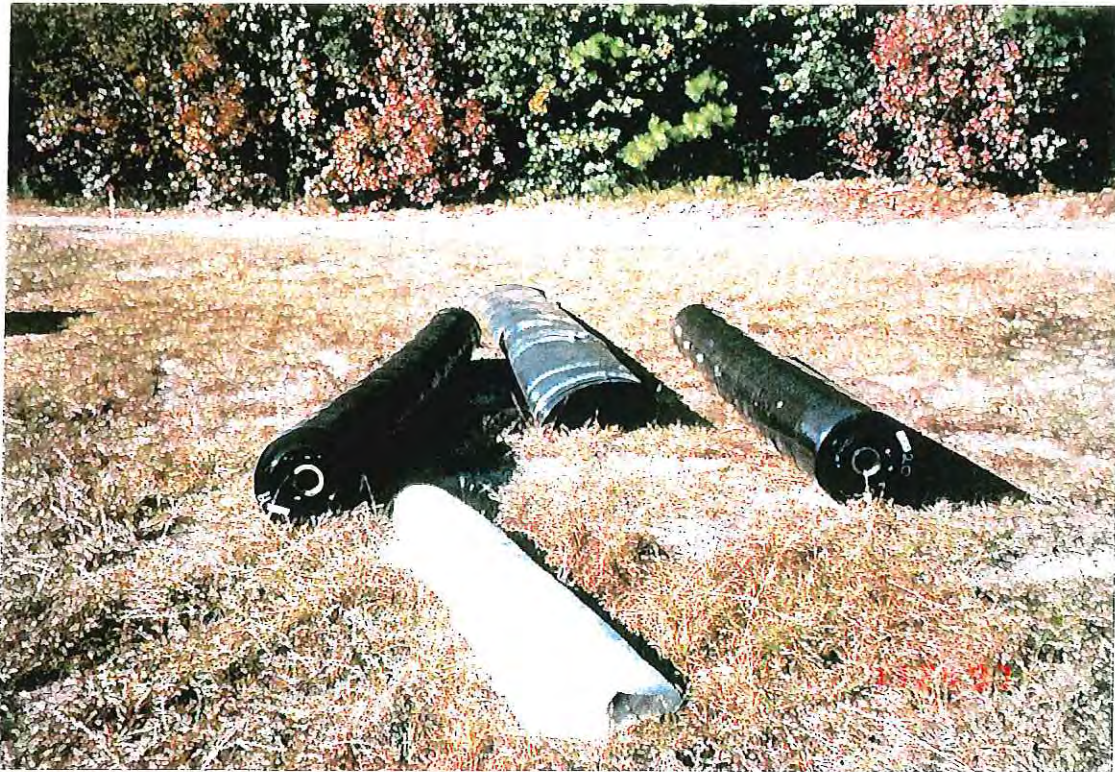
PHOTOGRAPH -26- DECON PAD PLASTIC SHEETING
