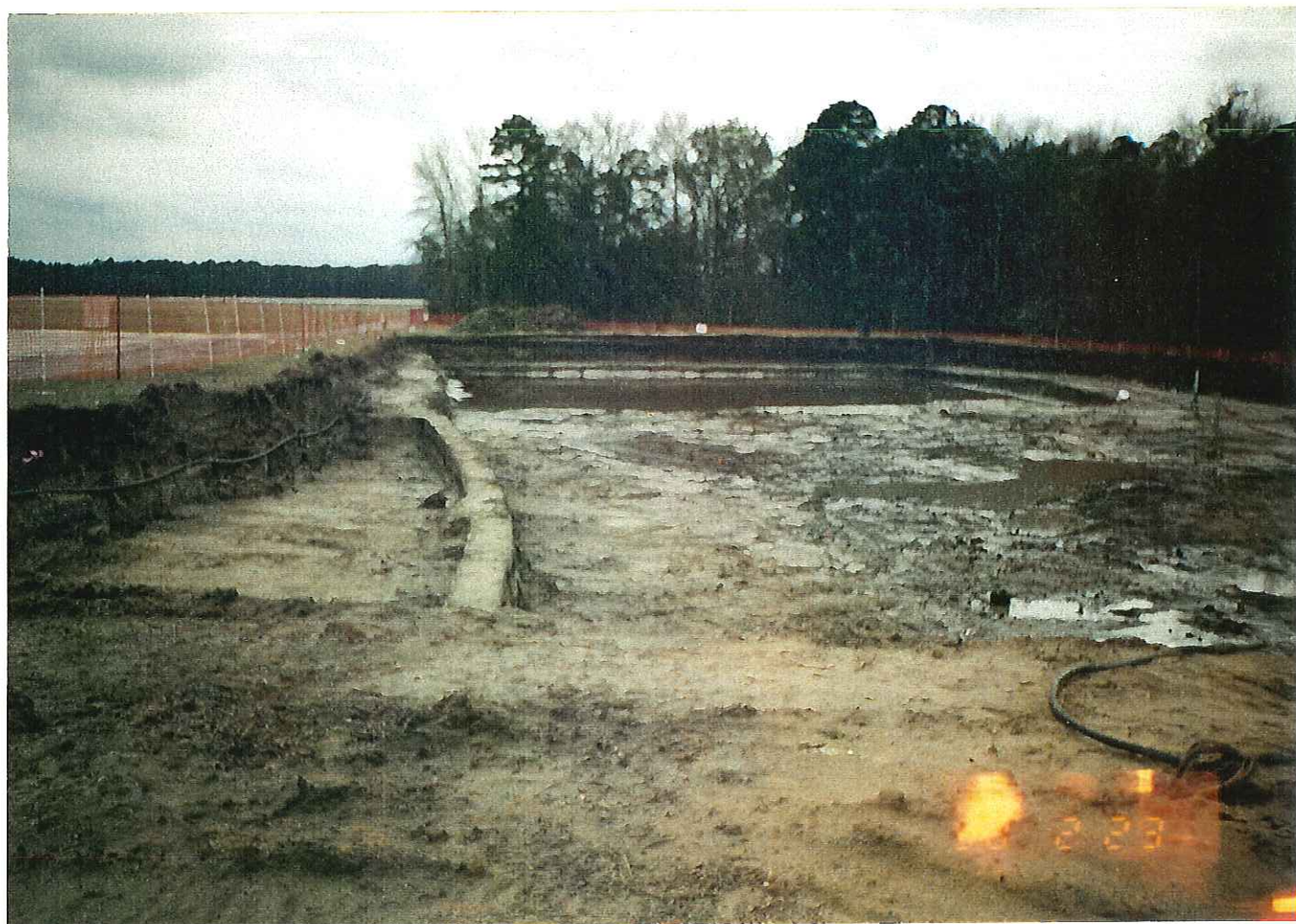
PHOTOGRAPH -78- EXCAVATION SITE
