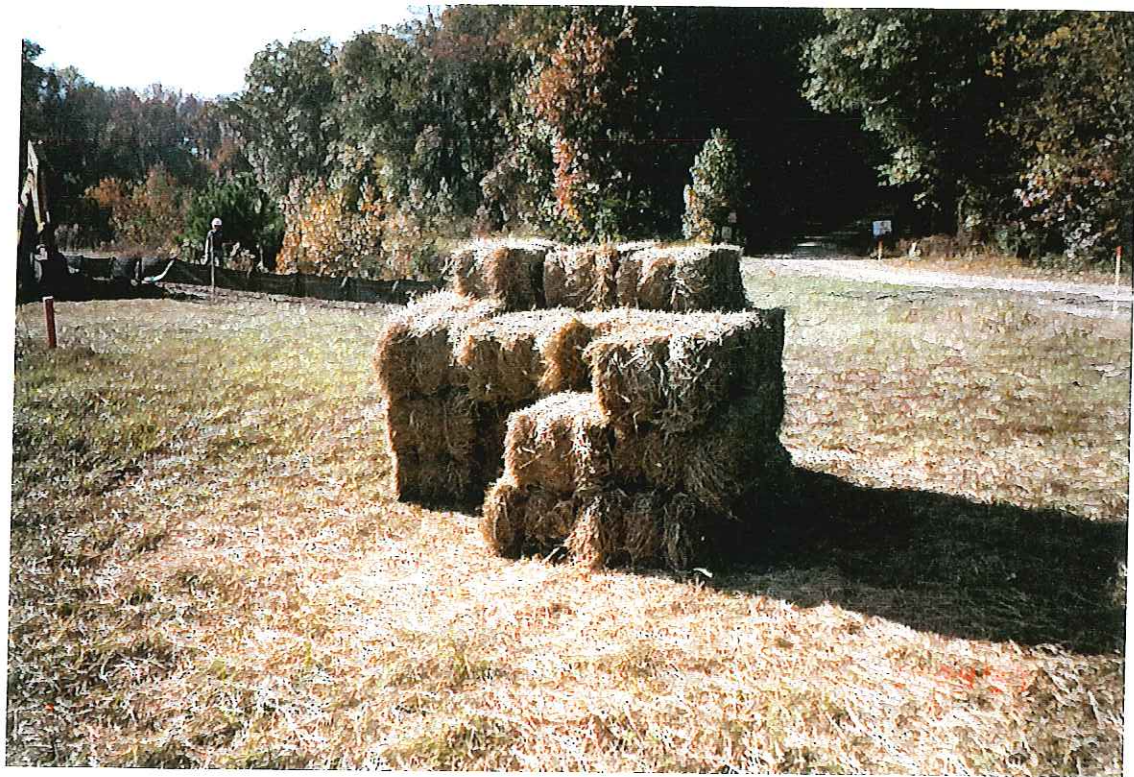
PHOTOGRAPH -23- HAY BALES TO BE PLACED ALONG OUTSIDE OF SILT FENCE
