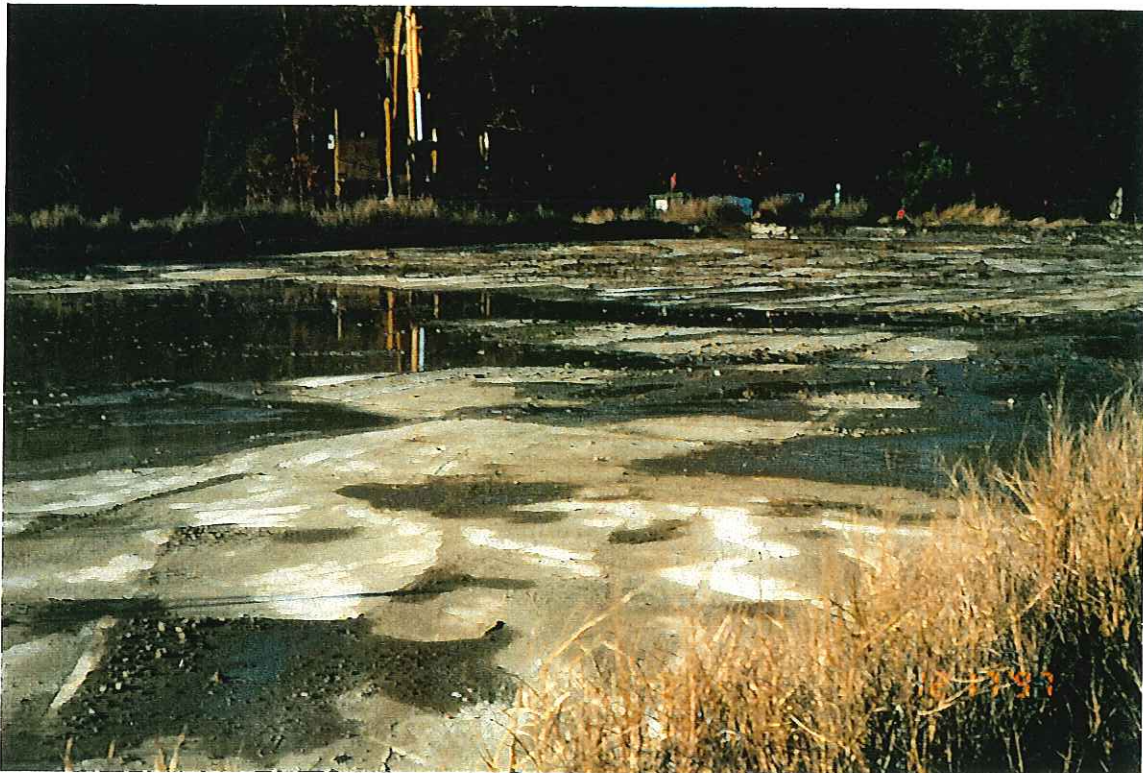
PHOTOGRAPH -48- CONCRETE PAD AFTER SOIL REMOVAL
