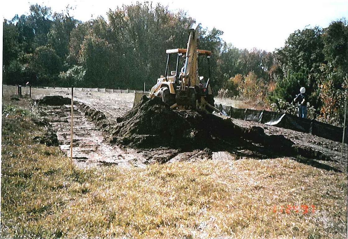
PHOTOGRAPH -27- DECON PAD BASE EARTHWORK
