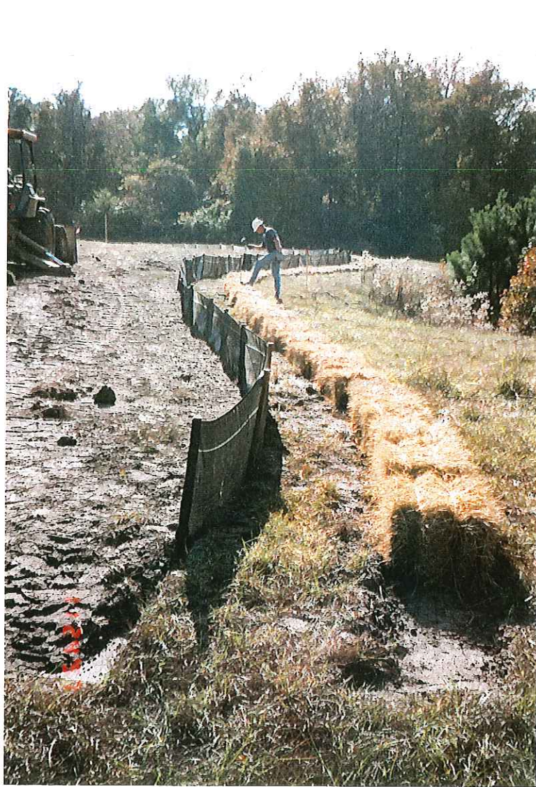
PHOTOGRAPH -24- INSTALLATION OF HAY BALES
