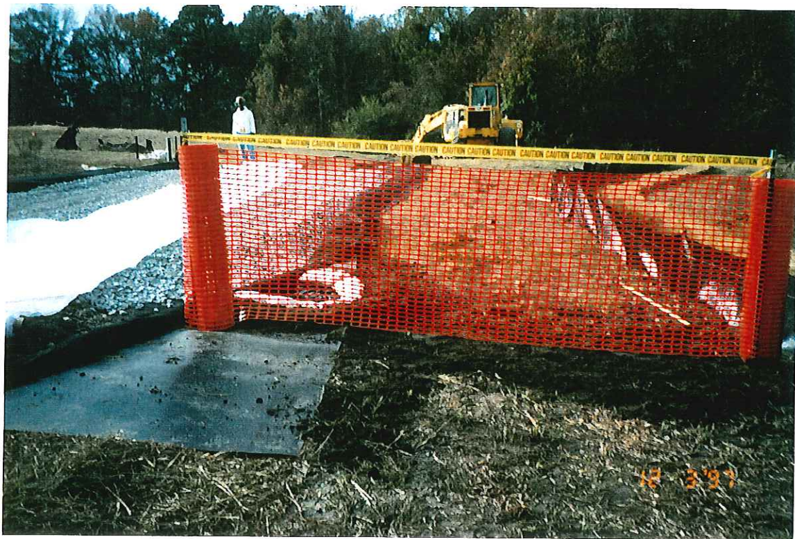
PHOTOGRAPH -36- COMPLETED DECON PAD
