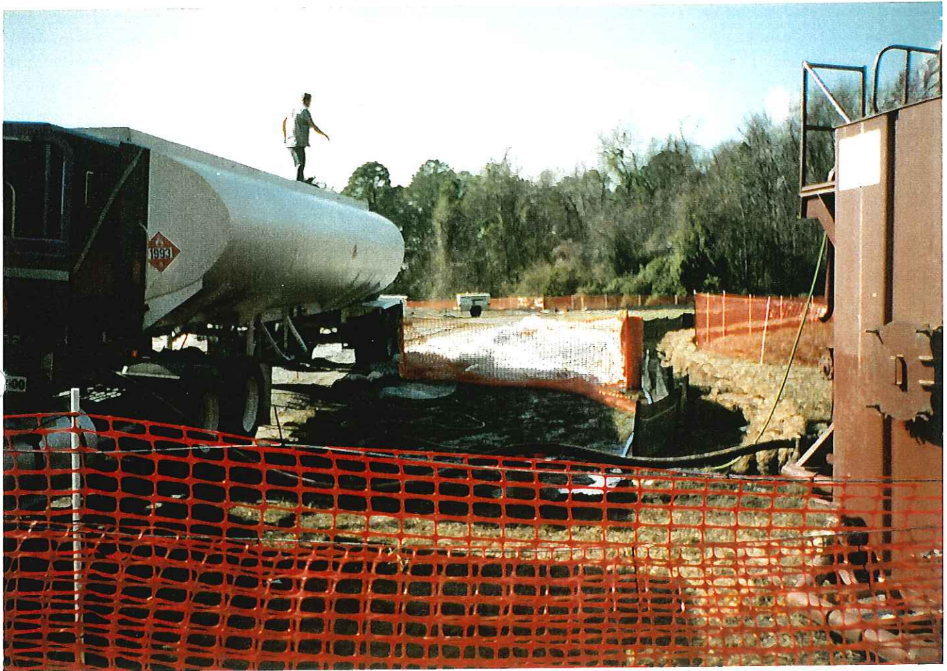
PHOTOGRAPH -76- REMOVAL OF GENERATED WASTEWATER
