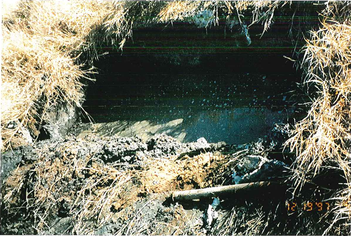
PHOTOGRAPH -51- SUMP AND VALVE REMOVAL ACTIVITIES
