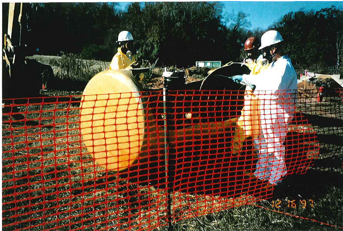
PHOTOGRAPH -46- ALUMINUM TANK CLEANING AND AIR MONITORING
