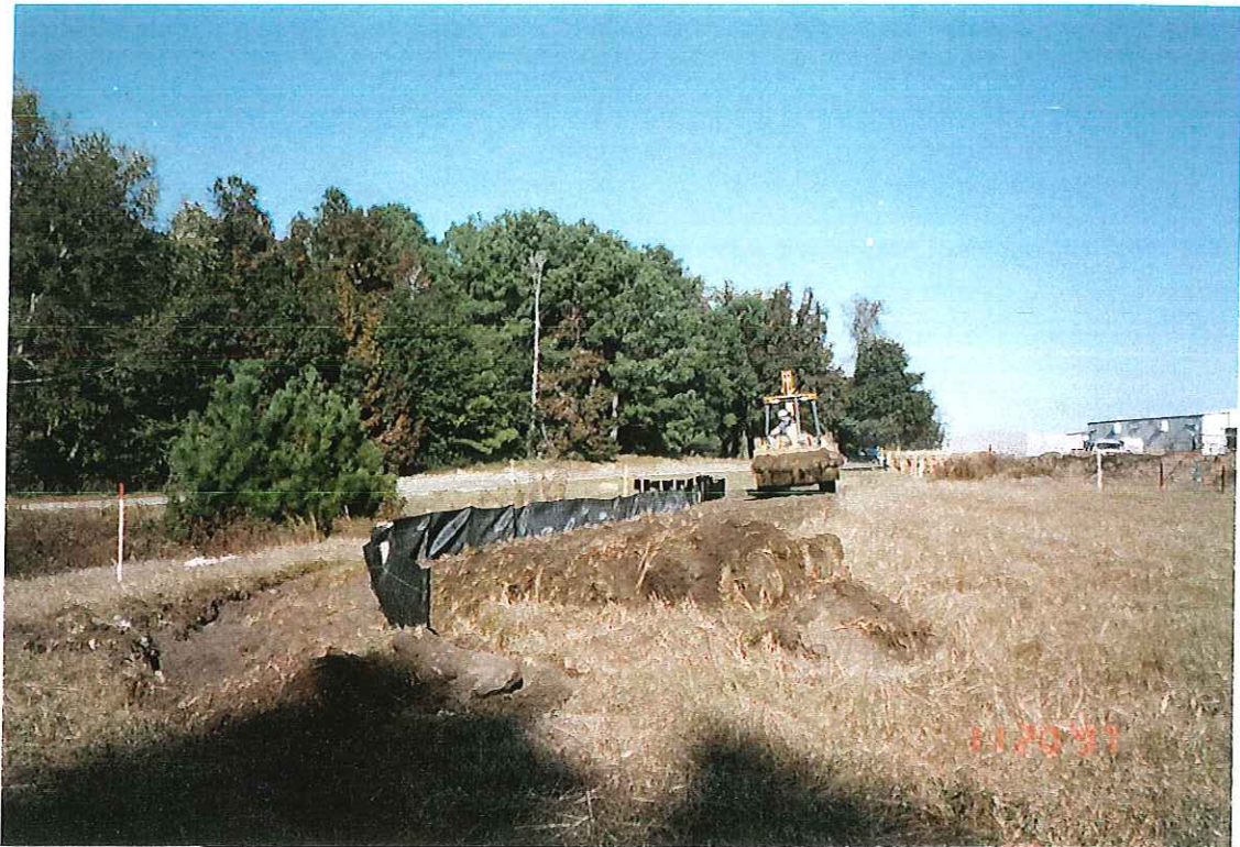
PHOTOGRAPH -19- SILT FENCE INSTALLATION
