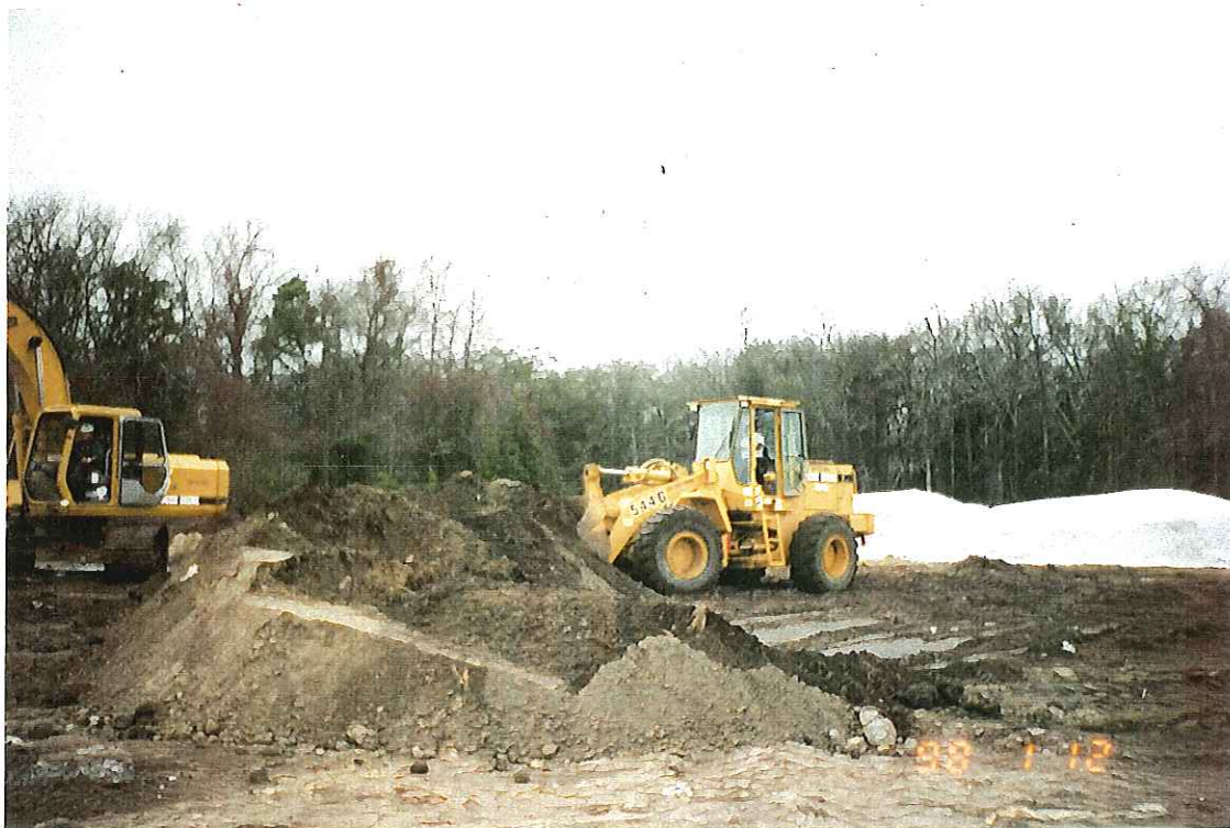
PHOTOGRAPH -56- STOCKPILING EXCAVATED SOILS
