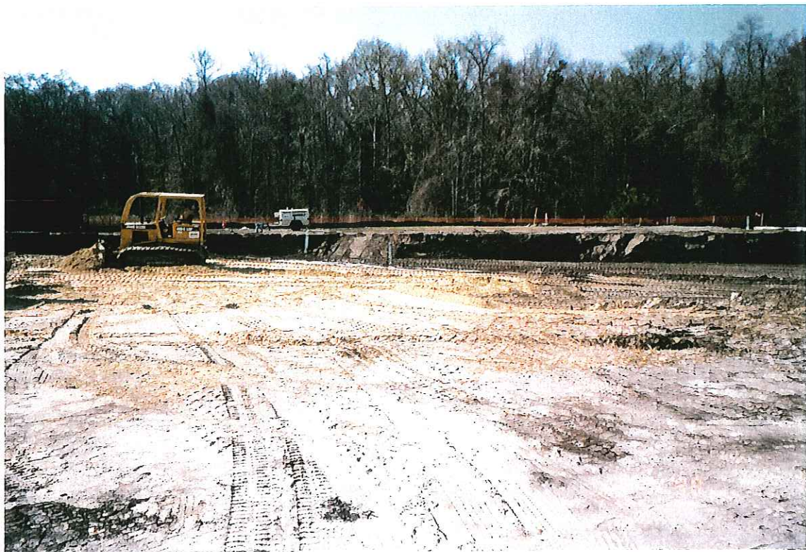
PHOTOGRAPH -90- BACKFILL ACTIVITIES
