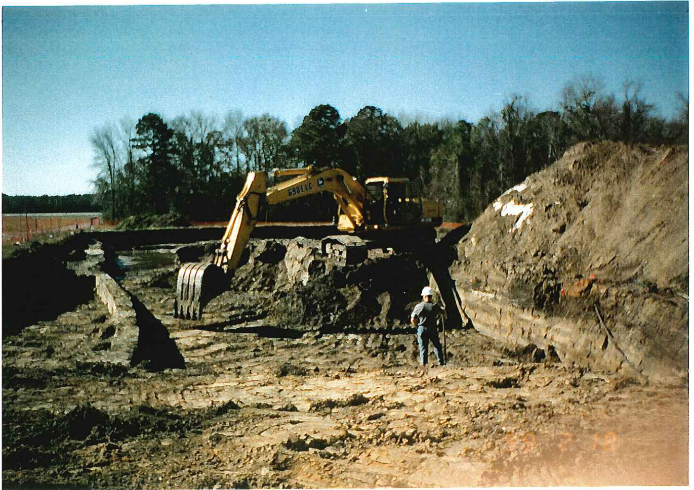
PHOTOGRAPH -77- EXCAVATION ACTIVITIES
