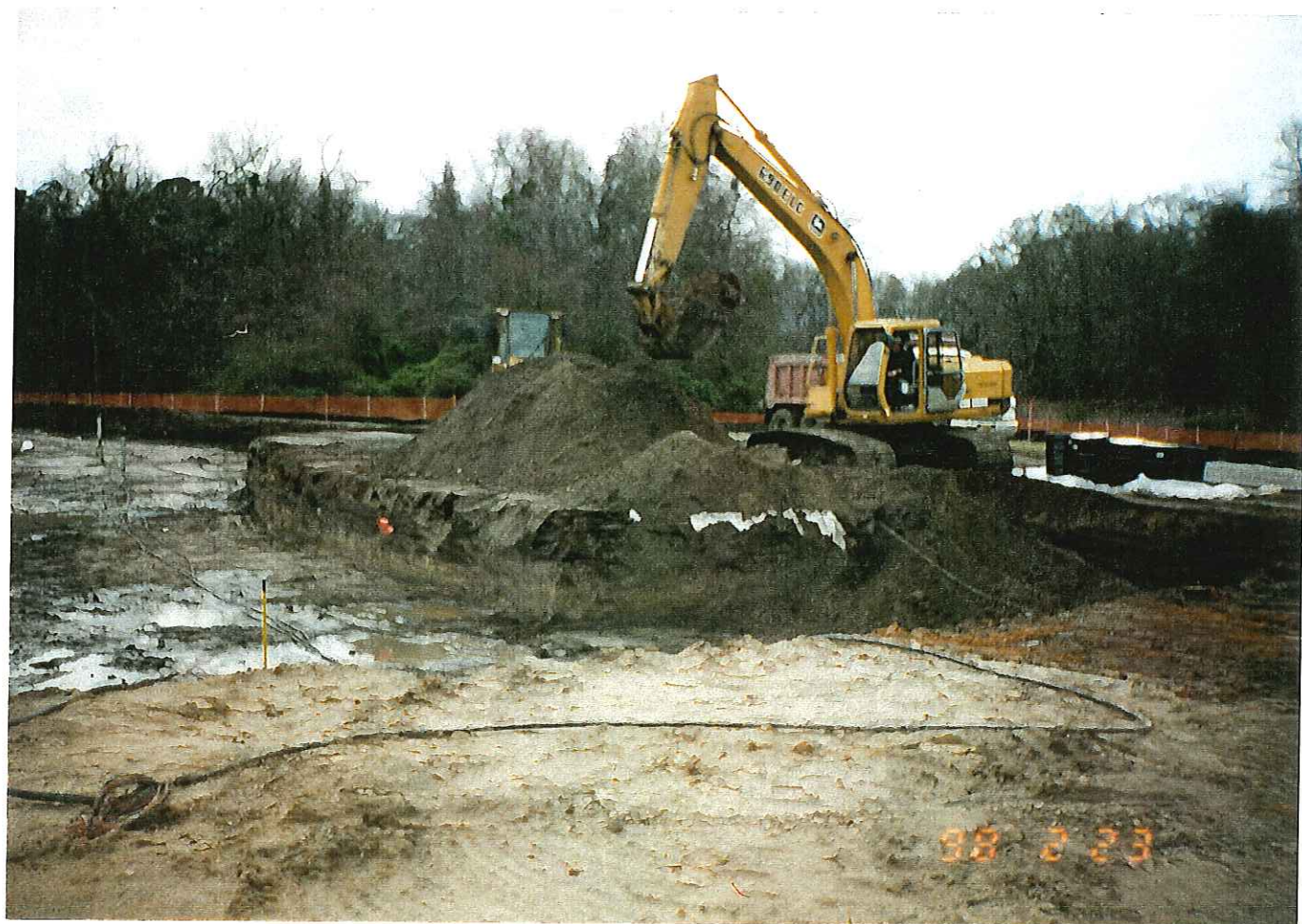
PHOTOGRAPH -81- EXCAVATION ACTIVITIES
