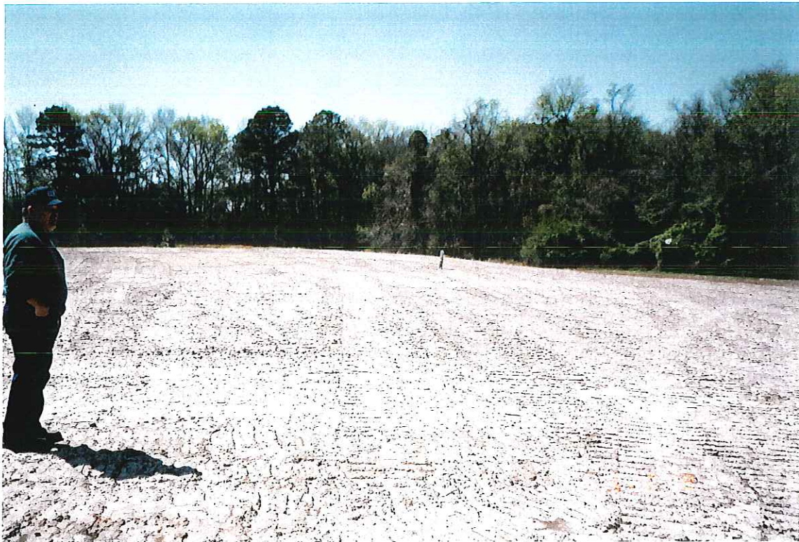
PHOTOGRAPH -93- BACKFILLED EXCAVATION
