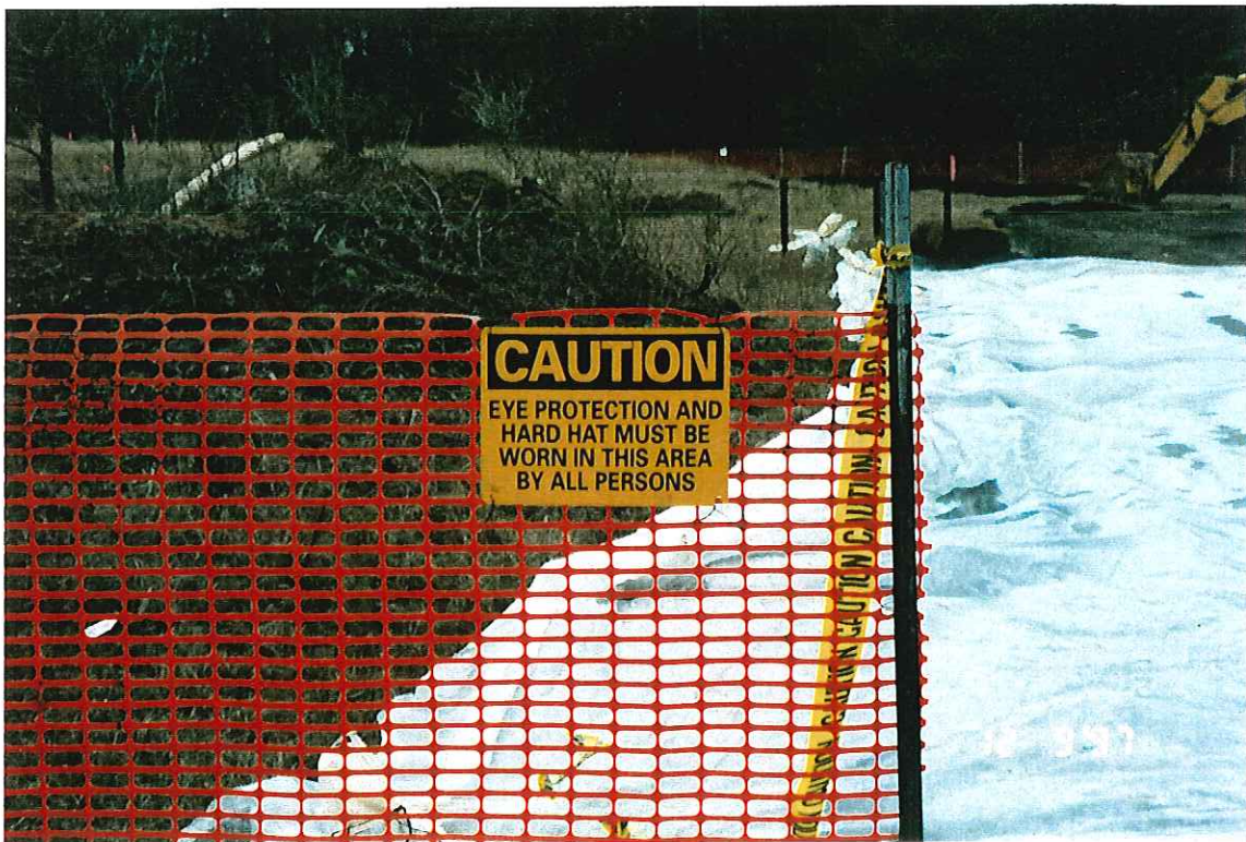
PHOTOGRAPH -38- PERIMETER FENCE SITE SIGN
