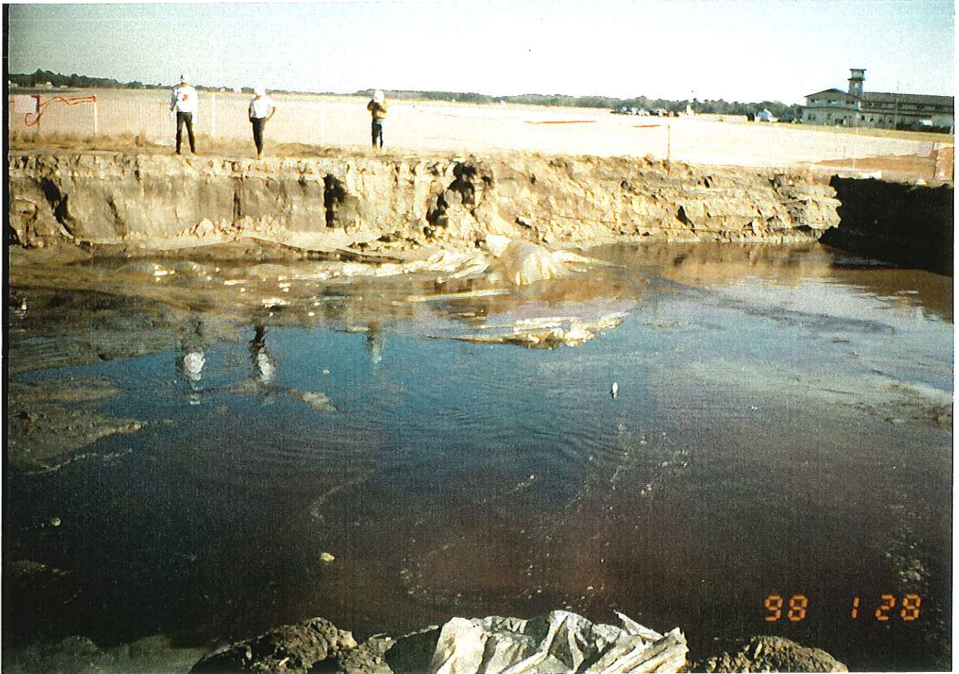
PHOTOGRAPH -68- FREE PRODUCT IN EXCAVATION
