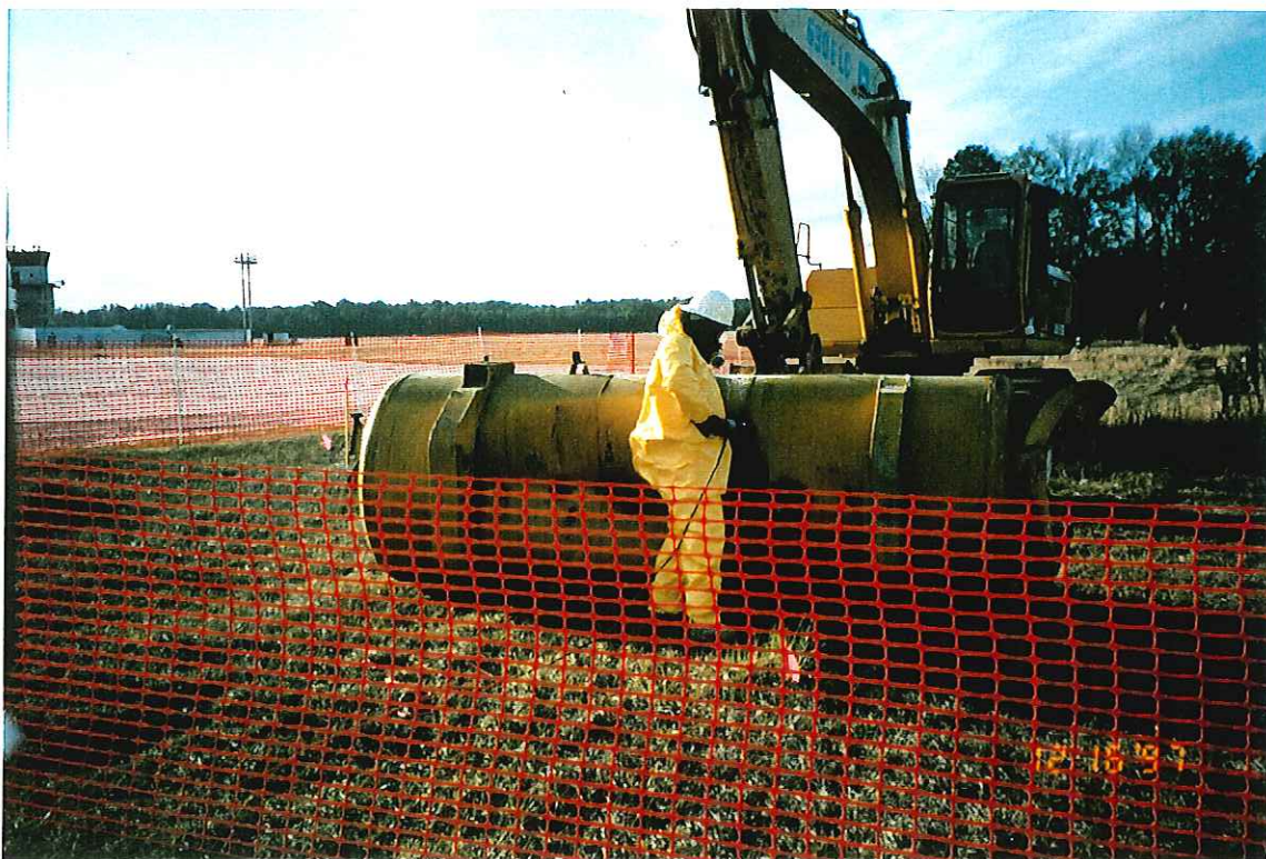
PHOTOGRAPH -44- DESTRUCTION OF 1100 GALLON ALUMINUM TANK
