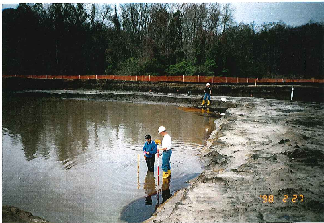
PHOTOGRAPH -86- SURVEY OF GRID AND CONFIRMATORY SAMPLE LOCATIONS
