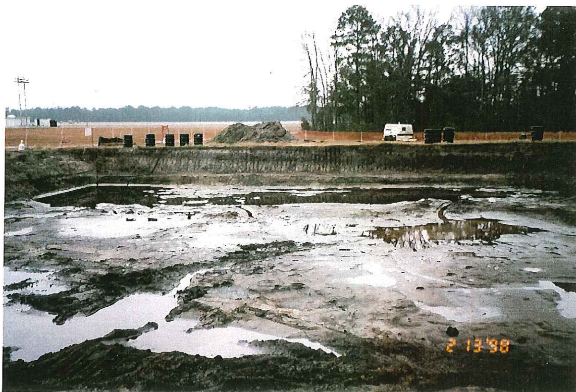
PHOTOGRAPH -72- EXCAVATION AFTER WATER AND PRODUCT REMOVAL ACTIVITIES
