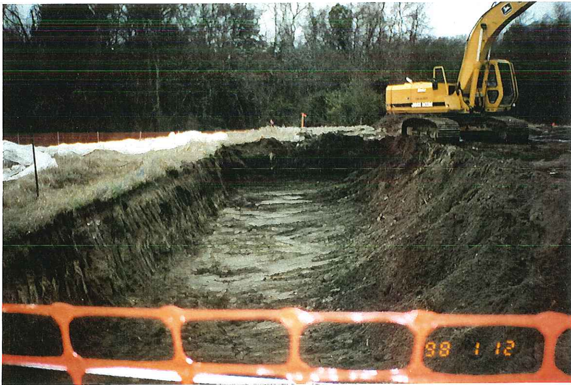
PHOTOGRAPH -55- EXCAVATION ACTIVITIES
