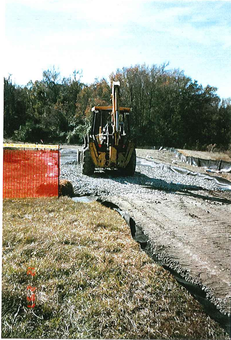
PHOTOGRAPH -34- DECON PAD CONSTRUCTION ACTIVITIES
