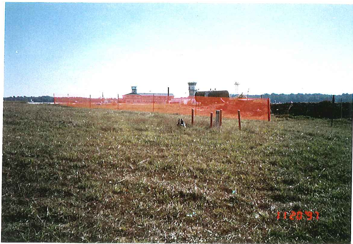
PHOTOGRAPH -20- PERIMETER FENCE INSTALLATION
