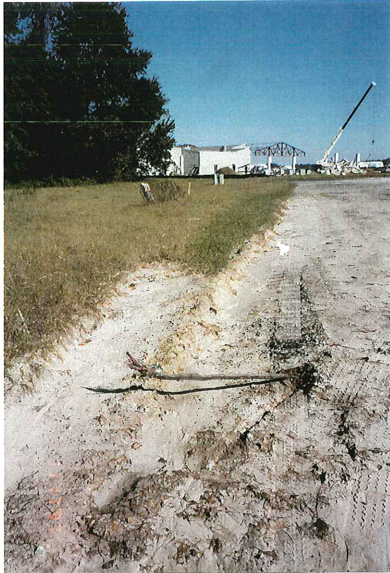
PHOTOGRAPH -10- OUT OF SERVICE UTILITY LINE ALONG DIRT ROAD NORTH OF THE SITE
