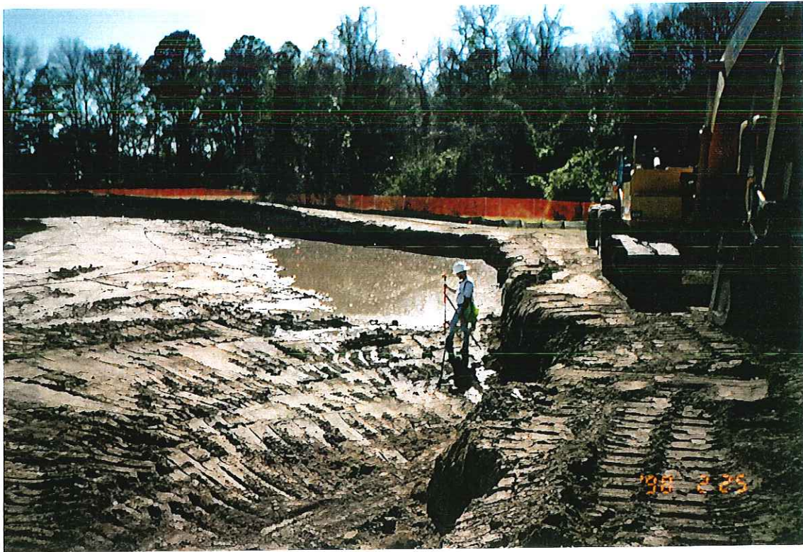
PHOTOGRAPH -83- SURVEY OF GRID AND CONFIRMATORY SAMPLE LOCATIONS
