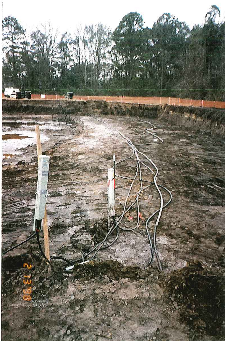
PHOTOGRAPH -73- EXPOSED UTILITIES
