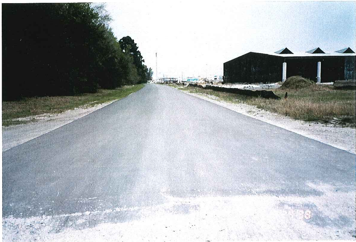
PHOTOGRAPH -100- STRACHAN ROAD (truck haul route)
