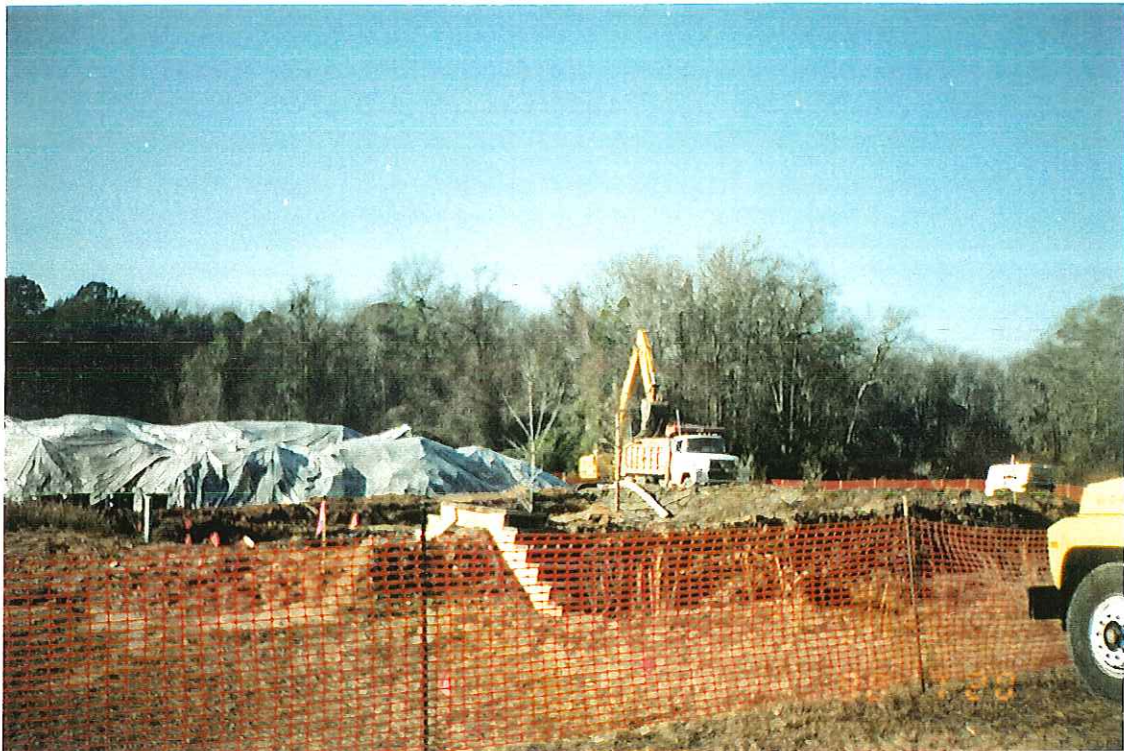
PHOTOGRAPH -65- COVERED STOCKPILED SOILS
