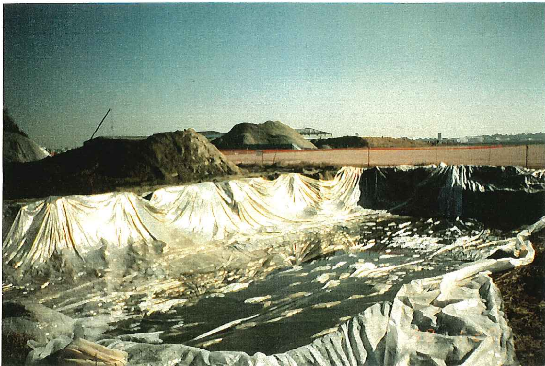
PHOTOGRAPH -66- LINING OF EXCAVATION
