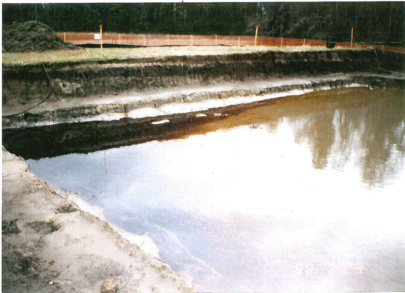
PHOTOGRAPH -80- FREE PRODUCT IN EXCAVATION
