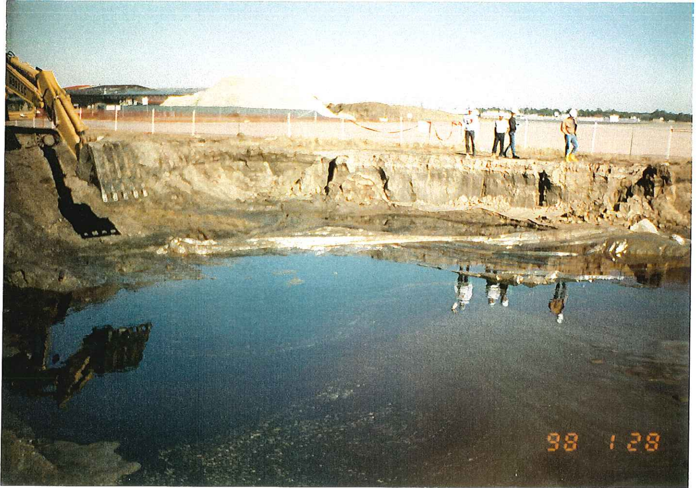
PHOTOGRAPH -69- REMOVAL OF PLASTIC LINING FROM EXCAVATION
