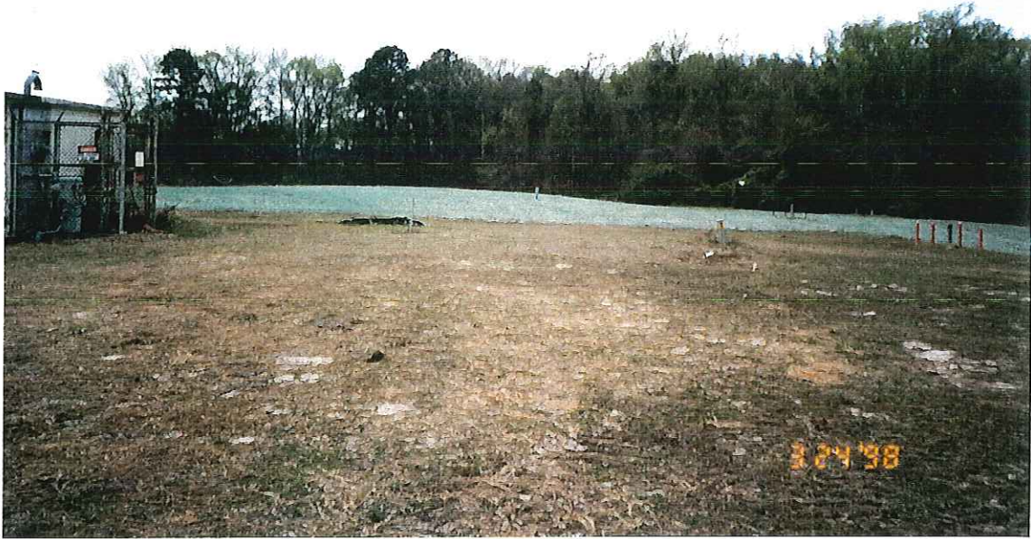
PHOTOGRAPH -97- EXCAVATION SITE AFTER HYDRO-SEEDING
