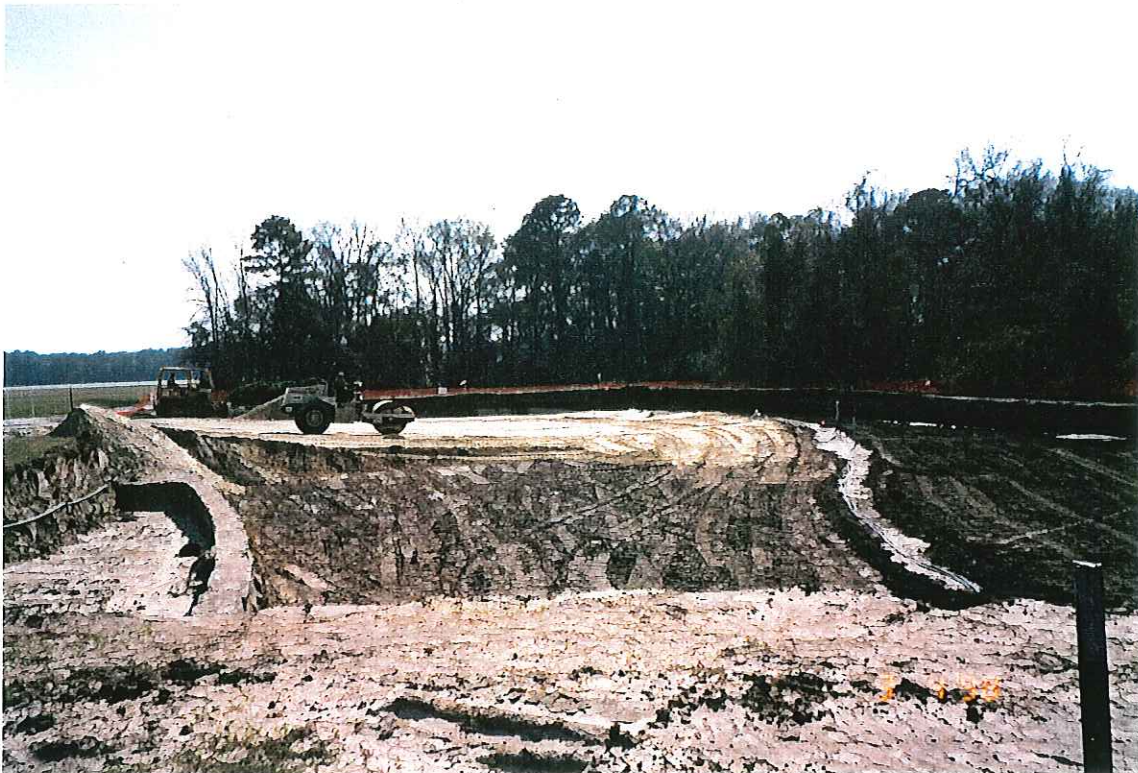
PHOTOGRAPH -88- BACKFILL ACTIVITIES
