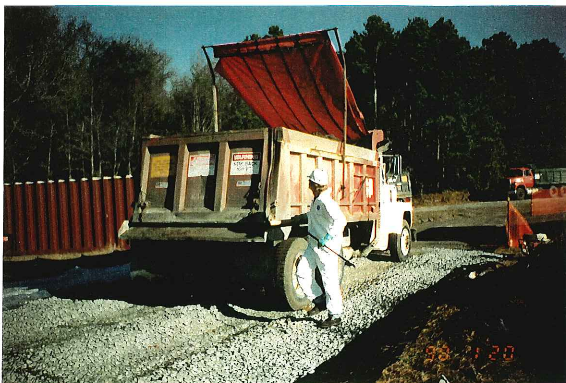
PHOTOGRAPH -60- CLEANING TRUCKS
