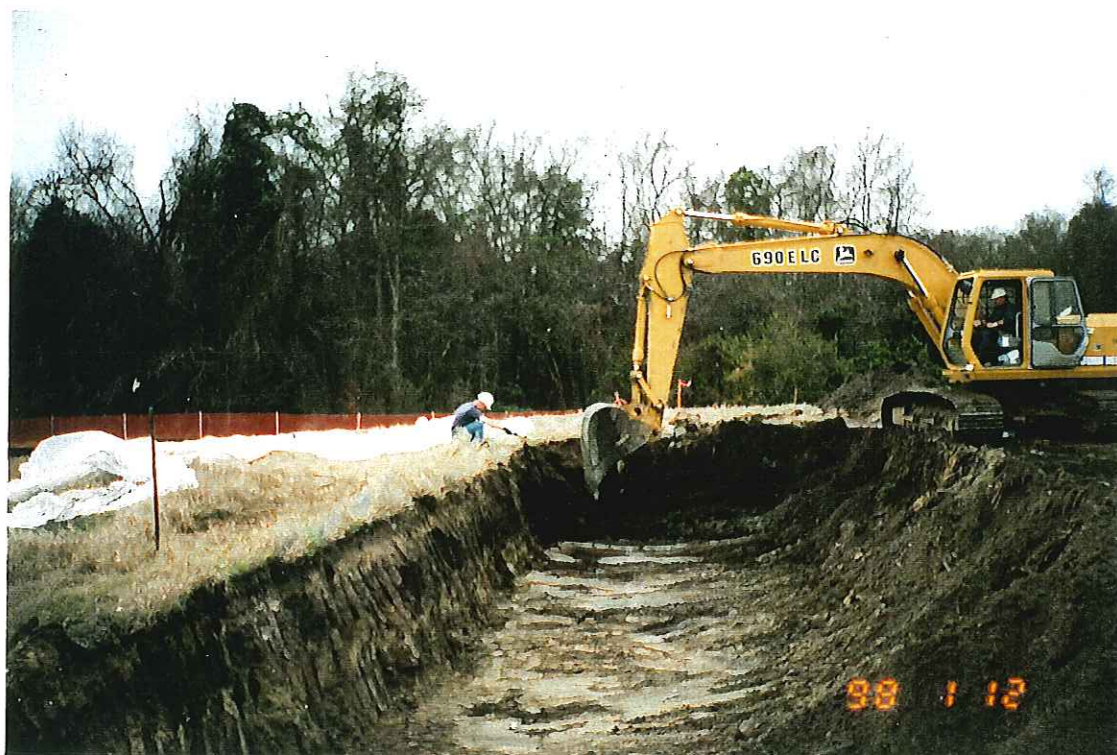
PHOTOGRAPH -54- AMBIENT AIR MONITORING DURING EXCAVATION ACTIVITIES
