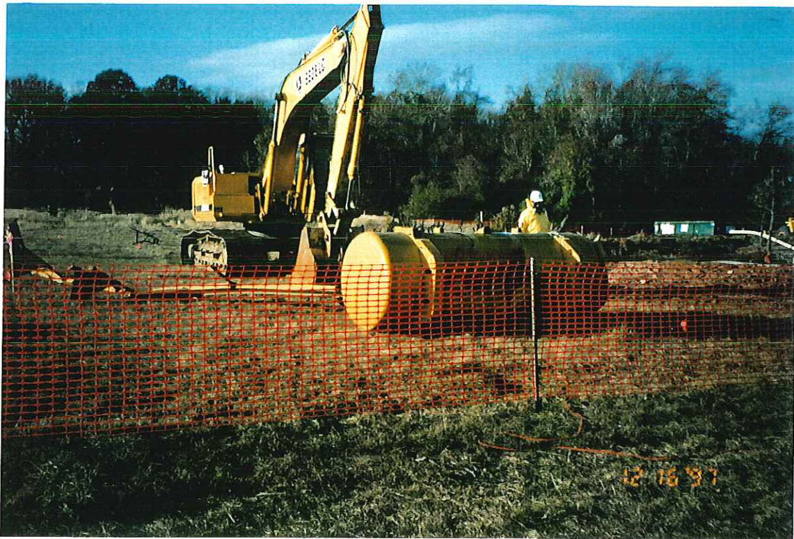
PHOTOGRAPH -43- DESTRUCTION OF 1100 GALLON ALUMINUM TANK
