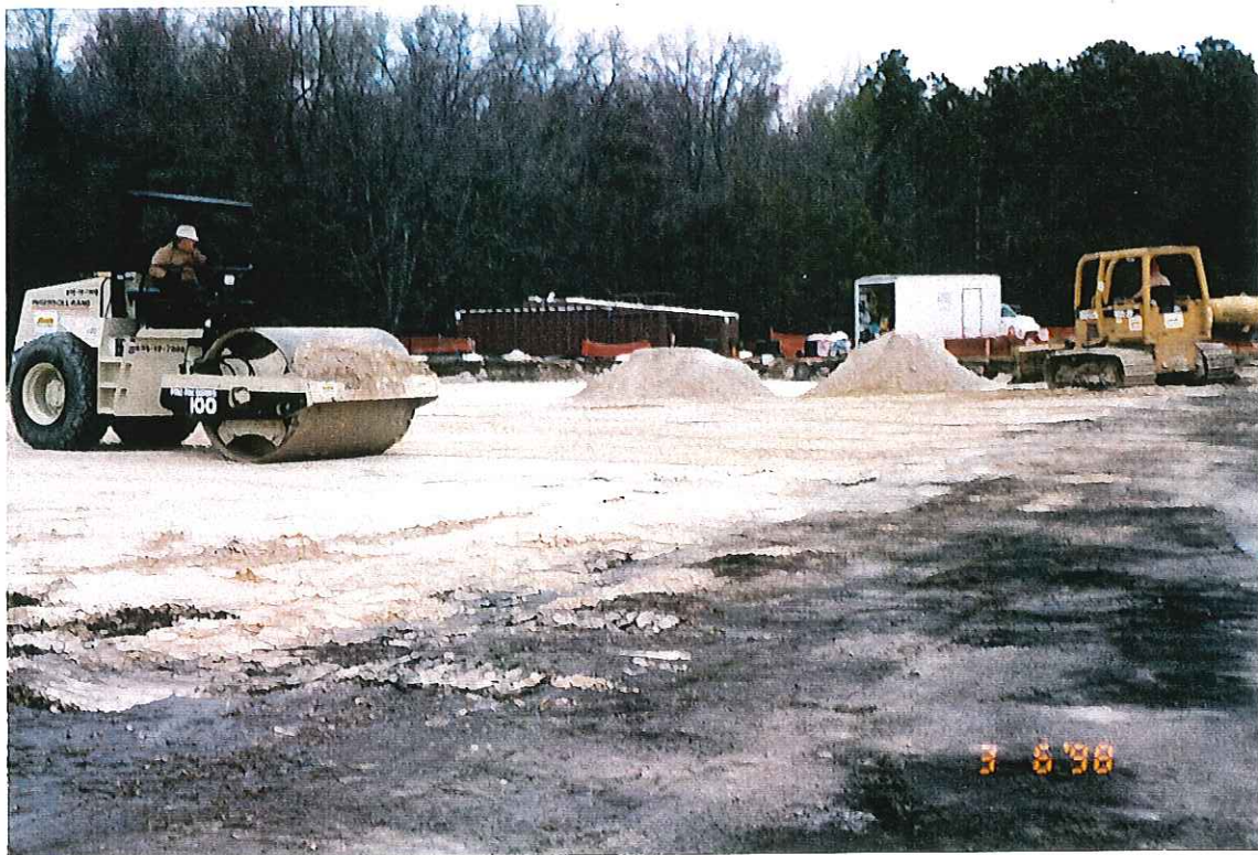
PHOTOGRAPH -92- BACKFILL ACTIVITIES
