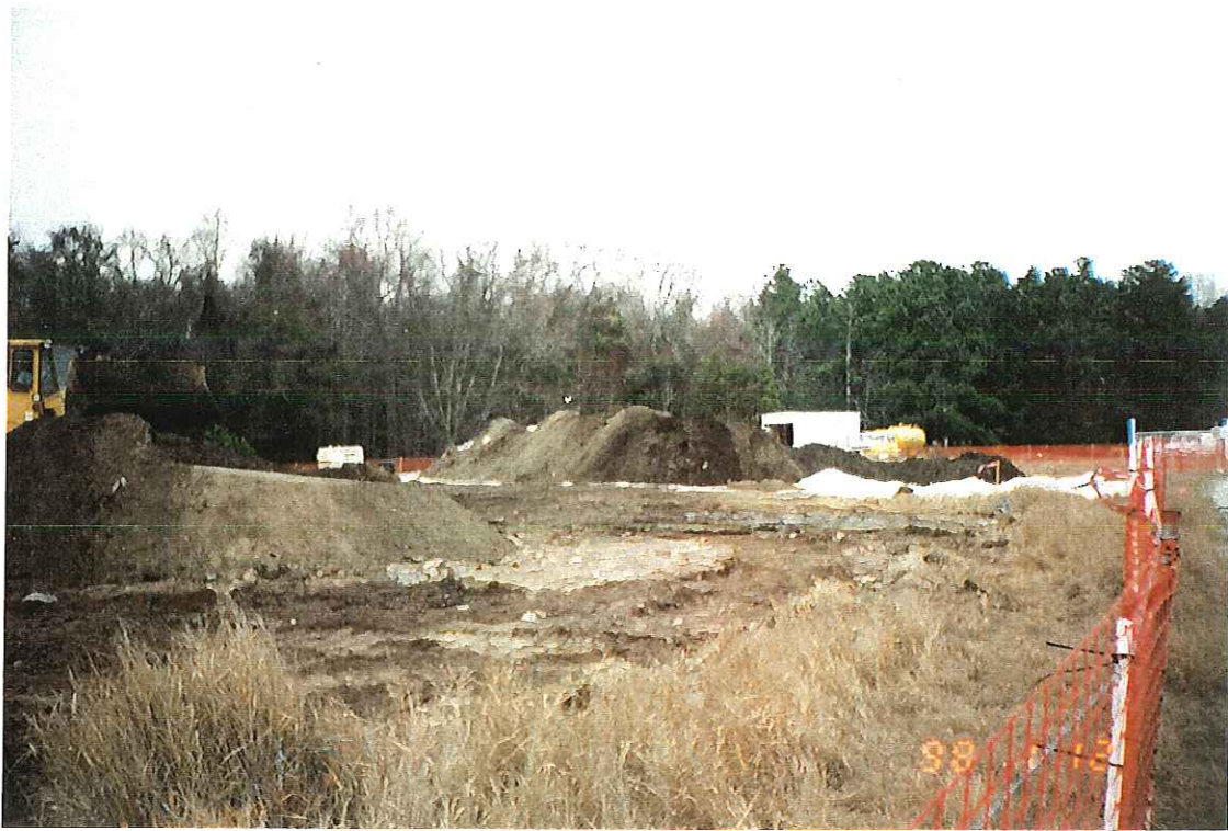
PHOTOGRAPH -57- STOCKPILED EXCAVATED SOILS
