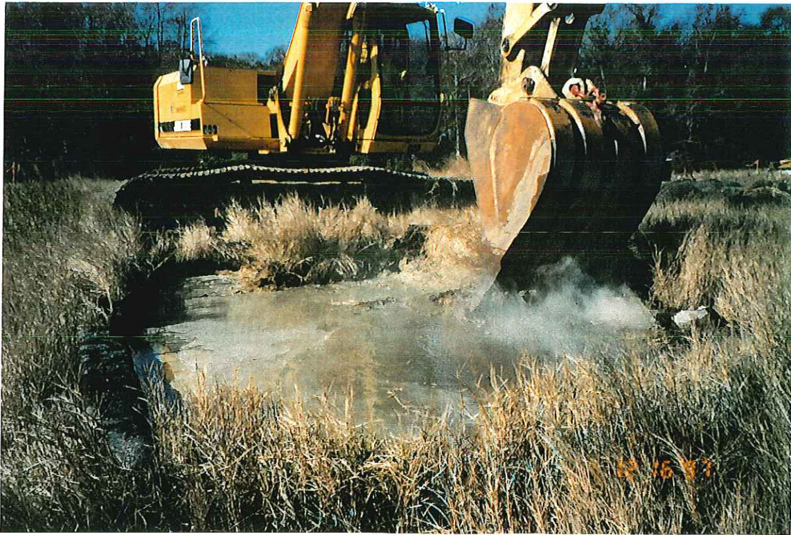
PHOTOGRAPH -47- SOIL REMOVAL FROM CONCRETE PAD
