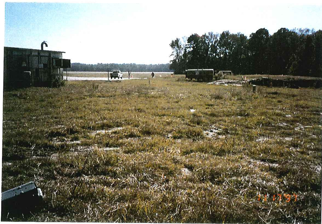
PHOTOGRAPH -6- SITE SURVEY OF EXCAVATION LIMITS
