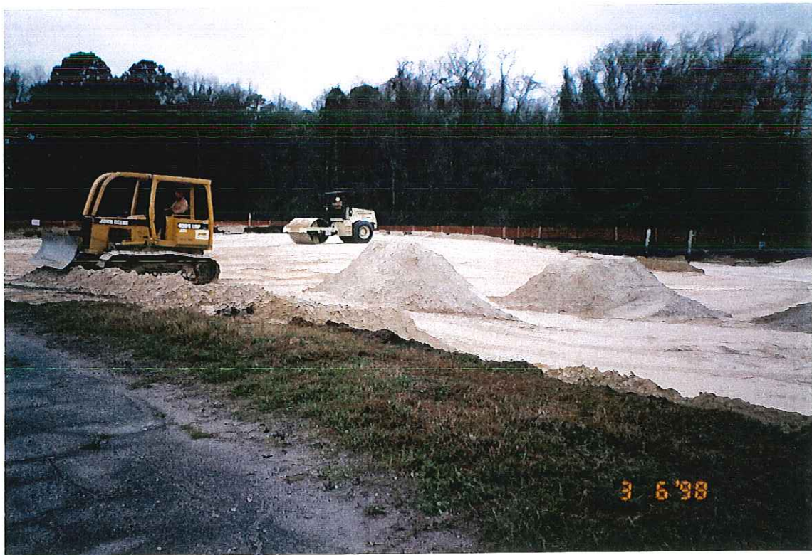
PHOTOGRAPH -91- BACKFILL ACTIVITIES
