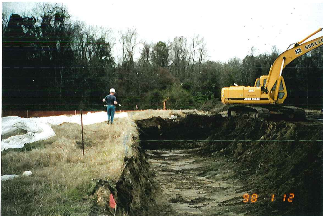
PHOTOGRAPH -53- AMBIENT AIR MONITORING DURING EXCAVATION ACTIVITIES
