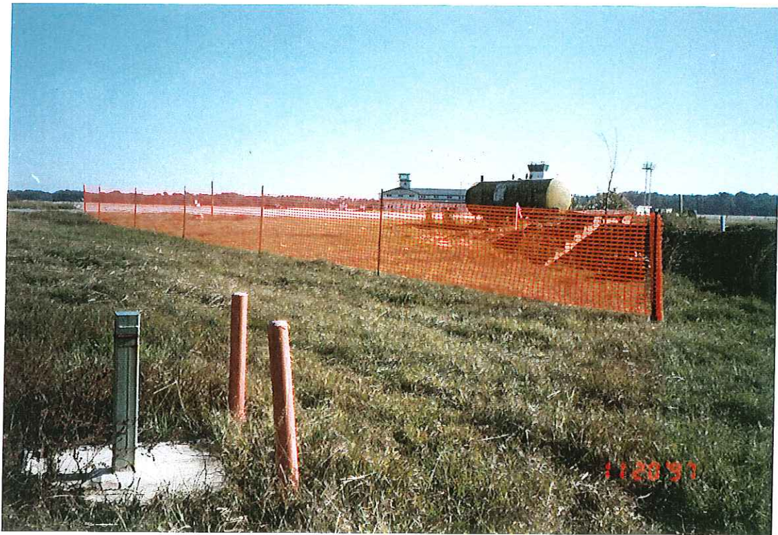
PHOTOGRAPH -21- PERIMETER FENCE INSTALLATION
