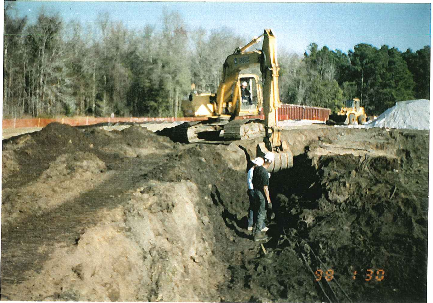
PHOTOGRAPH -70- EXCAVATION ACTIVITIES (EXPOSING UTILITIES)
