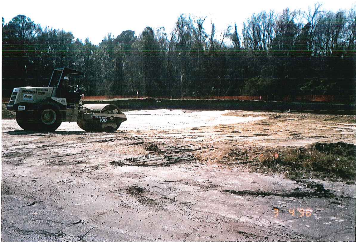
PHOTOGRAPH -89- BACKFILL ACTIVITIES
