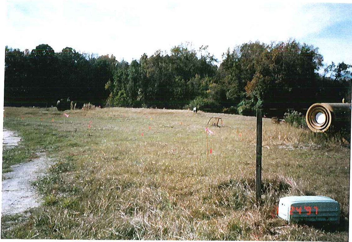
PHOTOGRAPH -28- MARKING OF ON-SITE UTILITIES
