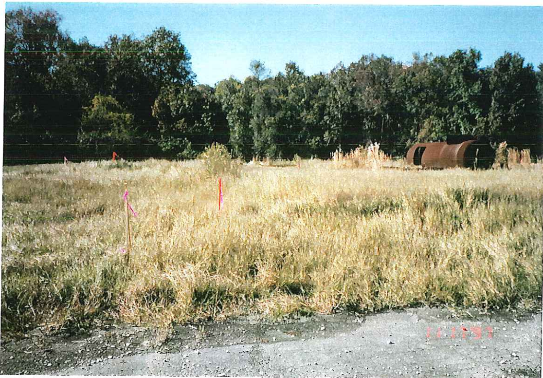
PHOTOGRAPH -7- SURVEY STAKES MARKING EXCAVATION LIMITS
