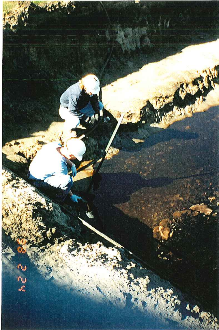
PHOTOGRAPH -82- REMOVAL OF FREE PRODUCT FROM EXCAVATION
