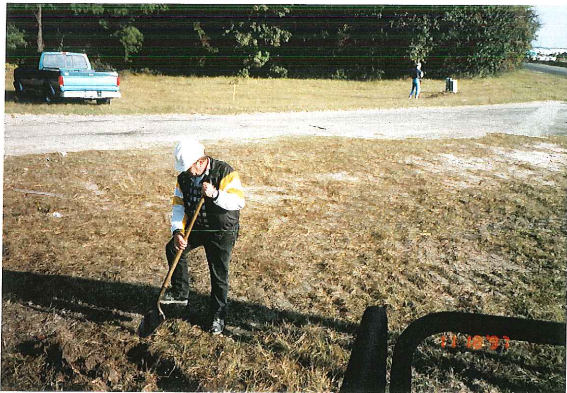
PHOTOGRAPH -17- HAND DIGGING LOCATING UTILITY LINES
