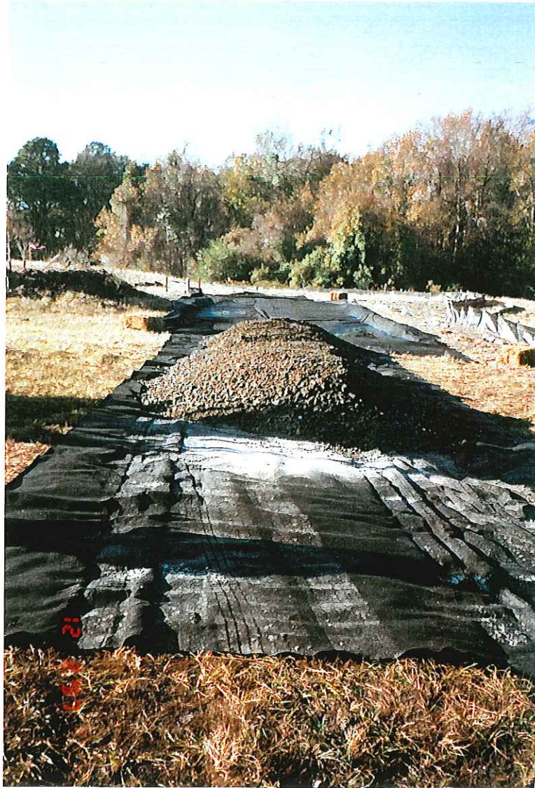
PHOTOGRAPH -32- DECON PAD CONSTRUCTION ACTIVITIES
