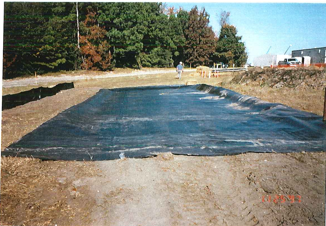
PHOTOGRAPH -30- DECON PAD CONSTRUCTION ACTIVITIES
