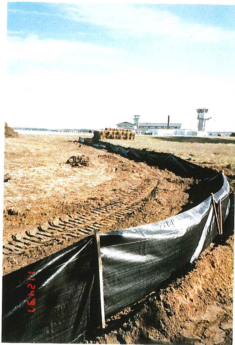
PHOTOGRAPH -22- SILT FENCE INSTALLATION
