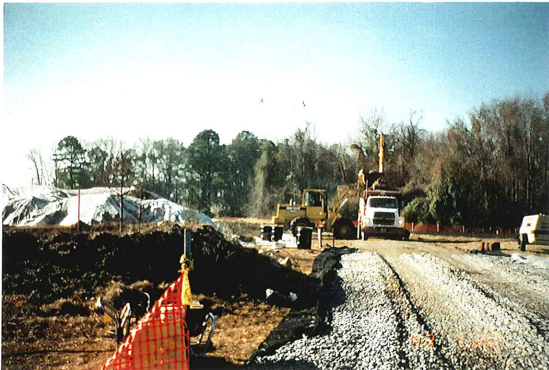
PHOTOGRAPH -58- LOADING OF EXCAVATED SOILS
