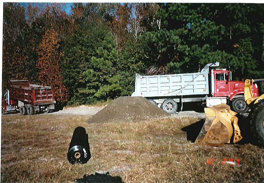
PHOTOGRAPH -31- DECON PAD CONSTRUCTION ACTIVITIES
