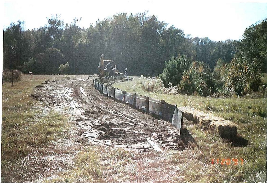
PHOTOGRAPH -18- SILT FENCE INSTALLATION
