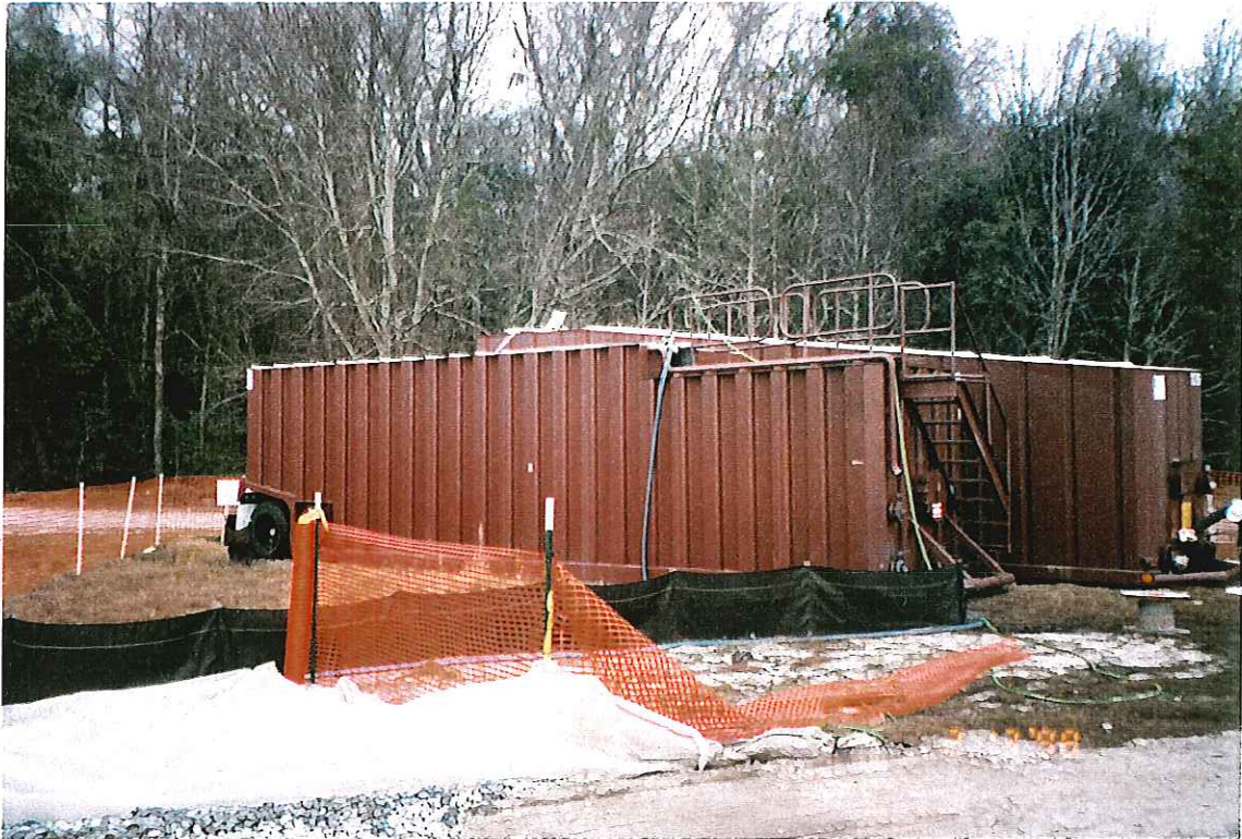
PHOTOGRAPH -74- MOBILE WATER STORAGE TANKS (Storing wastewater generated from excavation activities)
