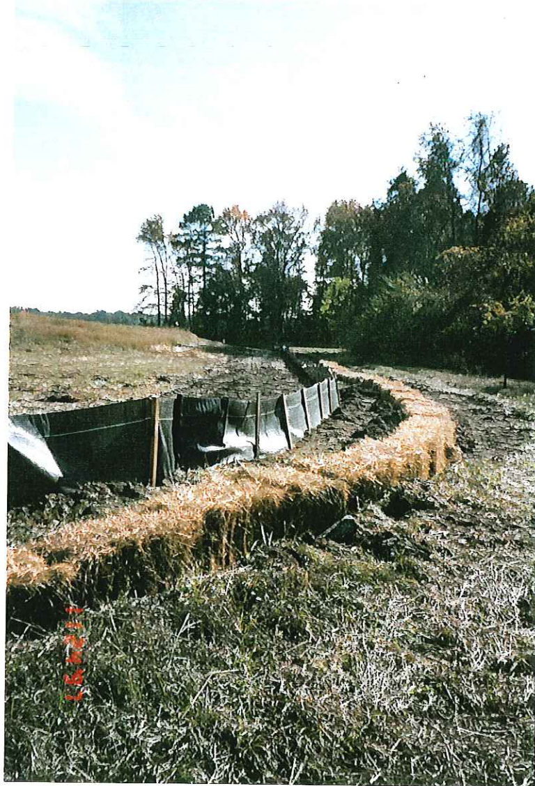
PHOTOGRAPH -25- INSTALLATION OF HAY BALES
