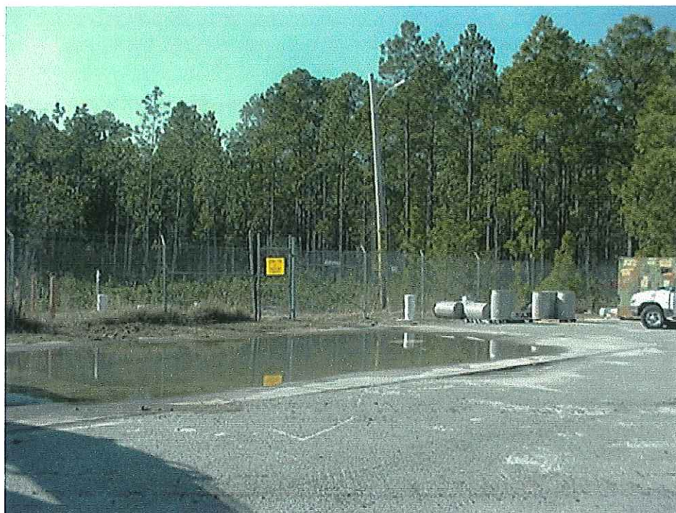
Former 724th TPS: Former 724th TPS prior to Interim Removal Action.
