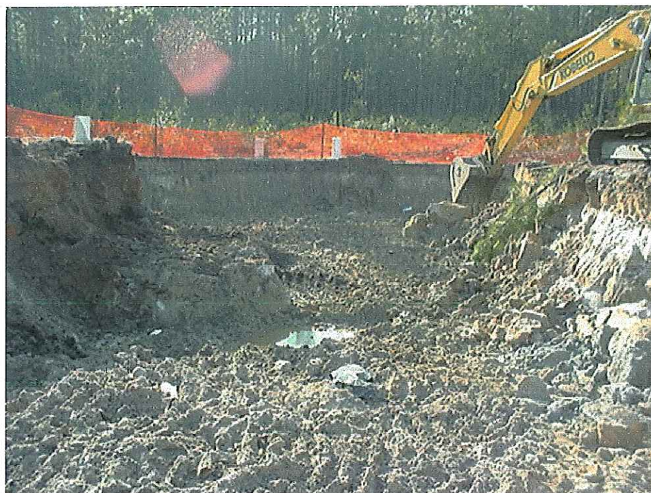
Former 724th TPS: Removal of contaminated soil at the Former 724th TPS.
