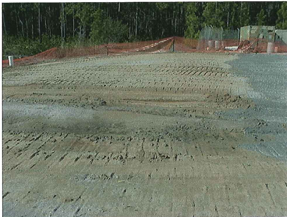
Former 724th TPS: Former 724th TPS area after backfilling.
