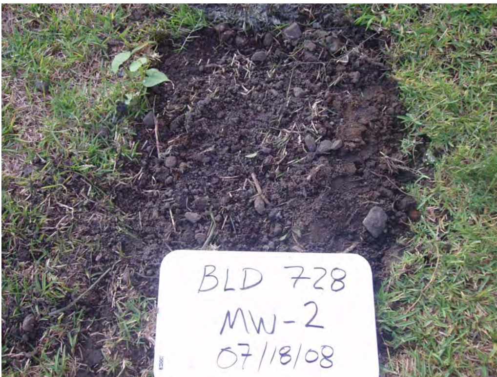
Former Building 728: Well Abandonment – 728-MW-02
