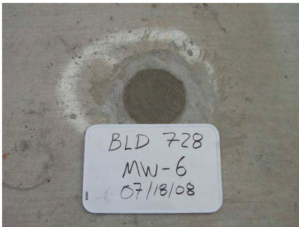
Former Building 728: Well Abandonment – 728-MW-06
