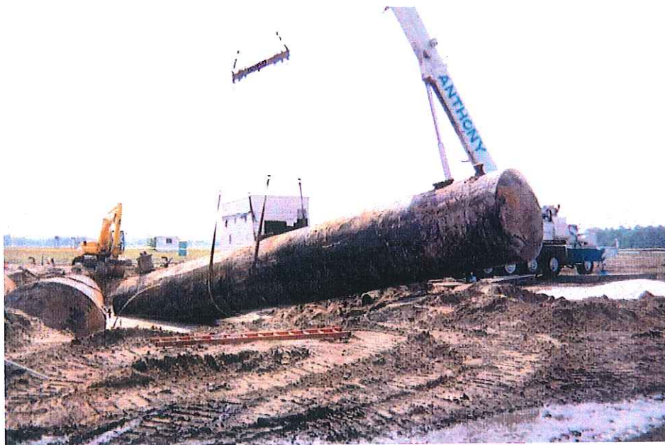
Pumphouse #6: Tank #83 being removed.
