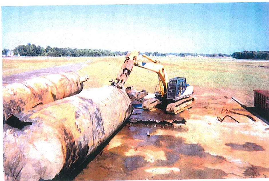
Pumphouse #6: Tank #82 being cut. Tank #83 is to the left.
