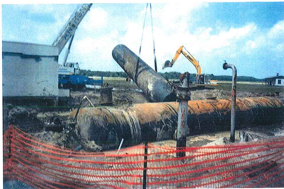
Pumphouse #6: Tank #82 being removed from excavation. Tank #89 in foreground.
