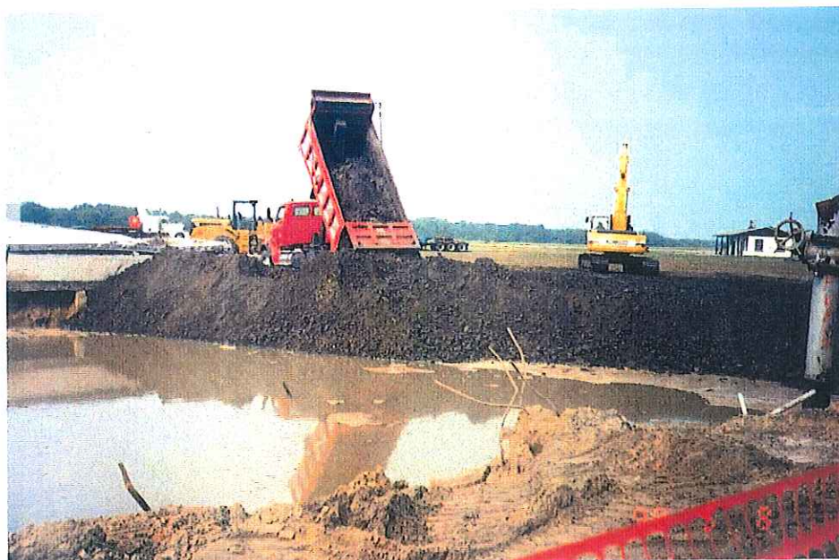
Pumphouse #6: View southwest of ongoing backfill activities.
