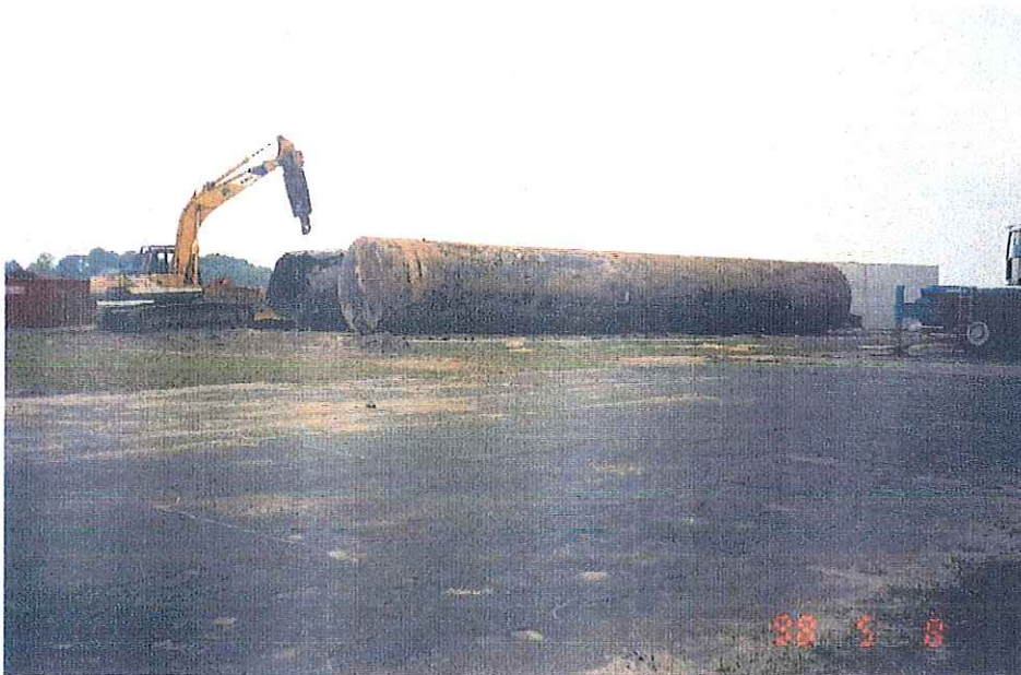
Pumphouse #6: Tank #90 staged at decontamination pad. Tank #91 is being sheared in background.
