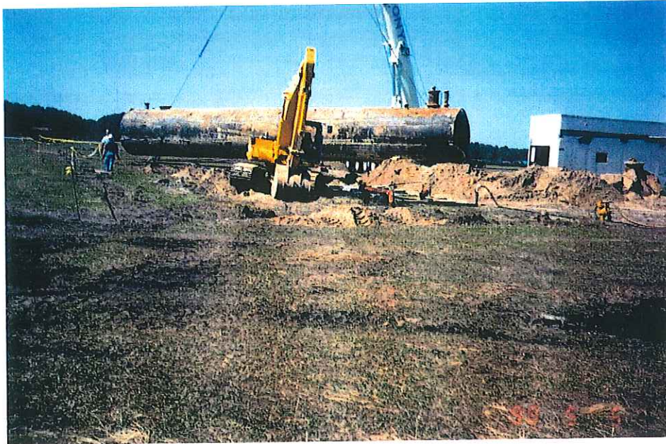
Pumphouse #6: Tank #87 after removal.
