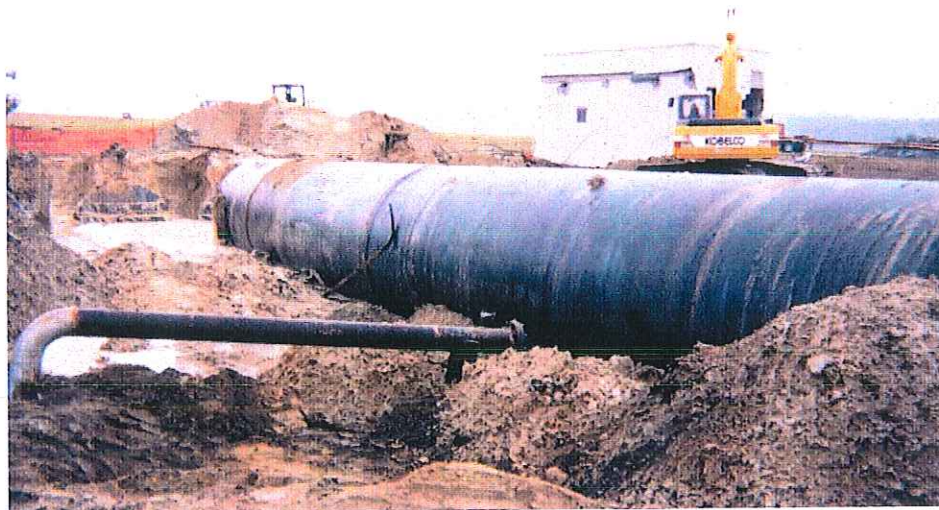
Pumphouse #6: Tank #86 excavation area.
