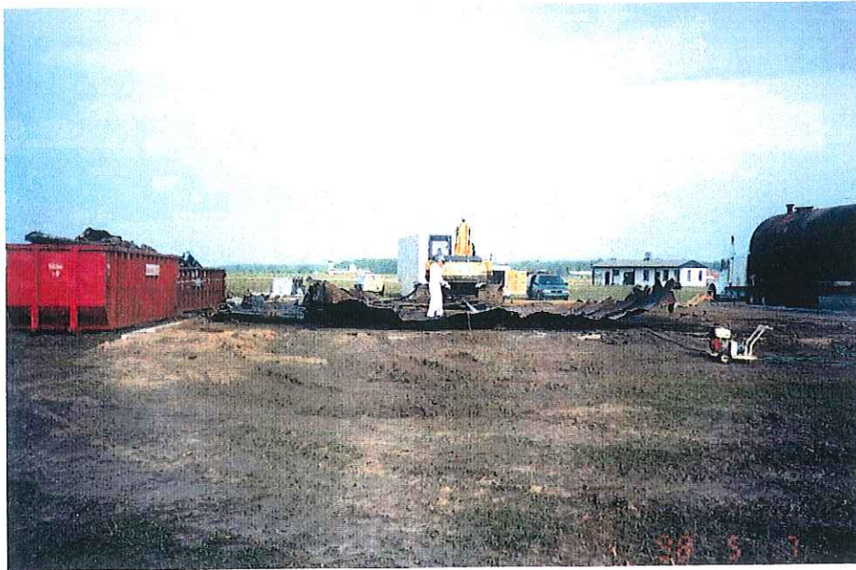
Pumphouse #6: Tank #88 being decontaminated.
