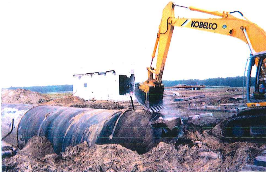
Pumphouse #6: Tank #84 being excavated.
