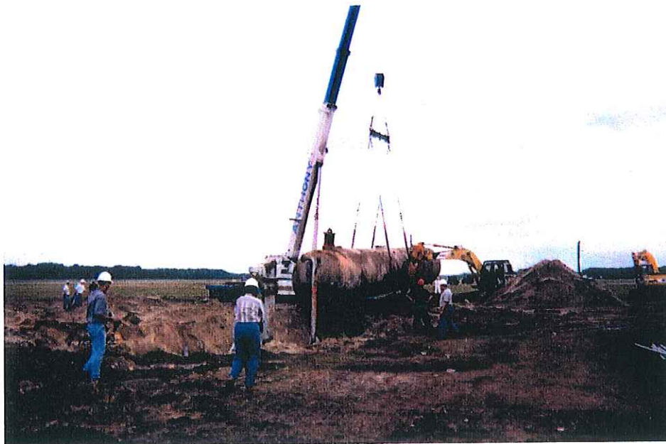
Pumphouse #6: Tank #86 removal.
