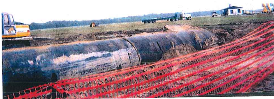
Pumphouse #6: Tank #85 in place.
