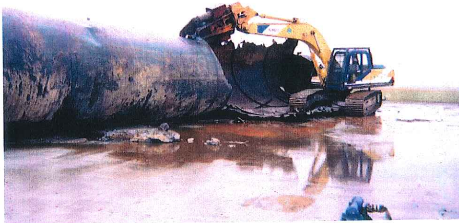
Pumphouse #6: Tank #86 being cut. Note no sludge in tank.
