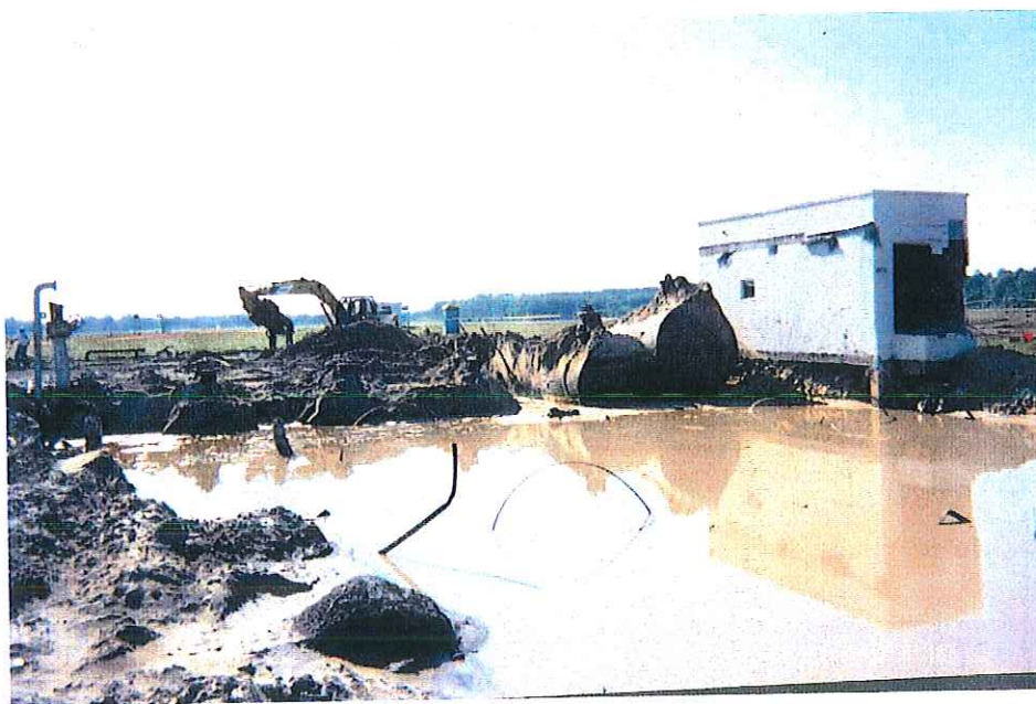
Pumphouse #6: Tanks #87 (nearest building) and #88 ready for removal.
