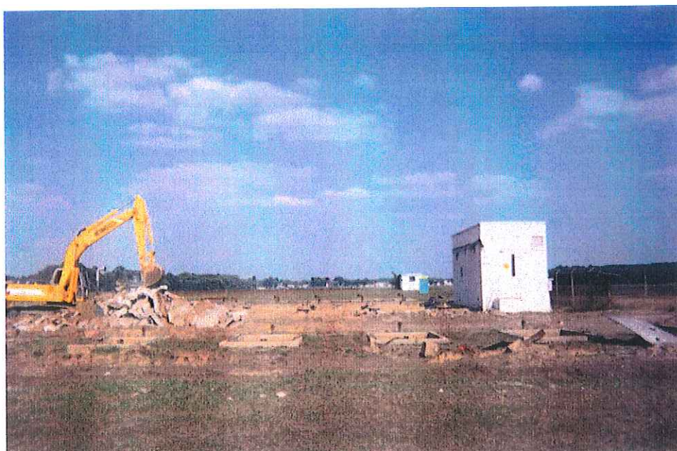
Pumphouse #6: Pumphouse #6 prior to removal of USTs.
