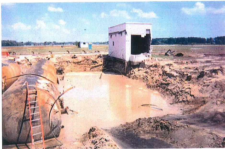
Pumphouse #6: Excavation area after removal of tanks #83 and #82.
