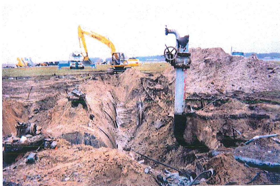
Pumphouse #6: Tank #86 excavation, view to west. Note fuel lines along right side of tank.
