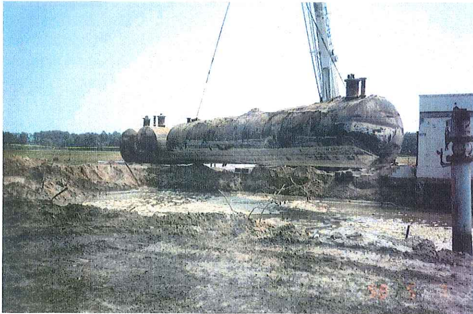
Pumphouse #6: Tank #91 being removed from excavation area.
