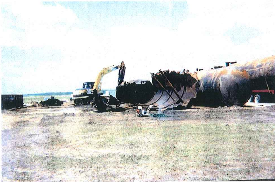
Pumphouse #6: Tank #84 being sheared.
