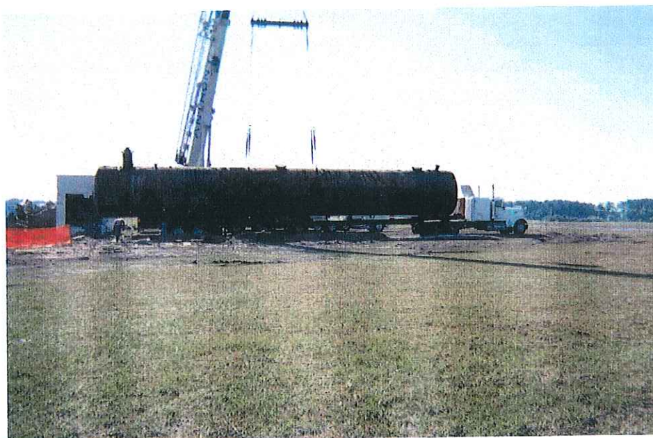
Pumphouse #6: Tank #85 being loaded onto trailer prior to restaging at decontamination pad.
