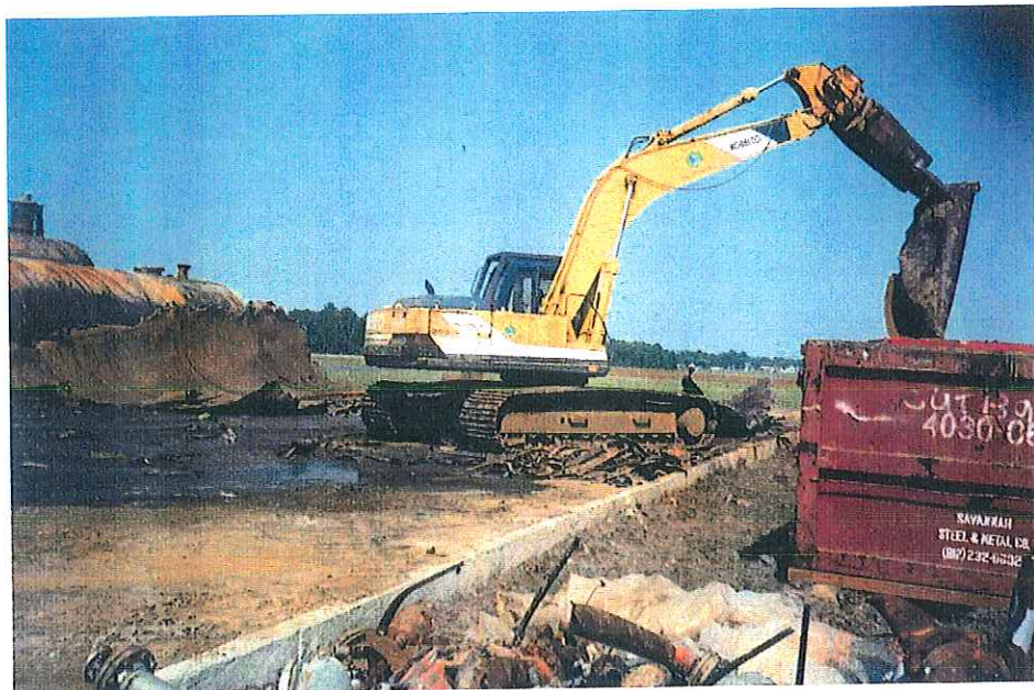
Pumphouse #6: Tank #87 being cut up for scrap and loaded.
