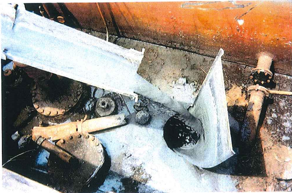
Pumphouse #6: 50,000-gallon defuel tank (#92) being filled with concrete.
