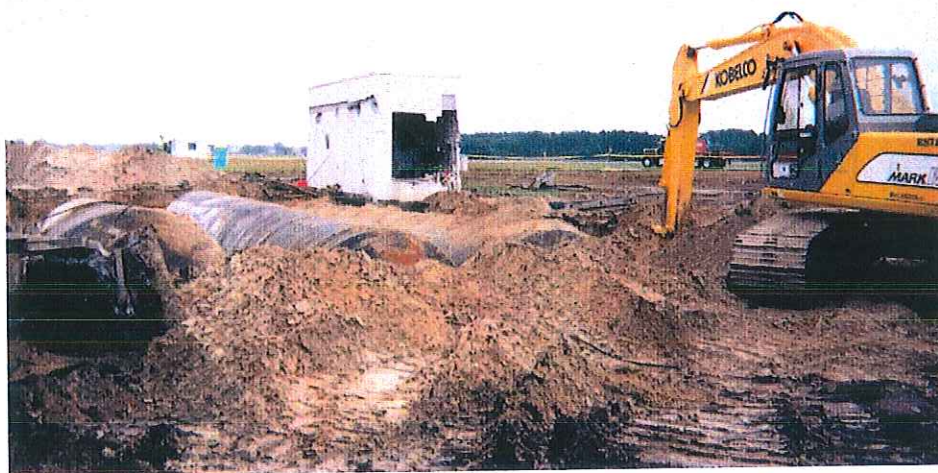
Pumphouse #6: Tanks #84, #83, and #82 being excavated.
