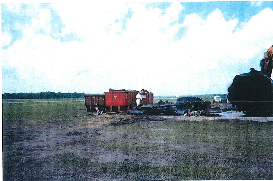
Pumphouse #6: Tanks #88 and #87 being cut for scrap.
