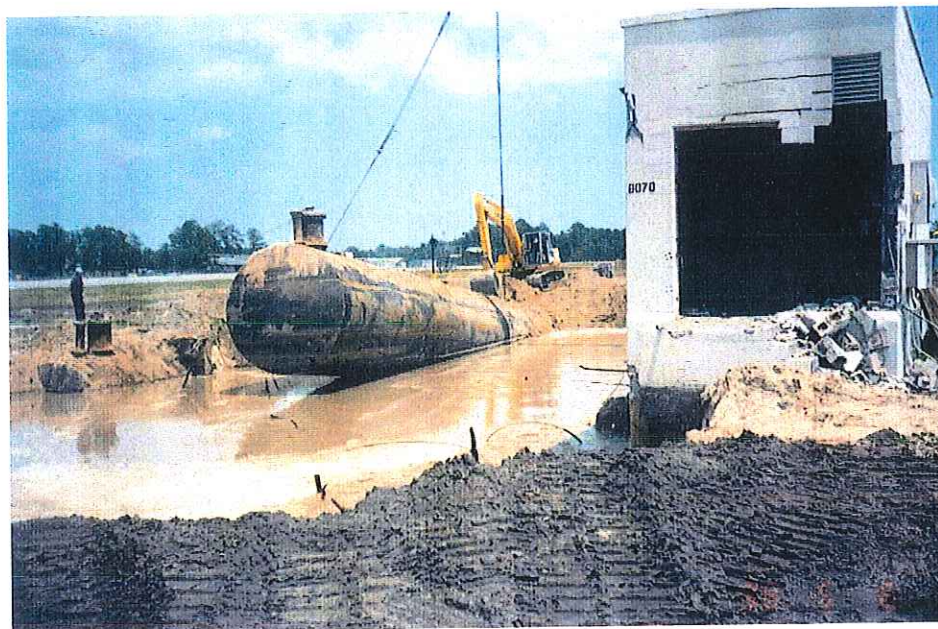
Pumphouse #6: Tank #90 being removed from excavation.
