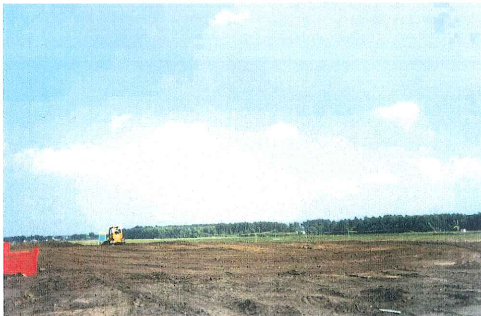
Pumphouse #6: Final grading of tank removal area. View to southeast.
