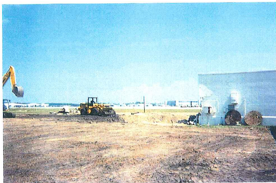
Pumphouse #6: View northwest of backfilling activities.
