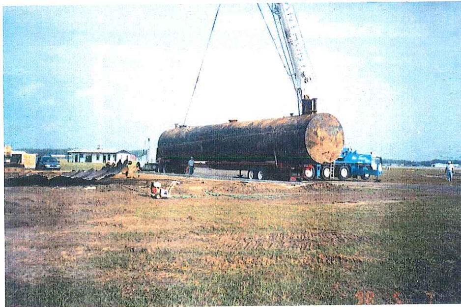
Pumphouse #6: Tank #89 being unloaded at decontamination pad. Tank #88 to the left is being cut for disposal.
