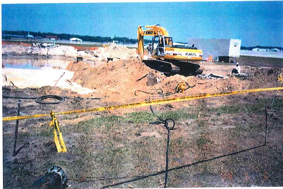
Pumphouse #6: Tanks #87 and #88 excavation area. From left to right, tanks still in ground, #89, #90, and #91.
