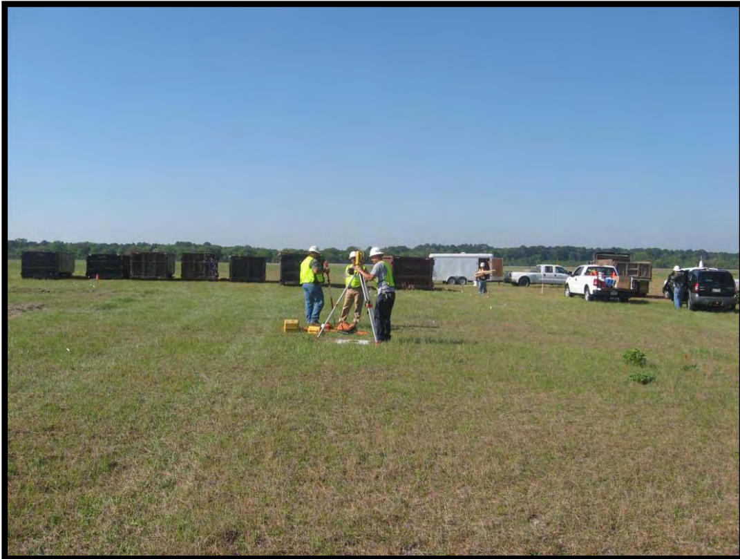
Site preparation – staking excavation area
