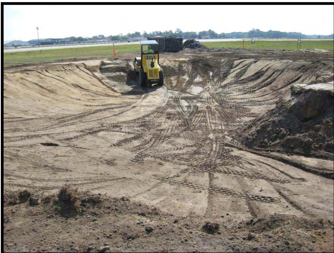
Continued backfilling and compacting
