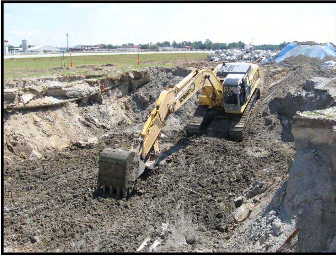
Backfilling excavation
