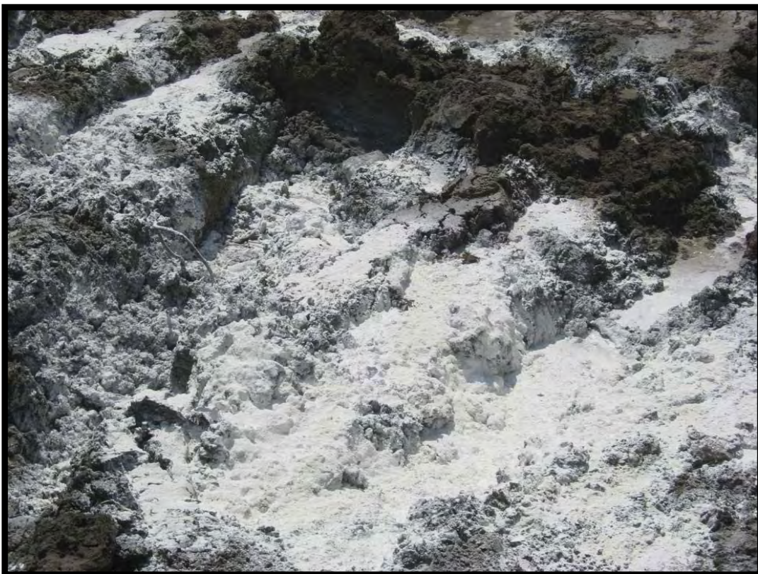
ORC® application to the excavation
