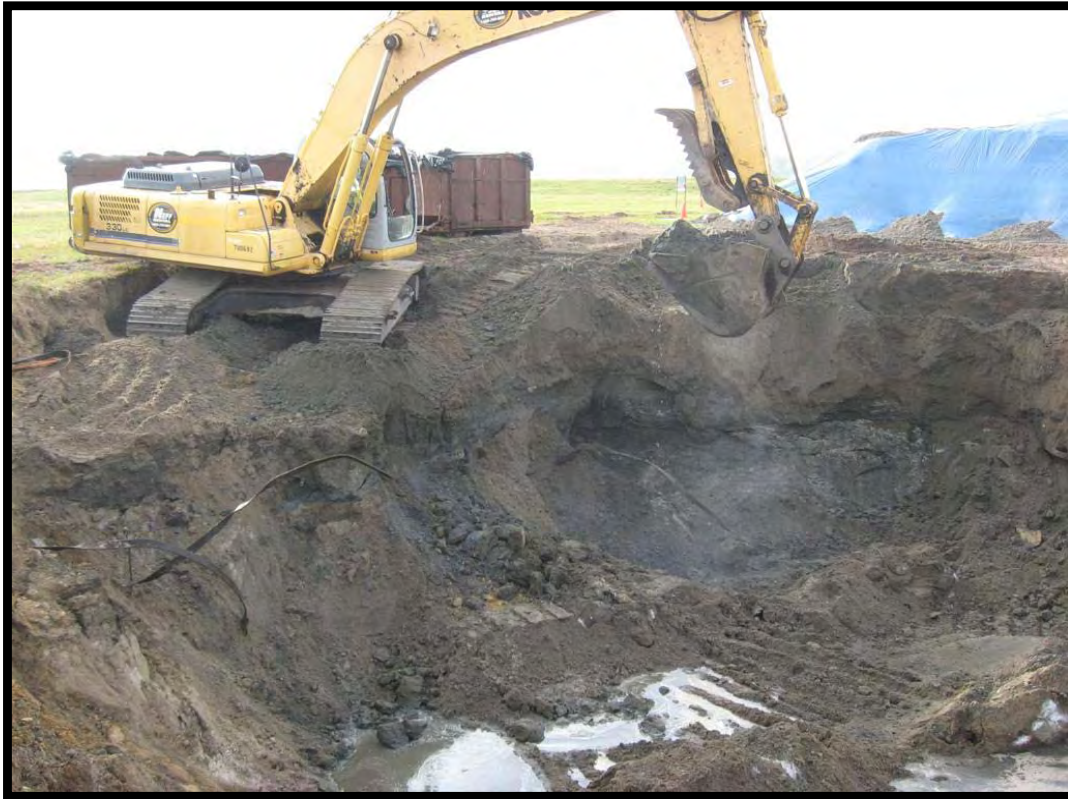
Excavation – groundwater encountered
