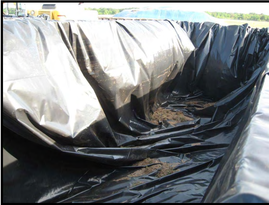
Plastic-lined roll-off for contaminated soils
