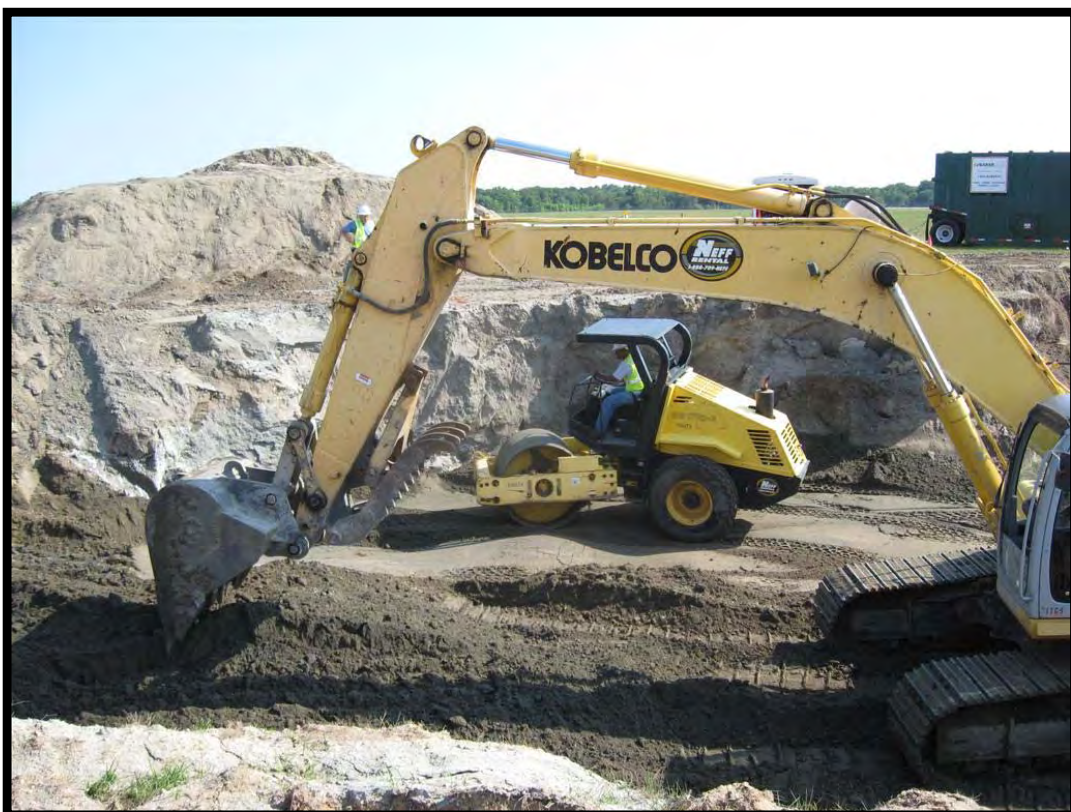
Placing and compacting of backfill
