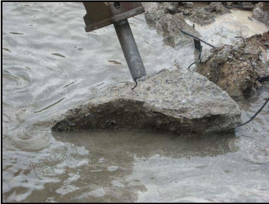
Breaking concrete into manageable pieces
