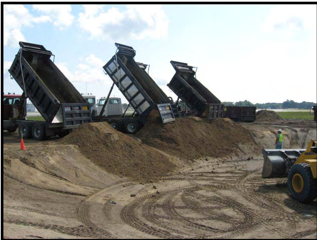
Placing backfill from borrow source
