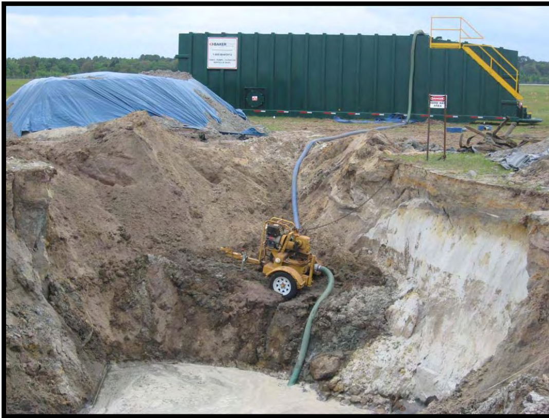
Dewatering the excavation into a Baker Tank
