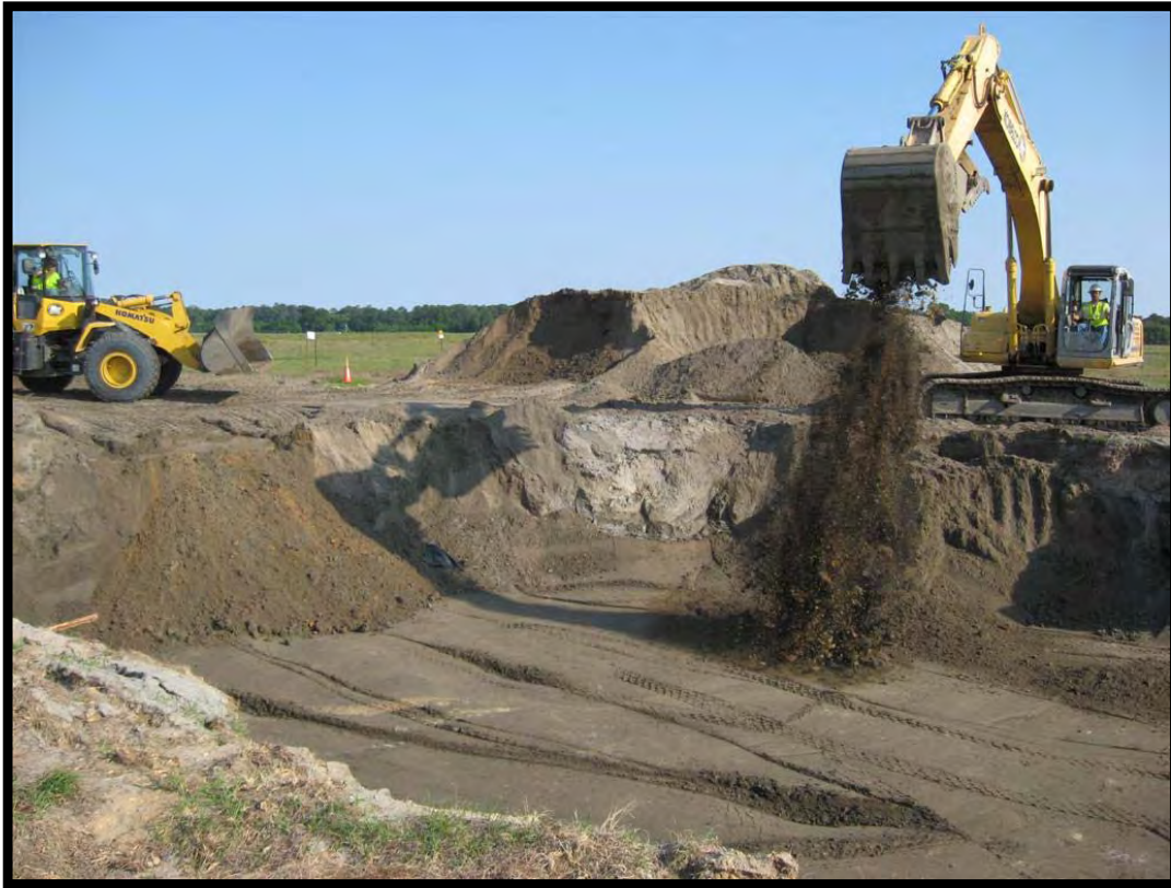
Placing clean soil backfill
