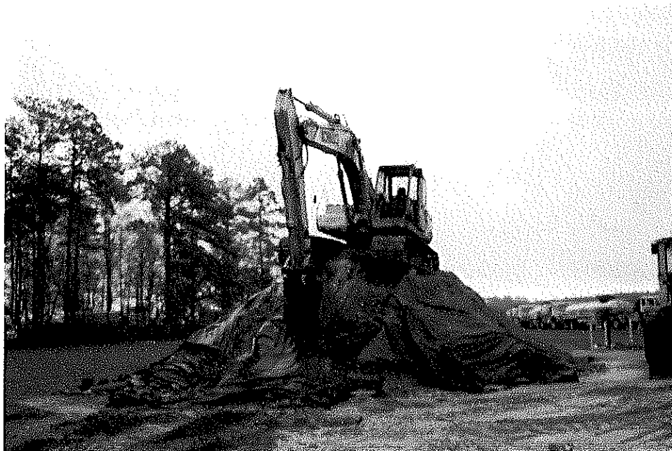
WAAF SWMU 13: Stockpiled soil after removal.
