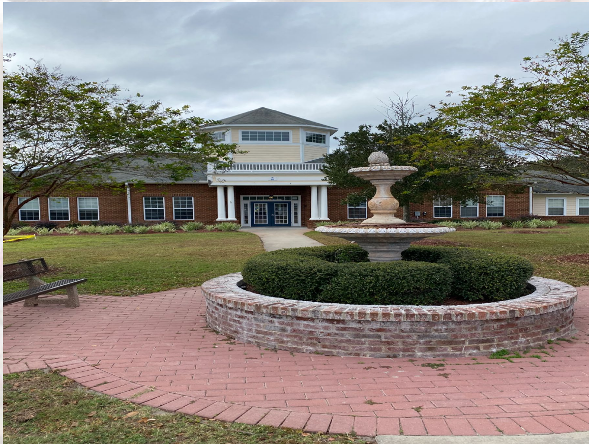
Liberty Woods Community Center, 50 Austin Road
