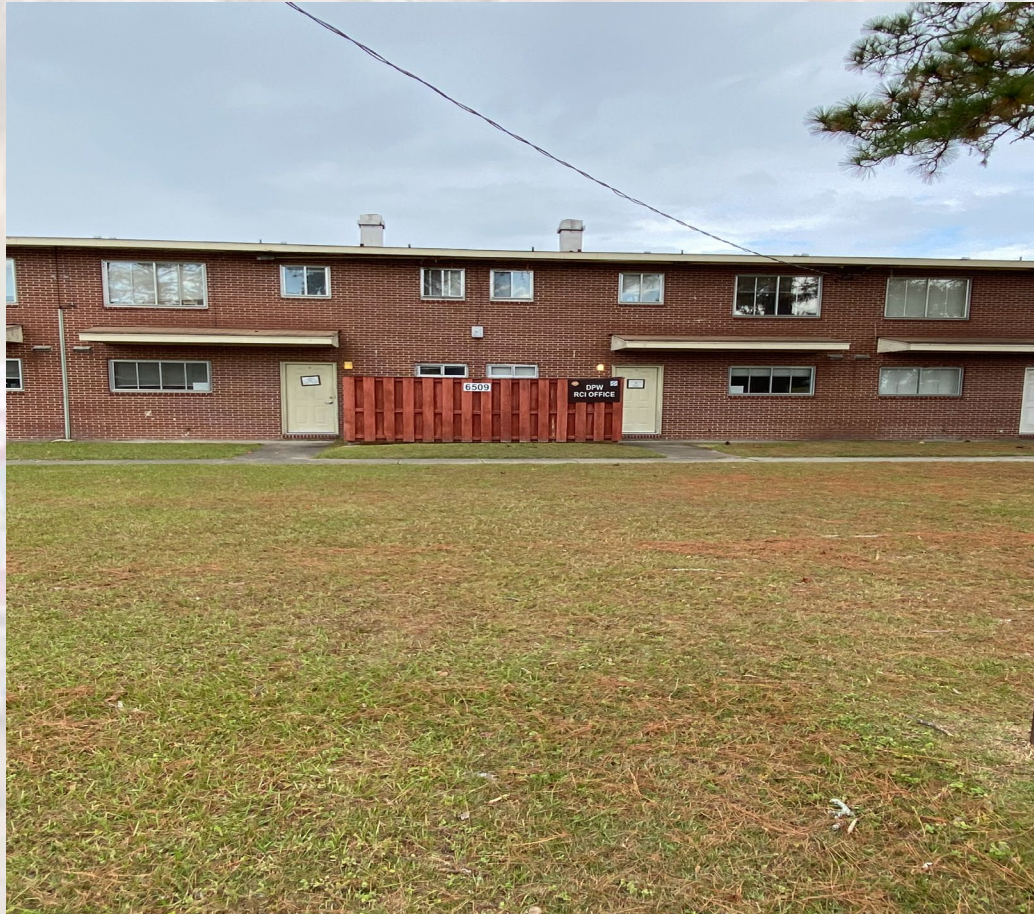
US Army Garrison Housing Office, Bldg. 6509 on Bundy Ave. (Suites 4 and 5)
