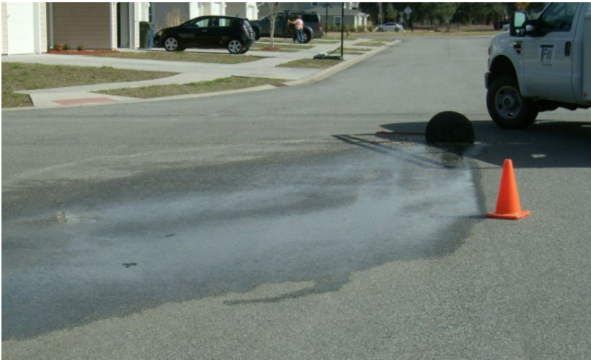
Caption: Sewage spills caused by grease-clogged pipes.
