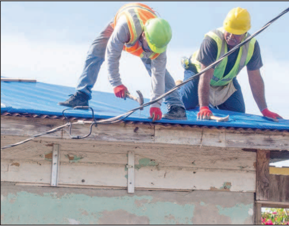
A contractor crew installs a temporary blue roof in Mayagüez, Puerto Rico, Dec. 30.
